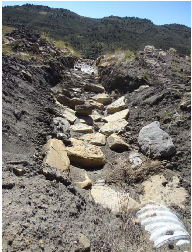
Photo 2: Armored ditch below C4
