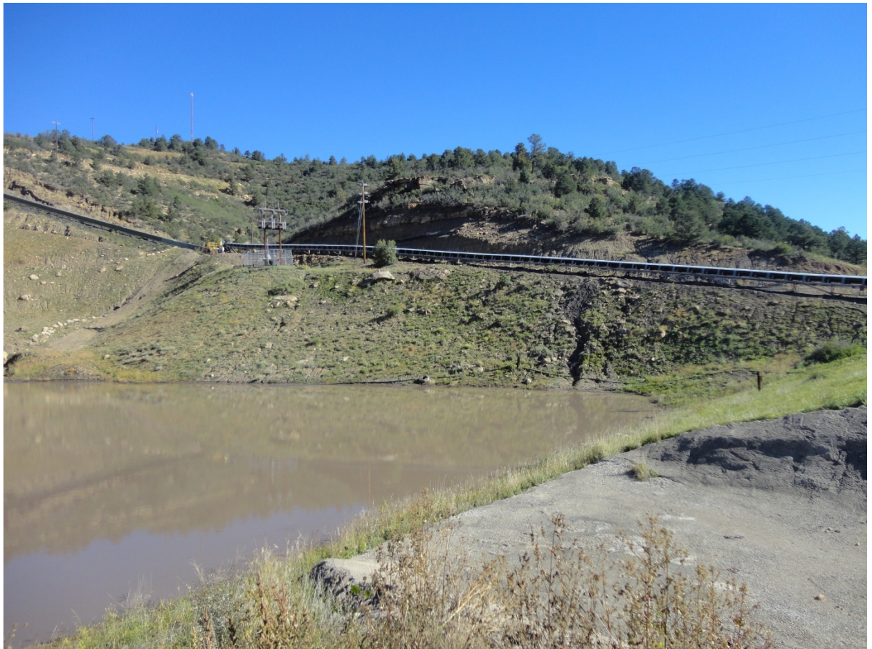
Photo 10: Erosion around pond 8, scheduled for repair
