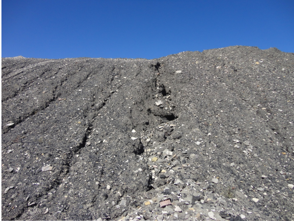
Photo 20: Surface erosion of DWDA2
