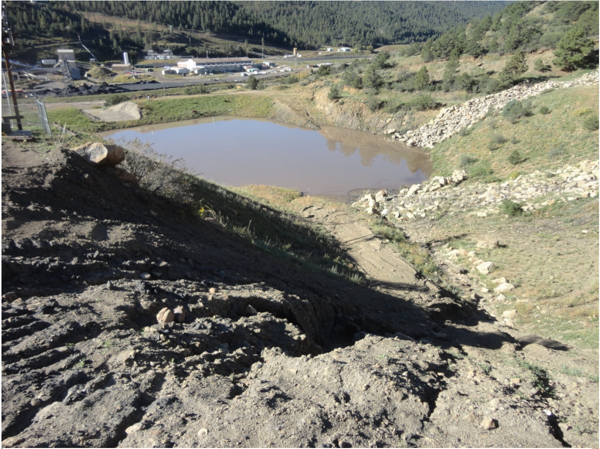
Photo 11: Pond 8 from above, showing where temporary gully repair had partially washed out
