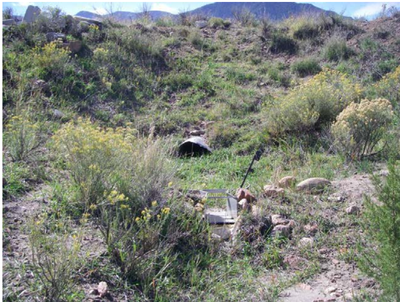
Pond 5 primary spillway below dam
