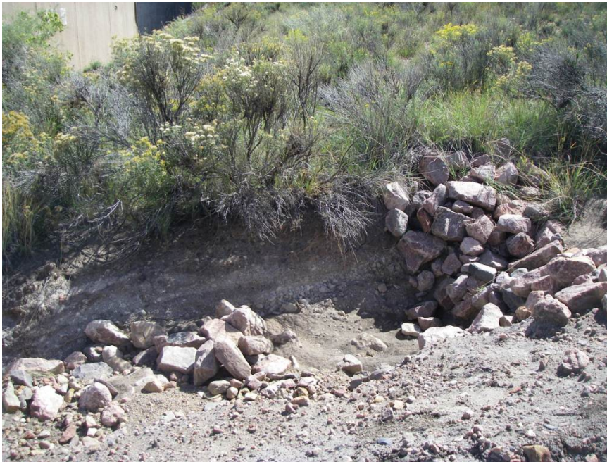
Check dam near truck tunnel
