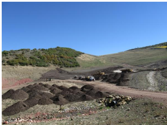
Reclamation at the former Pond 016A site. Topsoil application.
