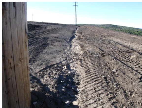
Drainage ditch on the top bench of Horse Gulch fill.
