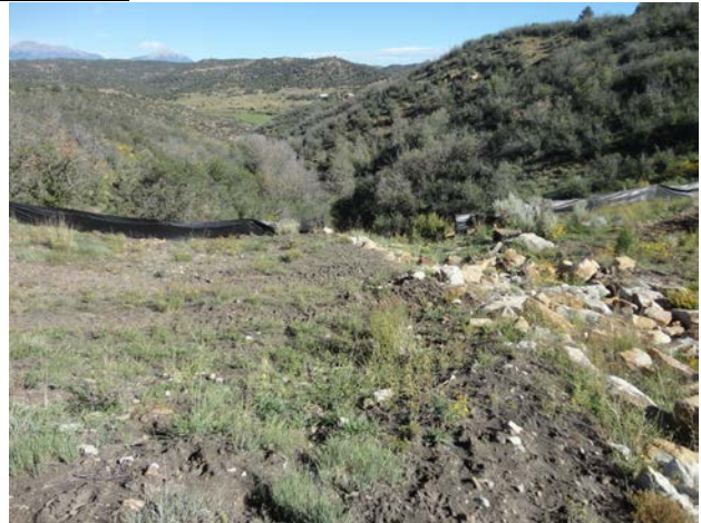
Photo 2: Restored silt fence below pond 9 embankment
