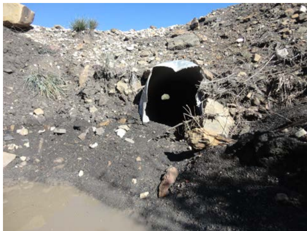
Photo 7: C1 to be flushed and repaired
