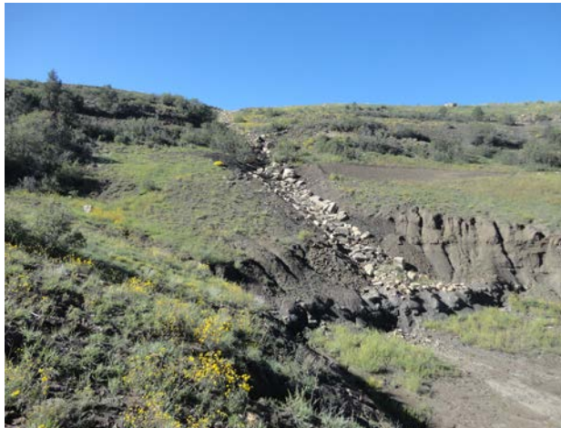
Photo 3: Pond 9, showing repaired gully (1)
