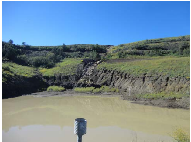
Photo 4: Pond 9, showing repaired gully (2)
