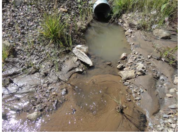
Photo 54: Upwelling from buried culvert bypassing C16c
