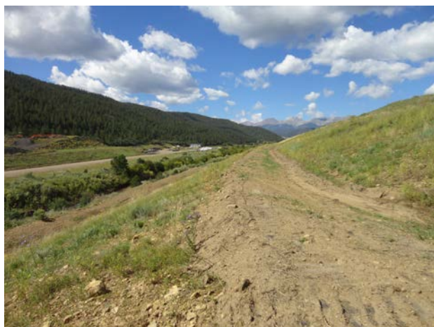
Photo 9: Repaired contour ditch on DWDA 1
