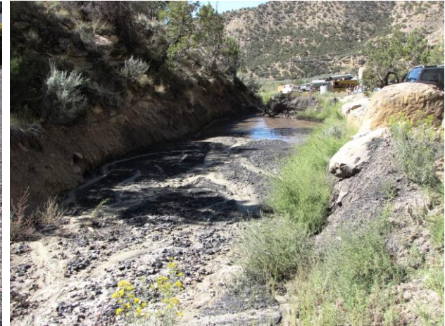
Sediment Trap on South Side of Haul Road
