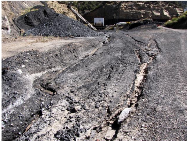
Rill Formation on Upper Portion of Haul Road
