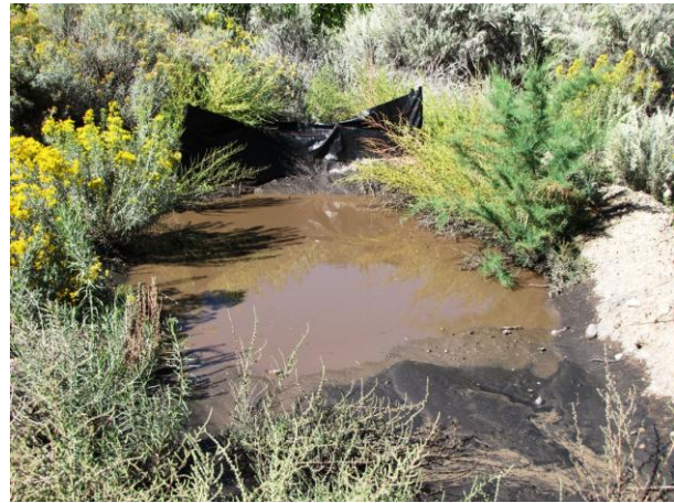
Silt Fence at Road Bridge Crossing
