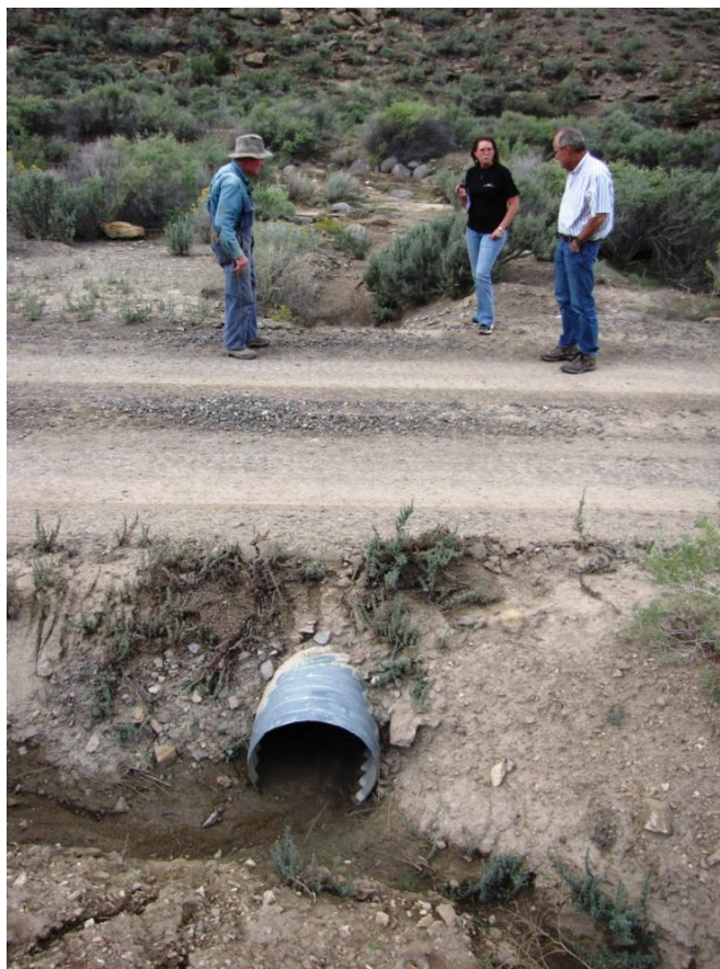
Photo No. 2 - Existing culvert at North Decline road requiring maintenance.
