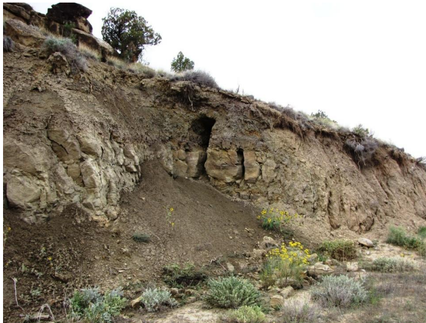
Photo No. 4 - Rockfall on cut slope above irrigation pipe location.
