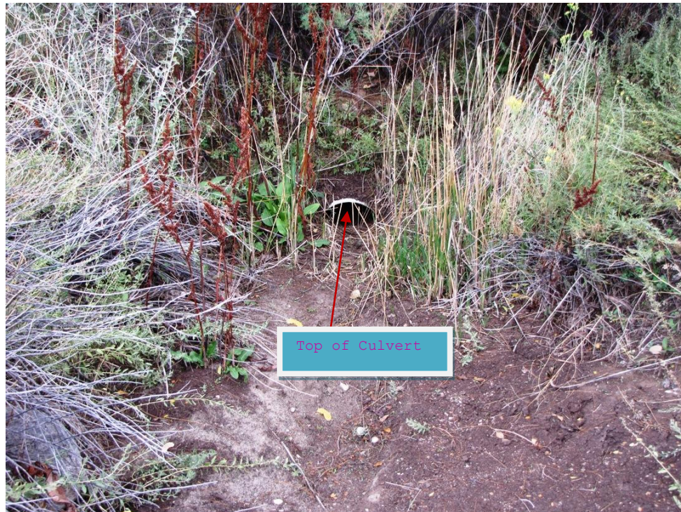
Photo No. 7 - Lower irrigation ditch culvert silted in.
