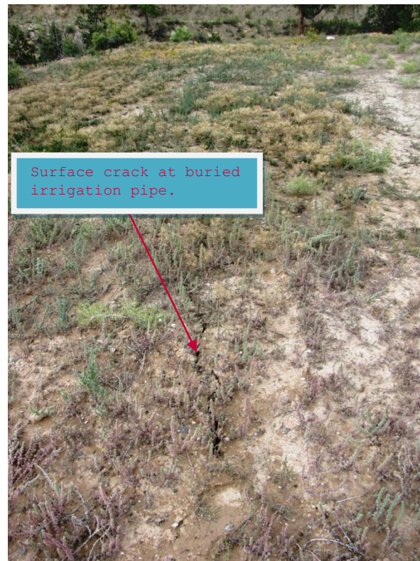
Photo No. 5 – Surface crack at location of buried irrigation pipe.
