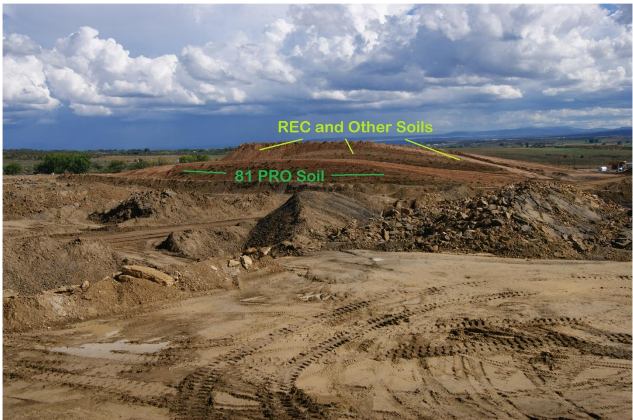
Photo 8 – Topsoil stockpiles, looking SE
