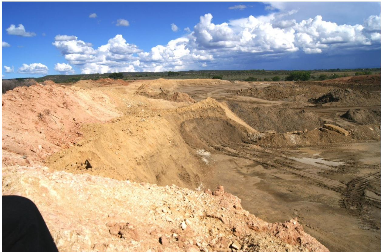
Photo 6 – Highwall, looking east
