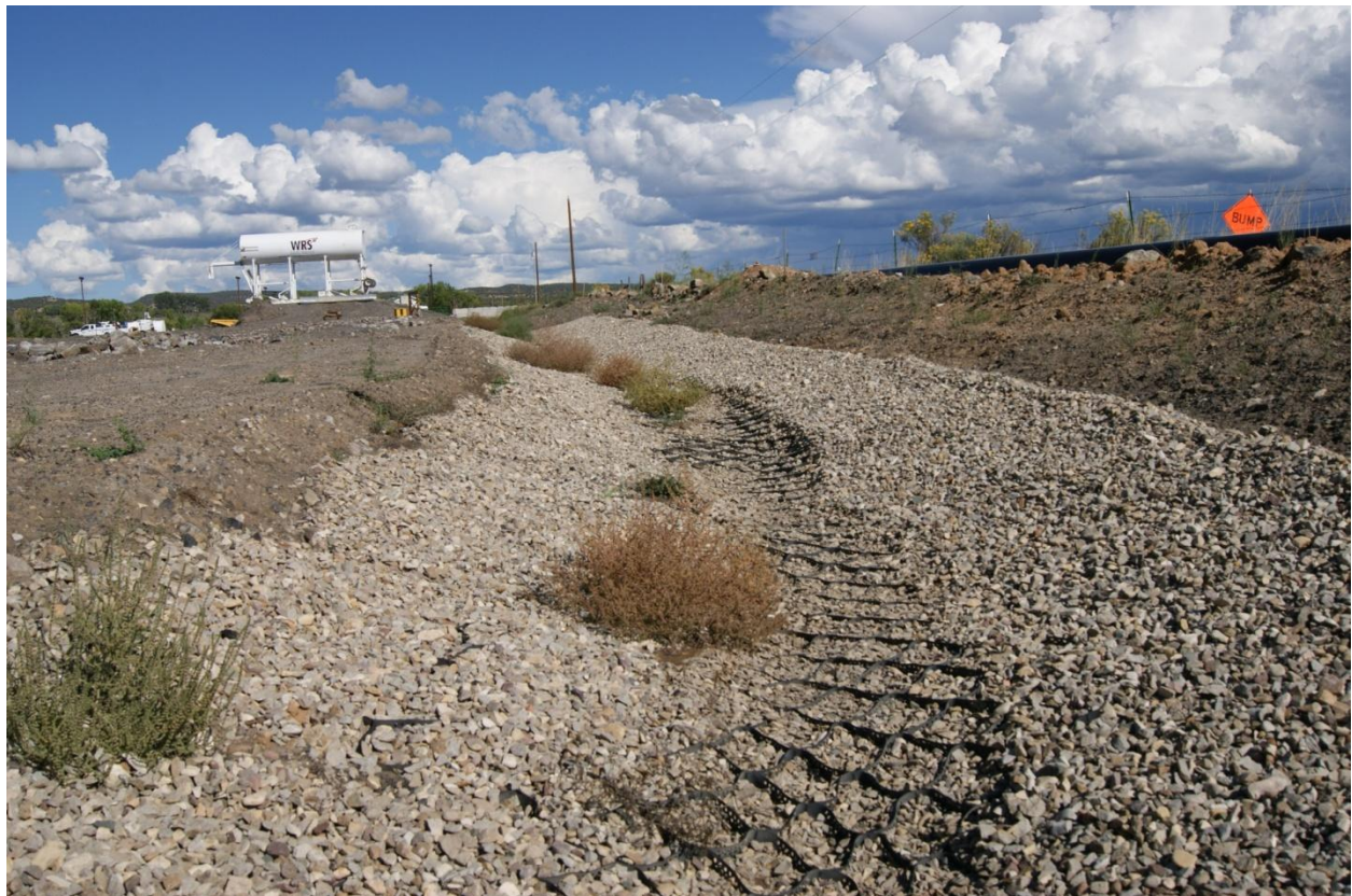
Photo 4 – Lined portion of Ditch NHN-001 East, west of mine entrance
