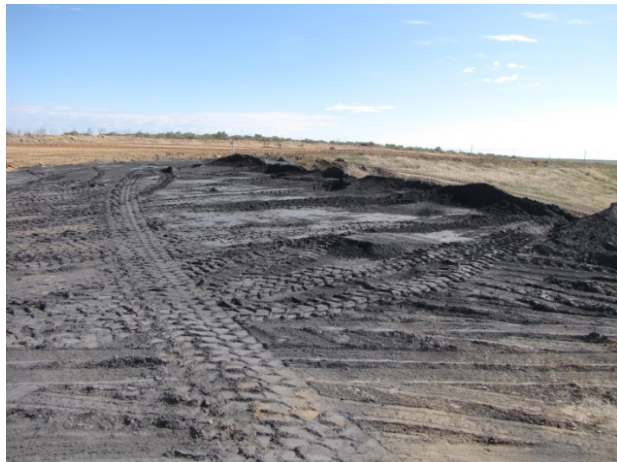
Photo 1 – Coal Ash Backfilled
