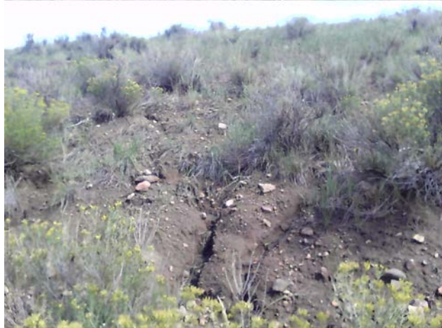
Photo 6: slope on northwest corner of truck tunnel requires stabilization.
