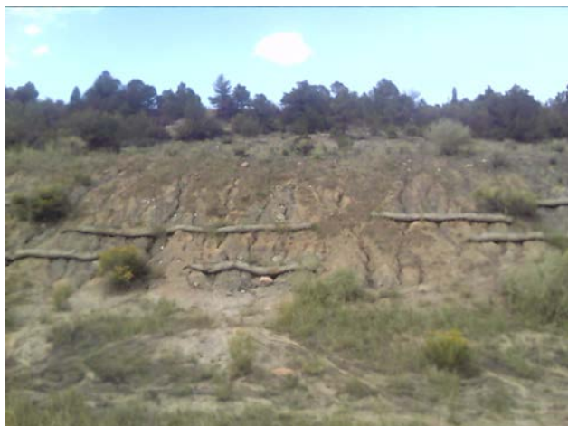
Photo 10: slope north of parking are. Slope and wattles need repair.
