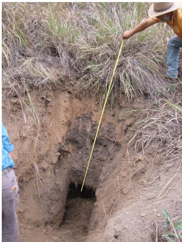
Photo 7 – Mine Adit 7.5 Feet Below Surface
