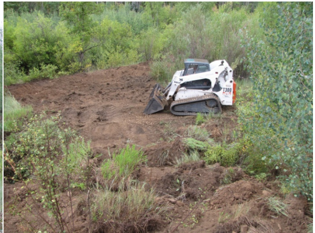
Photo 4 – Compacted Areas Roughened with Loader
