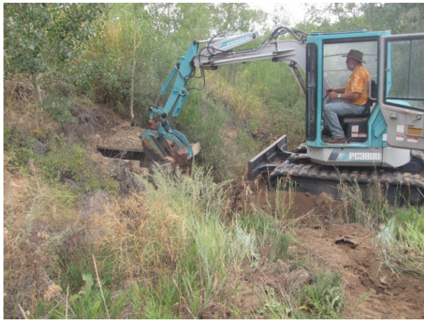
Photo 5 – Removing Wood Cribbing
