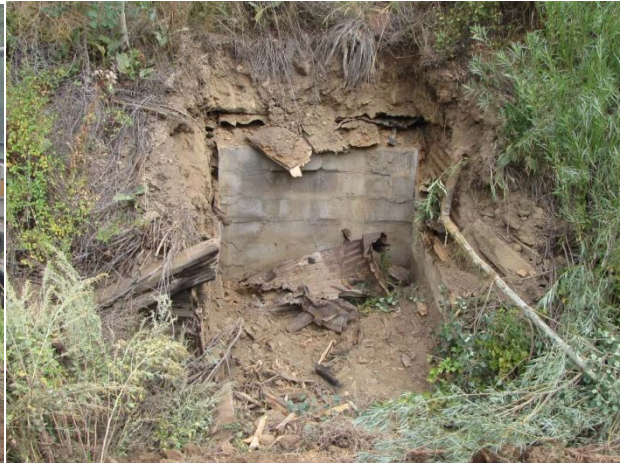
Photo 6 – Concrete Block Mine Seal
