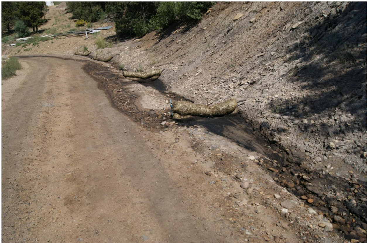
Photo 6 – Straw wattles in ditch on Belt Portal Access Road
