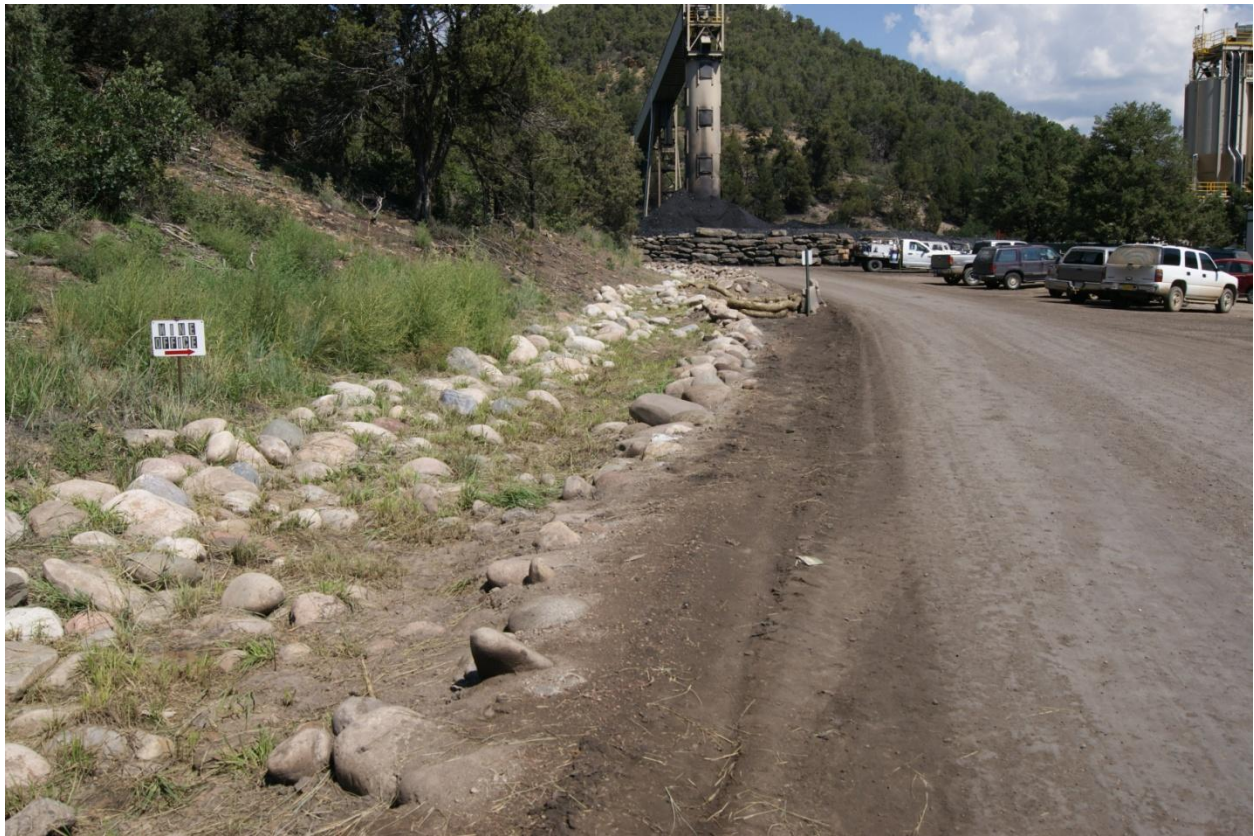
Photo 3 – Segment of West Clean Water Diversion where weeds have been removed
