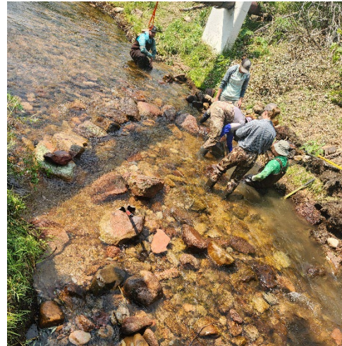
Figure 2 Hydrographers building a natural streamgage control South Boulder Creek above Howard Ditch
