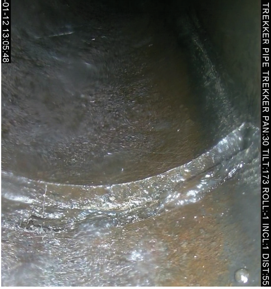
Photo 12 - Mechanical clamp at 55 ft
