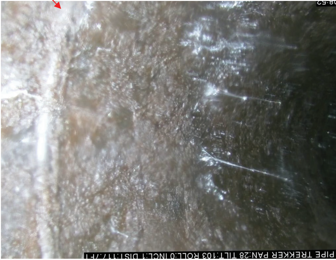
Photo 13 - Typical PE welded joint and webbing
