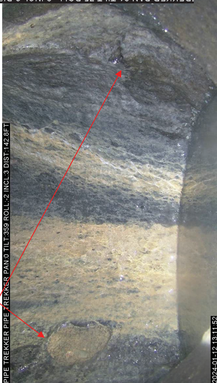
Pitting Photo 15 - South vertical intake pipe
