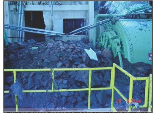
TURBINE HALL DAMAGE FROM PENSTOCK RUPTURE
