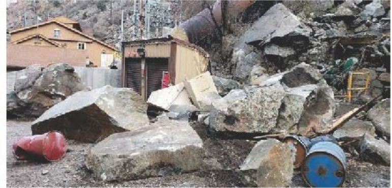
TURBINE HALL DAMAGE FROM PENSTOCK RUPTURE
