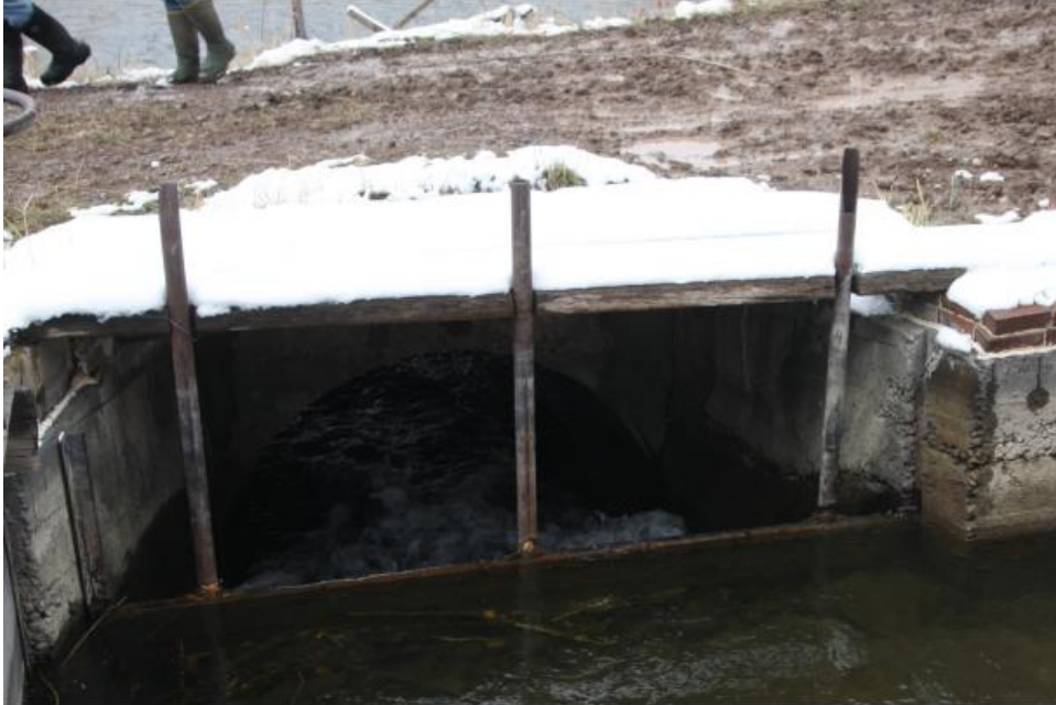
Diversion to river: Looking at old board slots and plank walkway.
