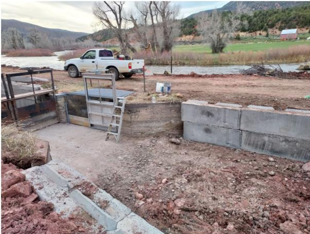
Concrete blocks were installed to control erosion both on both sides of embankment on both the upstream and downstream side of main structure.
