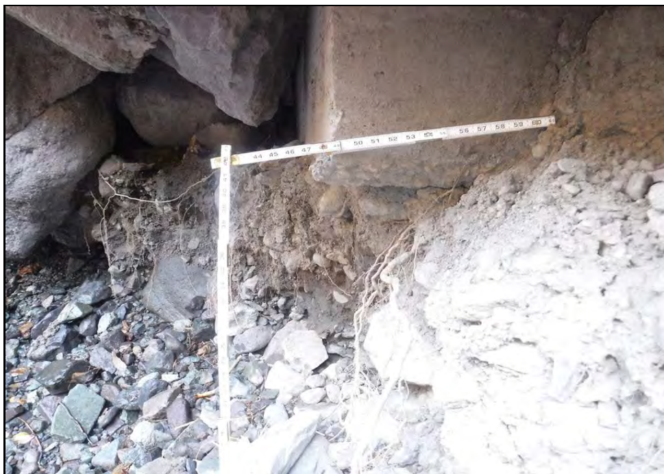
East end of Abutment 2 footing undermined 10 inches horizontally to the north
