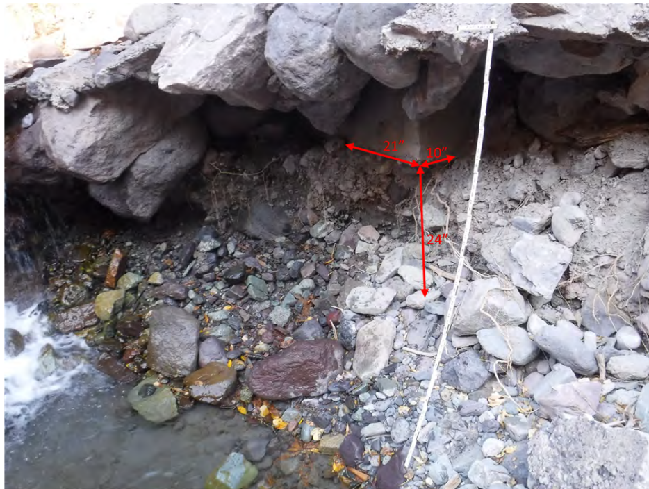
Photo 8 – Overview of exposed footing showing measurements of the extent of undermining
