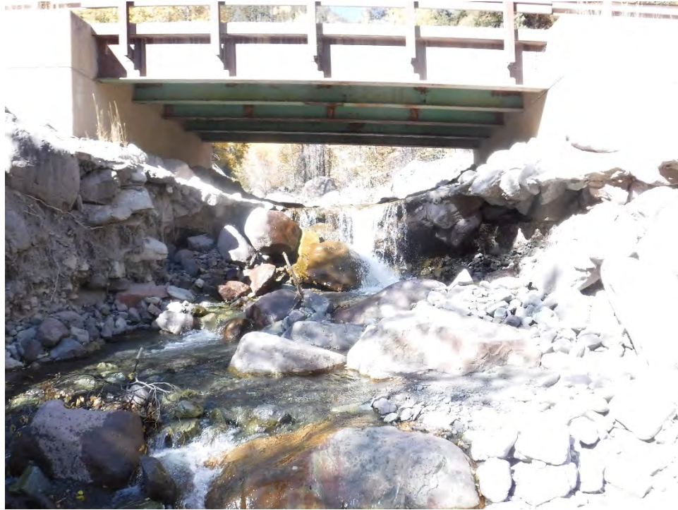
Photo 3 – Overview of channel headcut in 2019
