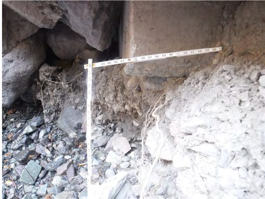
Photo 5 – East end of Abutment 2 footing undermined
