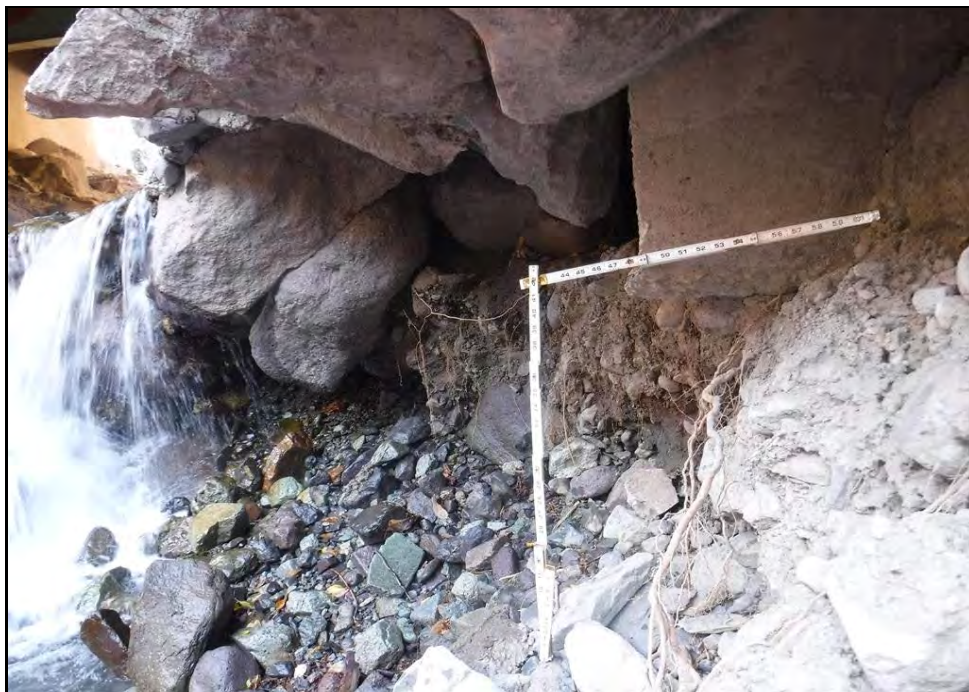
East end of Abutment 2 footing undermined 24 inches vertically
