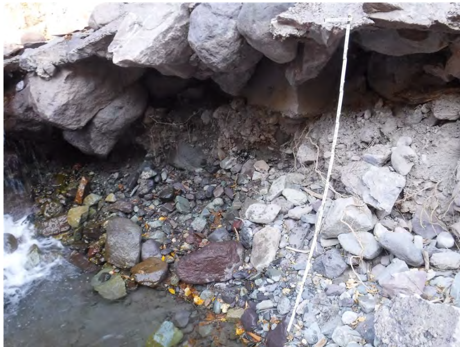
Photo 4 – Grouted rip rap at Abutment 2 undermined up to 6 ft vertically, footing exposed
