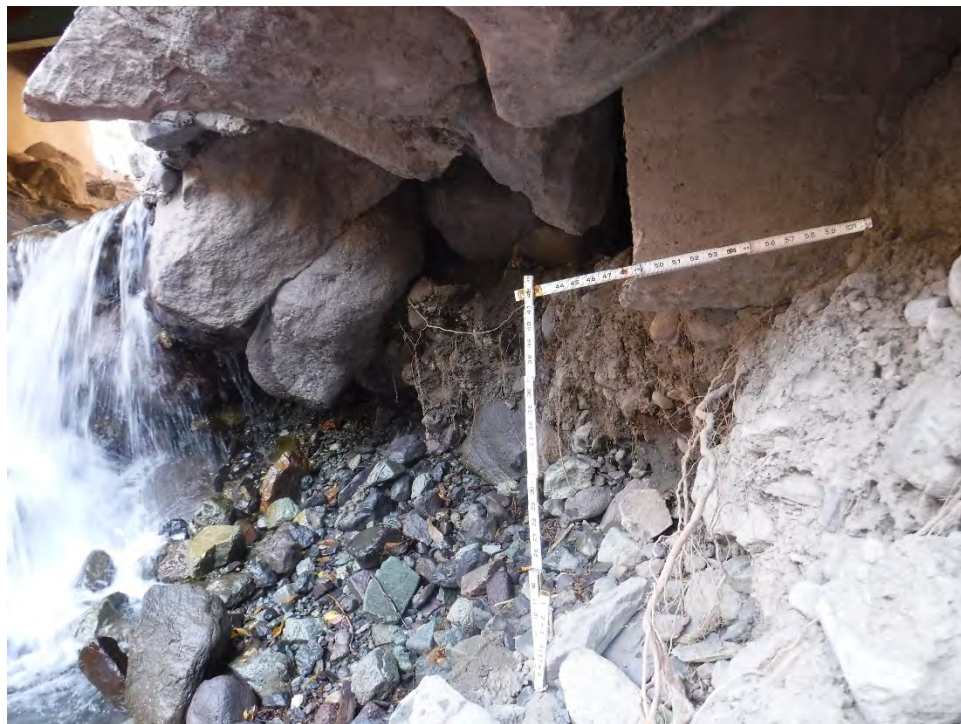
Photo 8 – The east corner of the North Abutment footing is undermined 24 inches vertically
