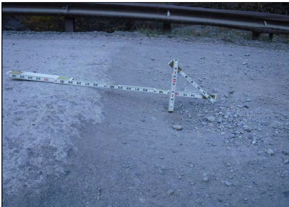
2.5 inch drop to roadway at north end
