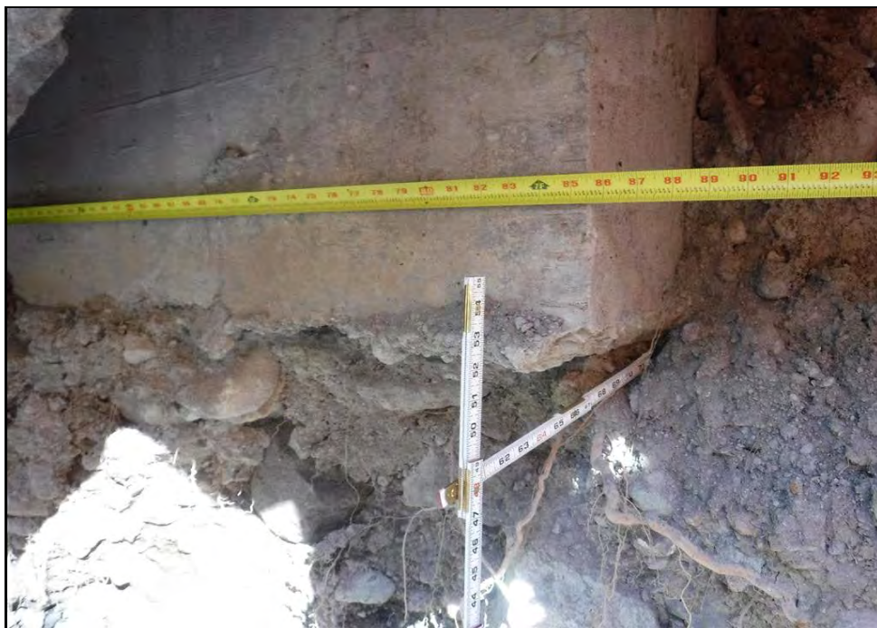
East end of Abutment 2 footing undermined 7 ft 1 inch horizontally to the west
