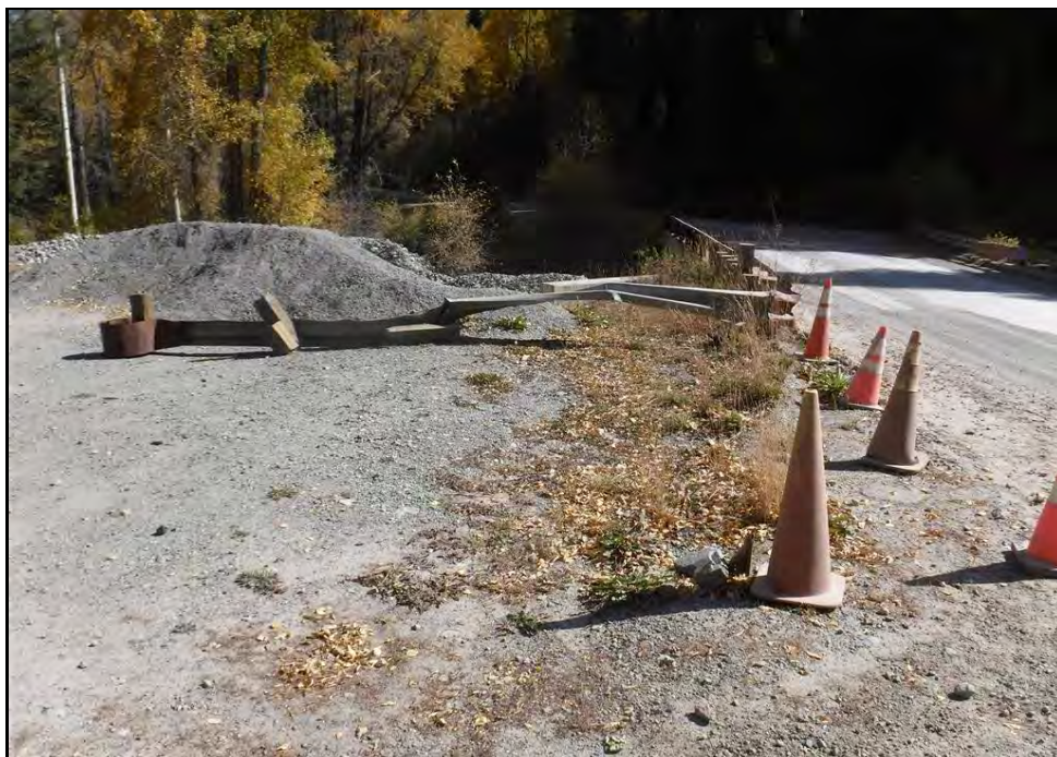
Damage of southwest rail
