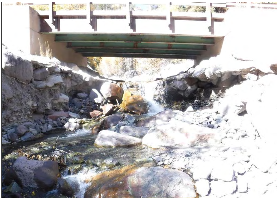
Overview of scour at east side of structure
