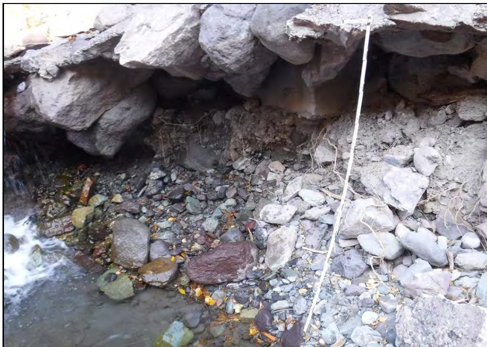
Grouted rip rap at Abutment 2 undermined up to 6 ft vertically
