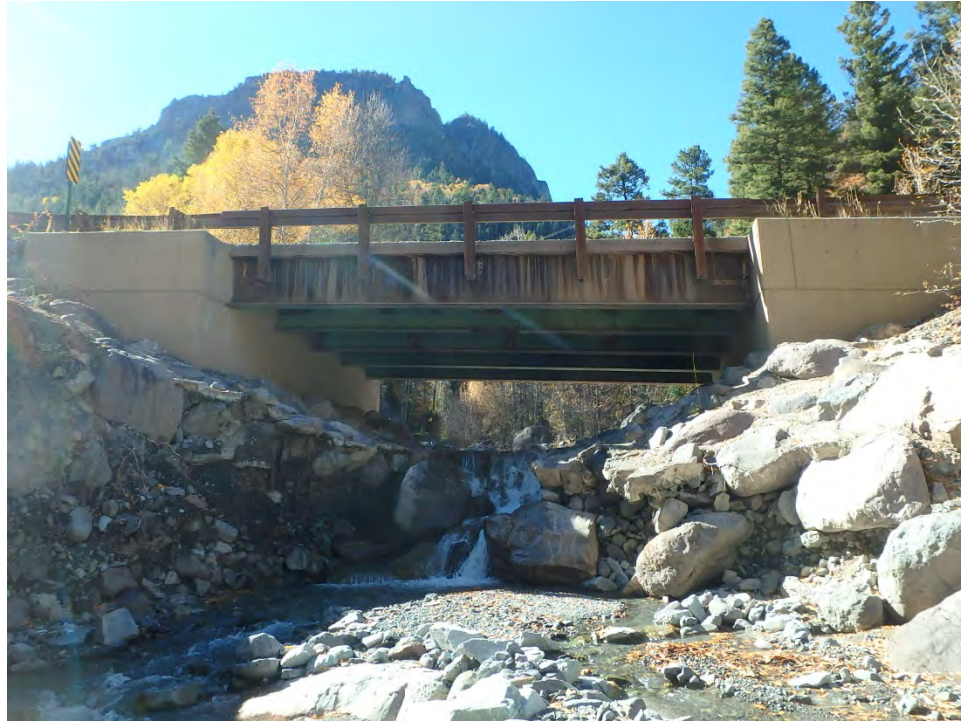
Photo 4 – Overview of channel headcut in 2017 (from previous inspection report)
