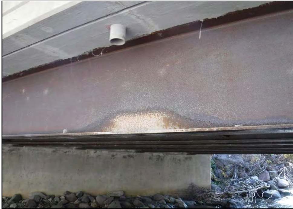
R1 corrosion of girder below deck drain
