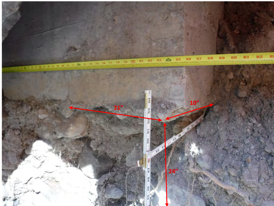
Photo 8 – Close-up of exposed footing showing measurements of the extent of undermining
