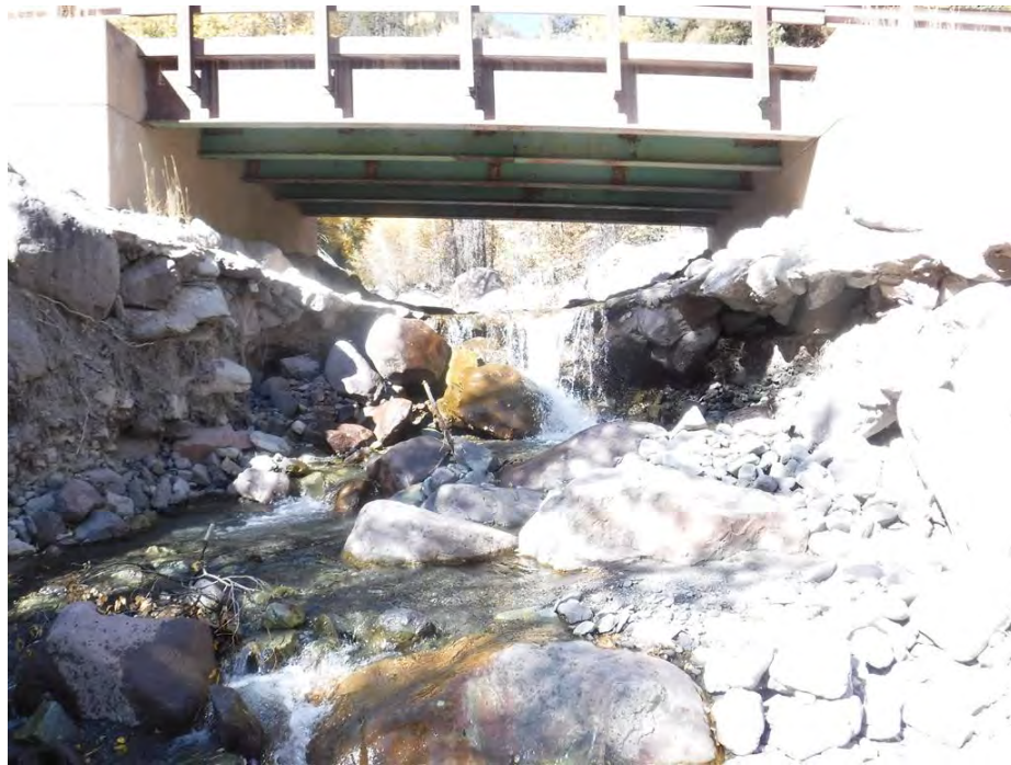
Photo 3 – 6 foot high headcut in channel at downstream side of bridge
