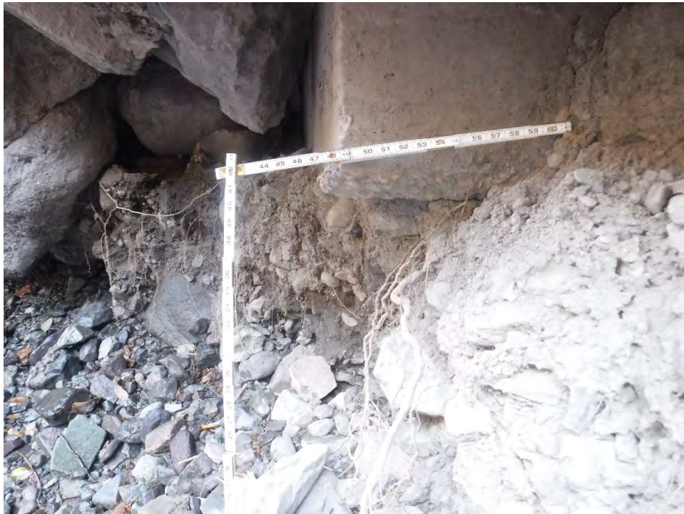
Photo 6 – The east face of the North Abutment footing is exposed and undermined
