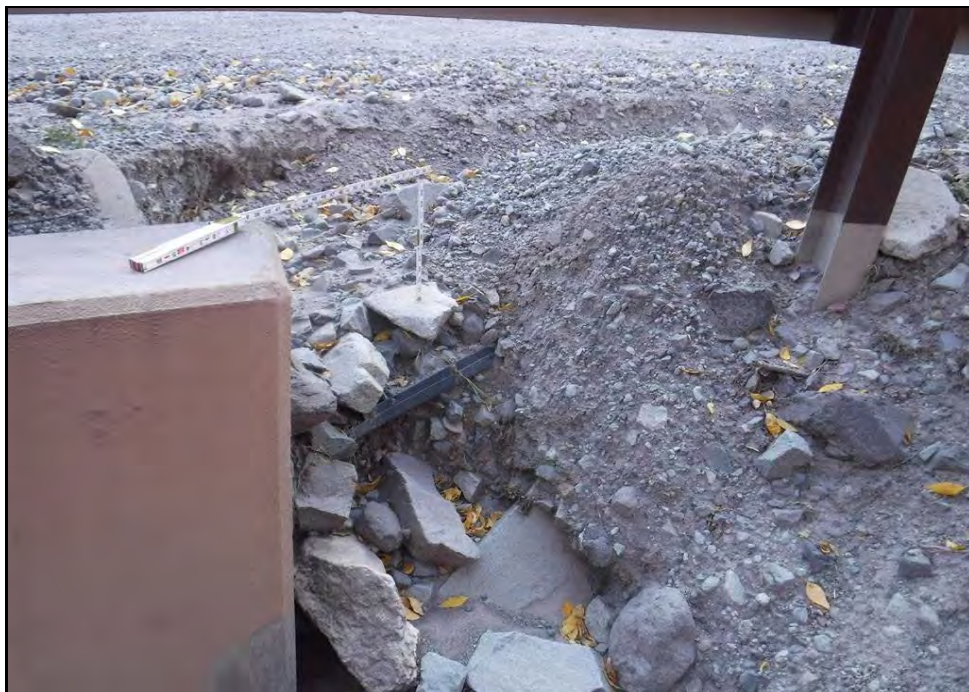
Erosion at southwest wingwall
