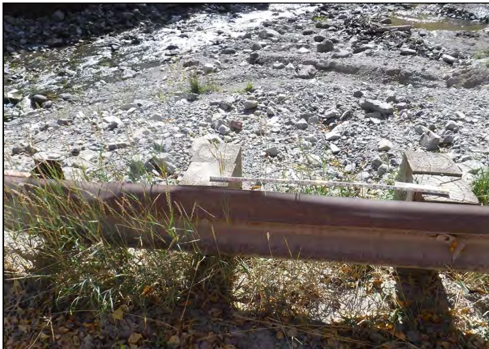
Approach rail transitions have inadequate post spacing and are not double nested
