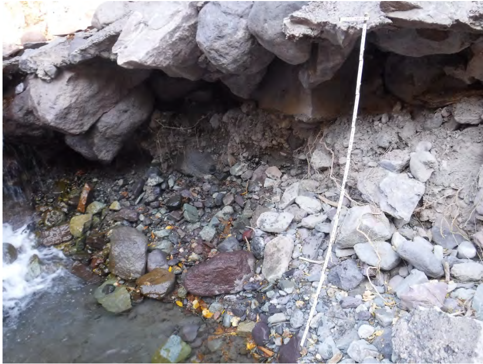
Photo 5 – The grouted riprap at along the east side of the structure (downstream side) is undermining up to 6 ft
