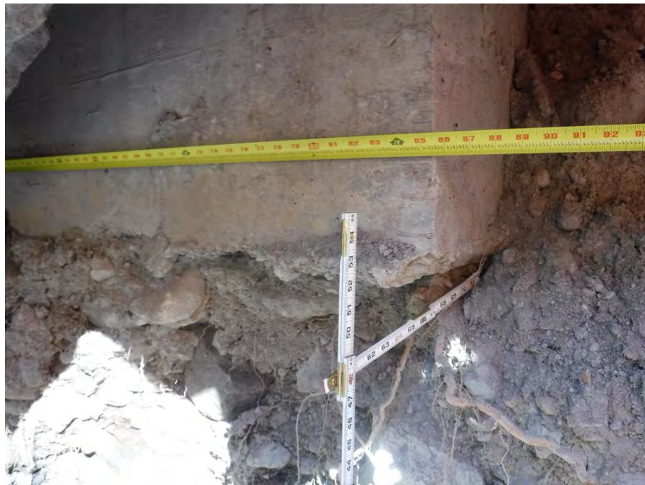
Photo 6 – Close-up view of the undermined east corner of the North Abutment
