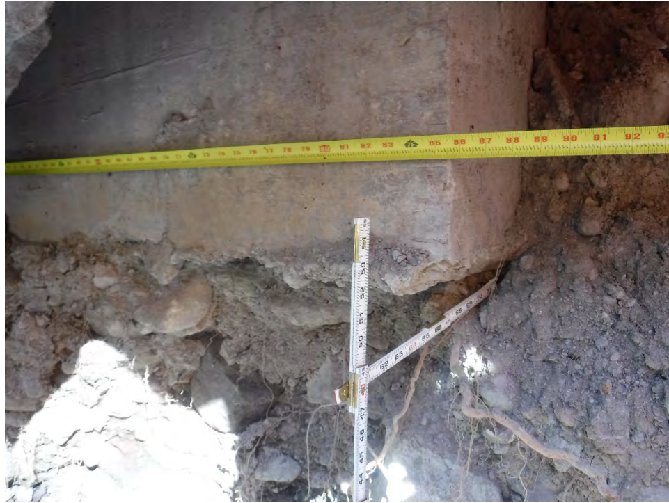
Photo 7 – Close-up view of the undermined east corner of the North Abutment
