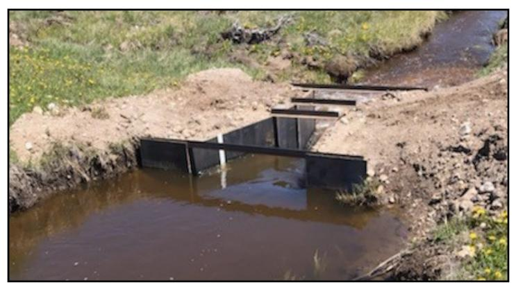
This 30 inch wide steel measuring device replaces the old rusted out structure on the Darling ditch and allows the water user to properly measure the amount of water in the ditch.
