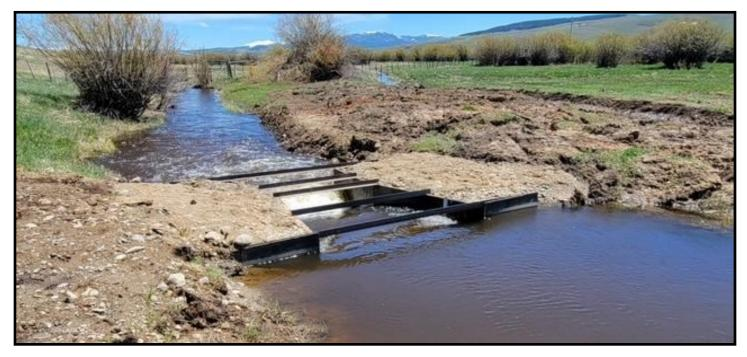
This 5 foot wide steel measuring device replaces the old rusted out structure on the Nairin ditch. Located directly the headgate, it allows the water user to properly measure the amount of water in the ditch.
