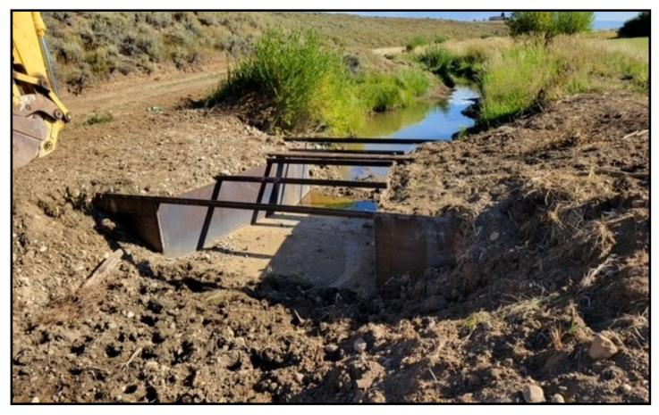
This 6 foot wide steel measuring device replaces the old wooden structure on the 969 ditch. Located just below the new headgate, it allows the water user to properly measure the amount of water in the 969 ditch.
