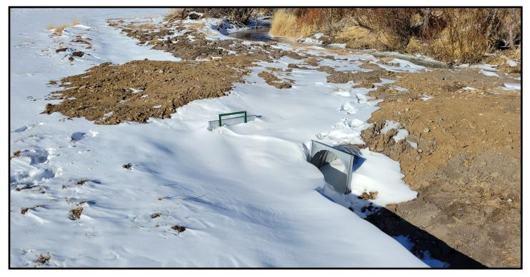
This 24' x 20' new check and turnout pair, with aluminum slide gates, simplifies the water users effort to check and utilize the water in the Willow ditch more efficiently.
