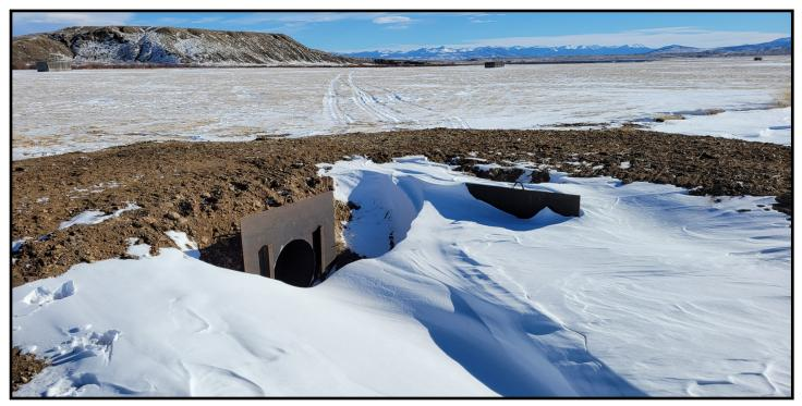
This 24' x 20' new check and turnout pair, with 4 x 4 steel headwall for check boards, simplifies the water users effort to check and utilize the water in the staples ditch more efficiently.
