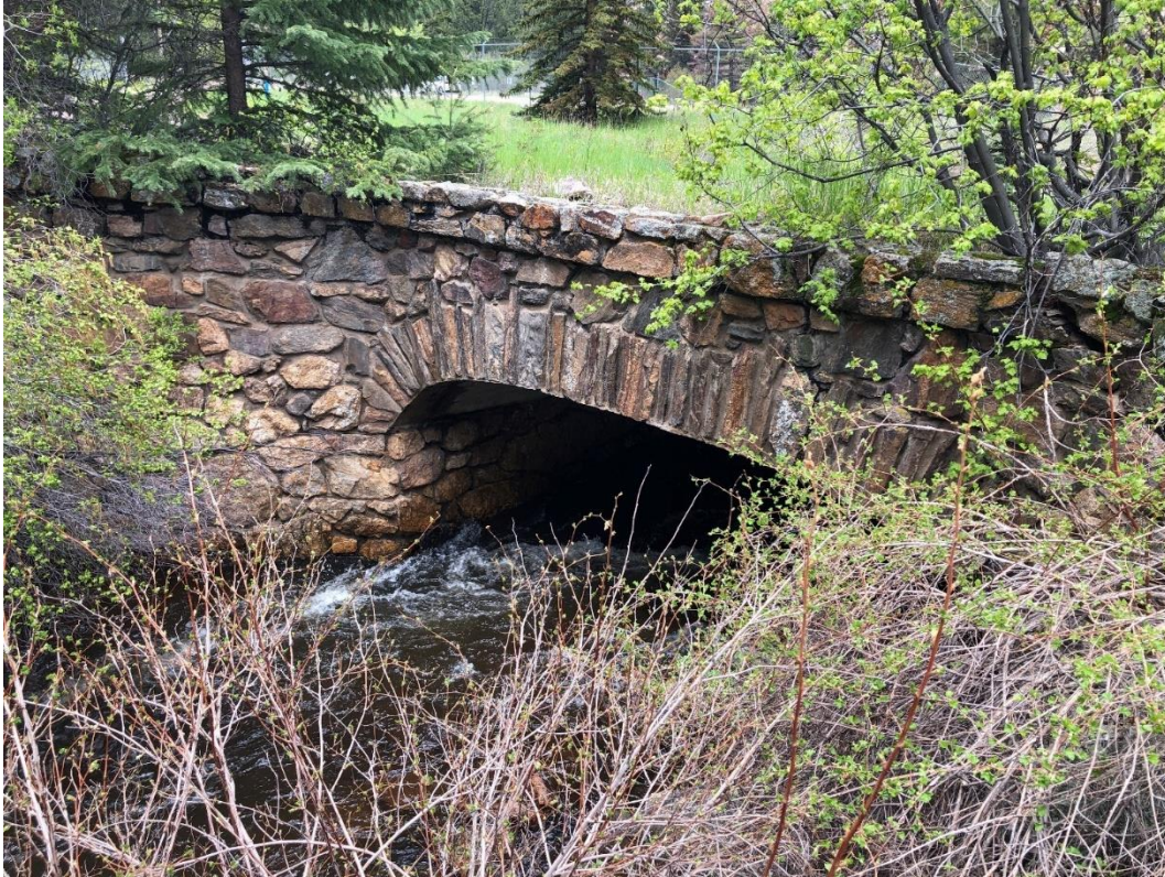
Figure 6 – Historic stone bridge located across State Highway 103 and possibly associated with 5CC.1151, facing northwest.
