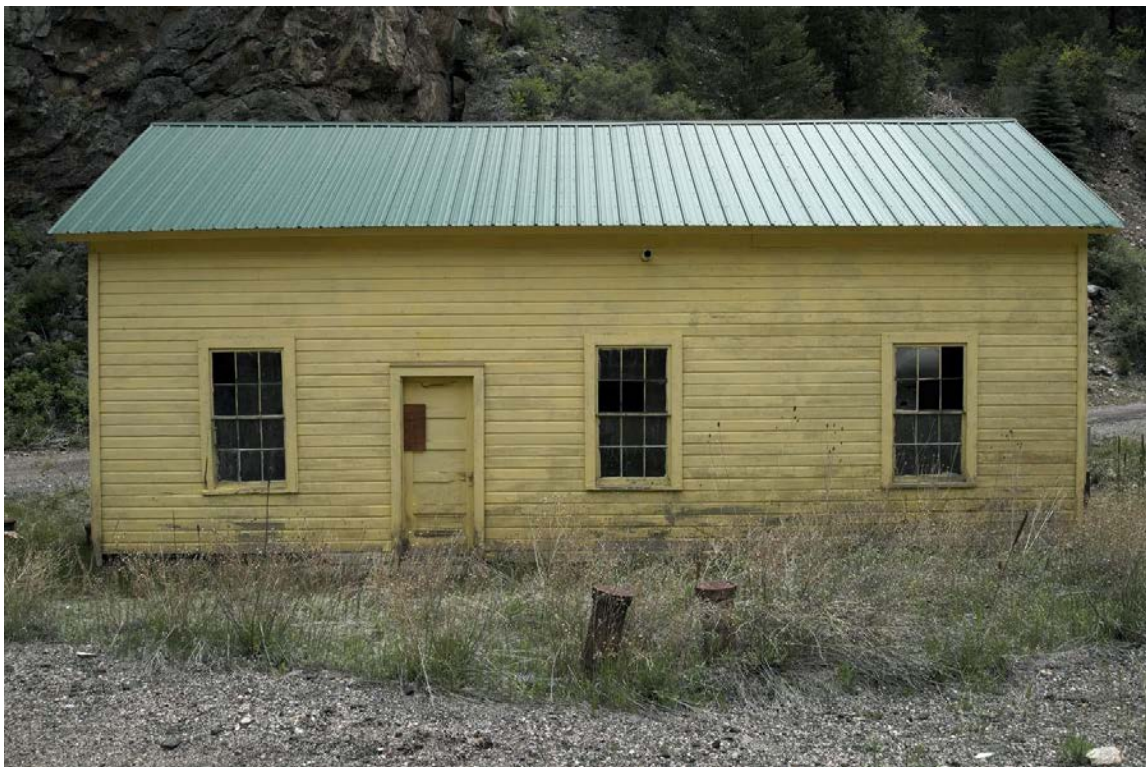
Figure 7 – Original structure (circa early 1900s) at the City of Idaho Springs Water Treatment Facility, facing southeast.
