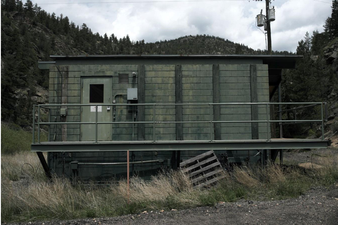
Figure 8 – 1969 structure at the City of Idaho Springs Water Treatment Facility, facing north/northwest.
