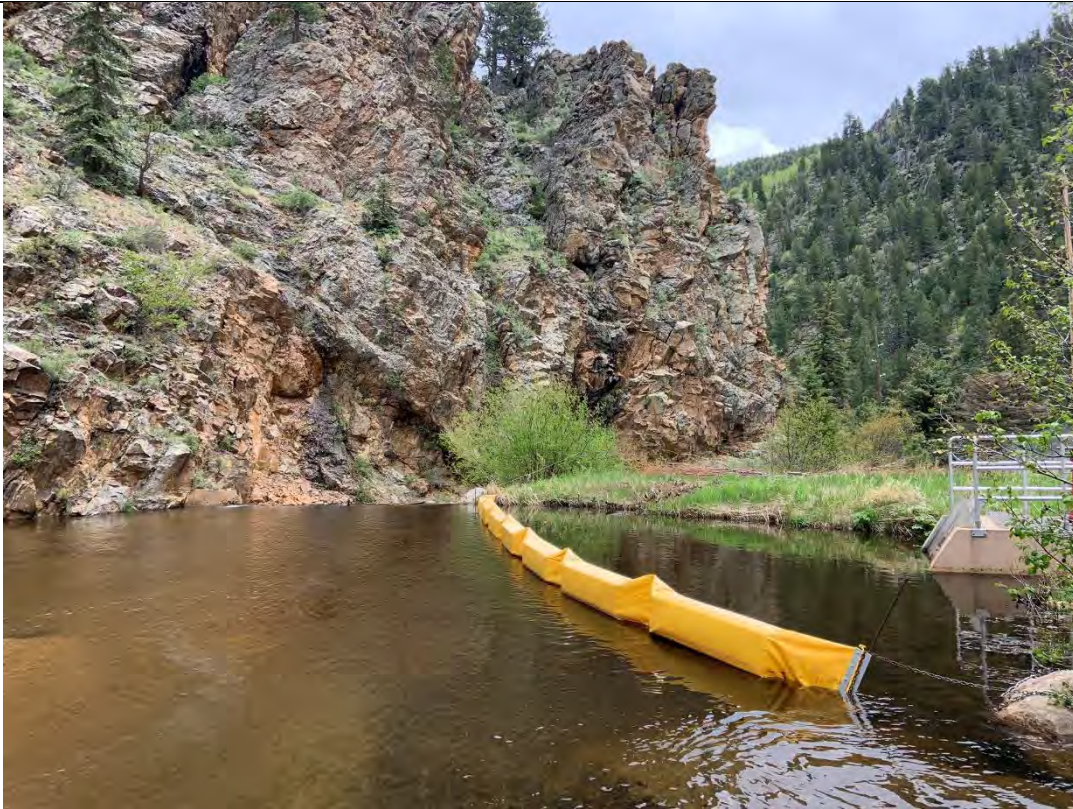
1. Overview of Mattie Dam, looking downstream. Stream overflow structure is just left of willow in center. Water intake structure is on right.
