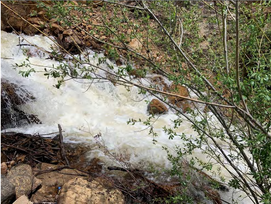
3. Chicago Creek just downstream of dam crest, in area stabilized with riprap.
