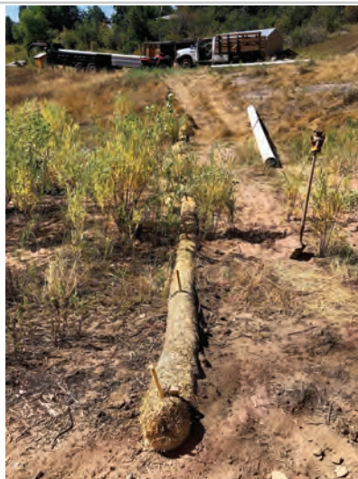
A sediment control log has been added at a strategic location where disturbances of concern drain drain to a channelized area.
