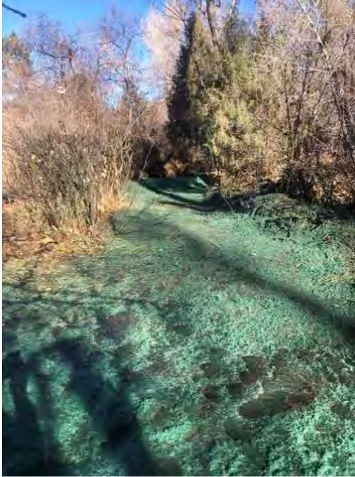
Figure 1-Fresh hydromulch after seeding in riparian section
