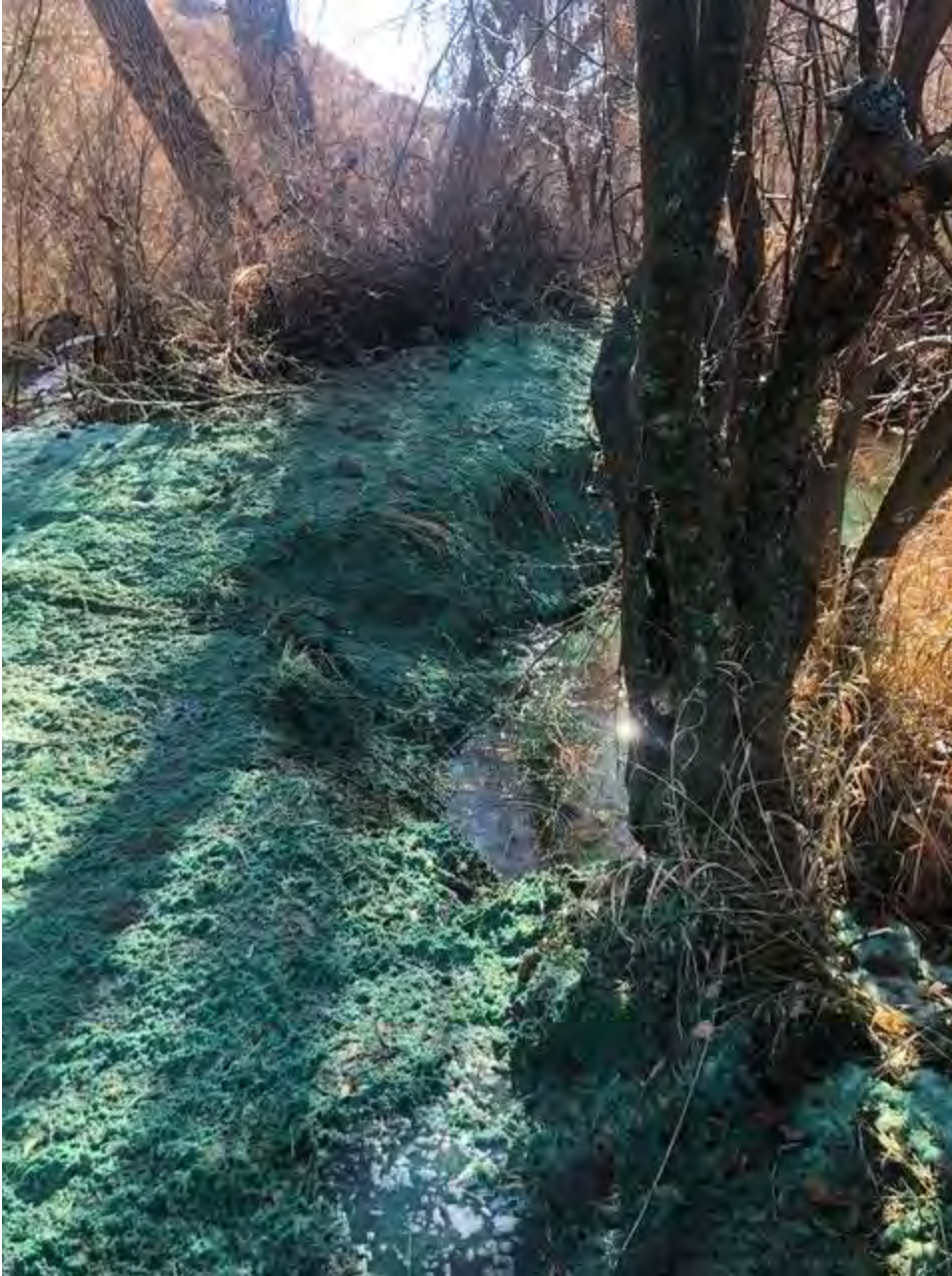
Figure 10 - Hydroseeding Sousy ditch following pipeline installation
