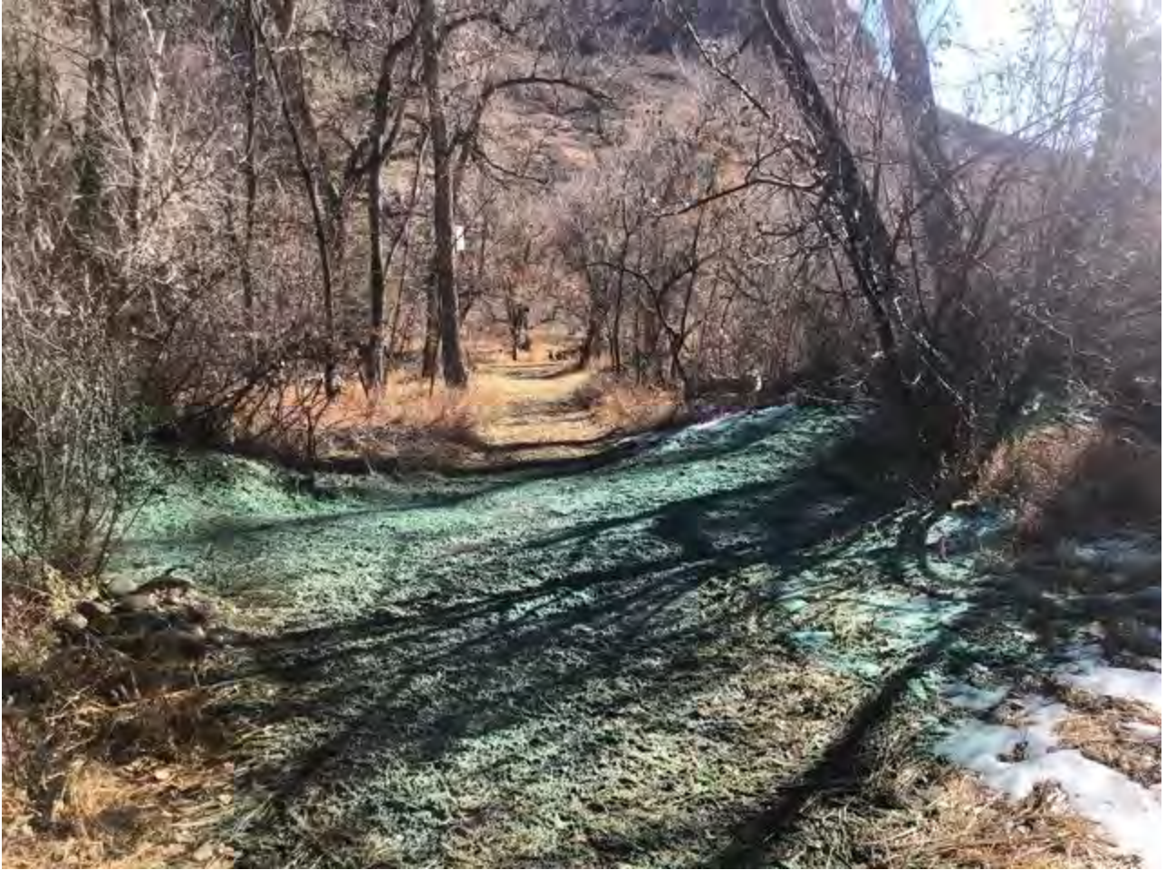
Figure 11 - Hydromulch lower section of project
