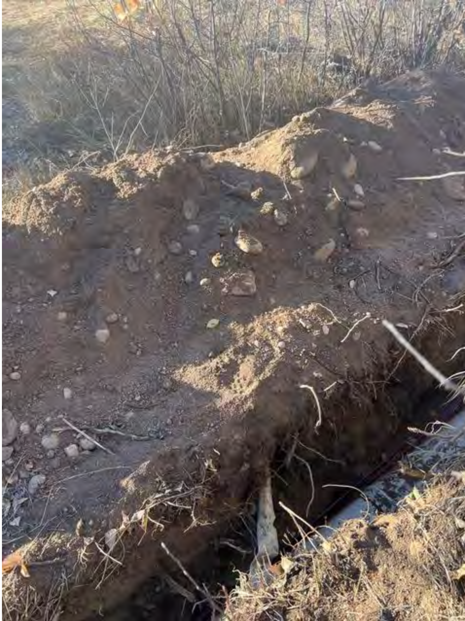
Figure 8 - 10" PVC pipe in ditch prior to backfill
