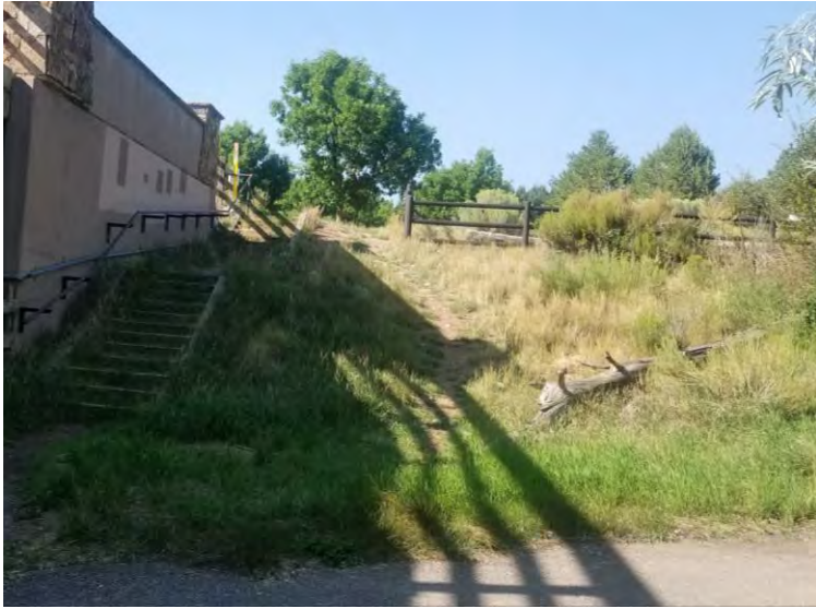
Pre- Construction Summer, 2018
