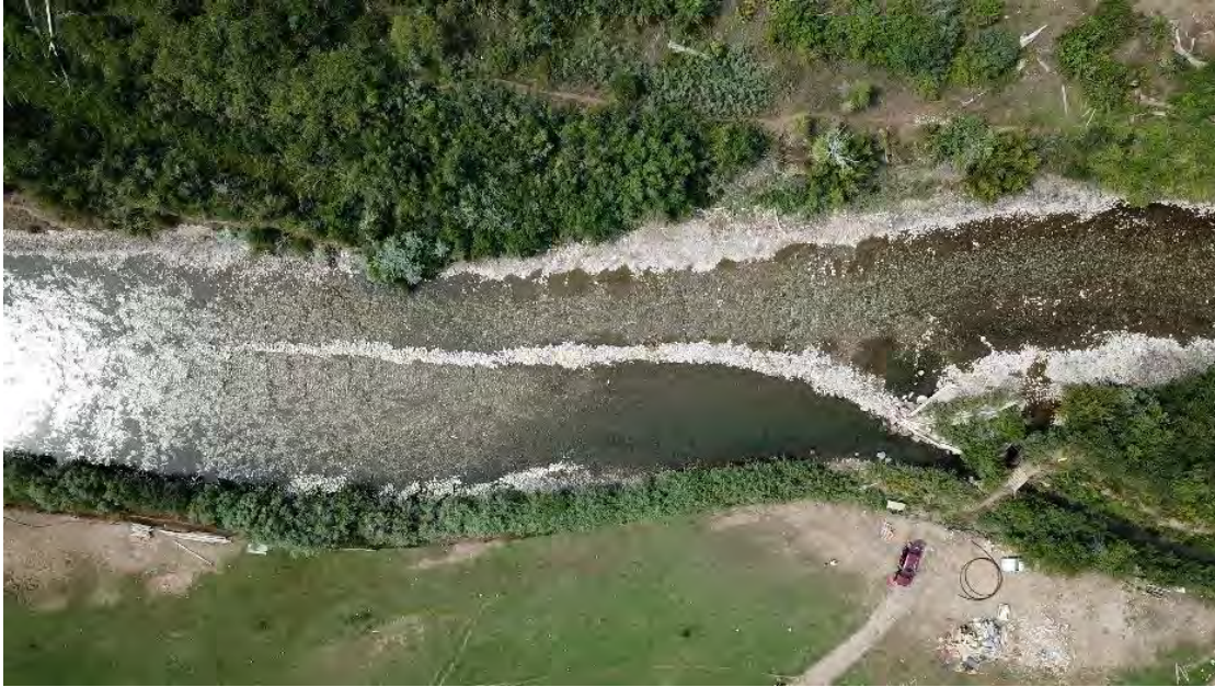
Pre- Construction Summer, 2018
