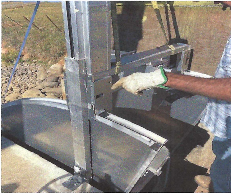
Figure 3 Lowering headgate into bracket on Oct 9th
