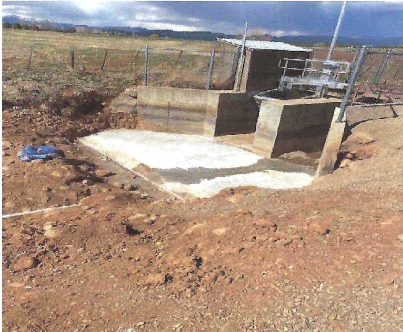
Figure 6 Extending concret splash pad March 2025
