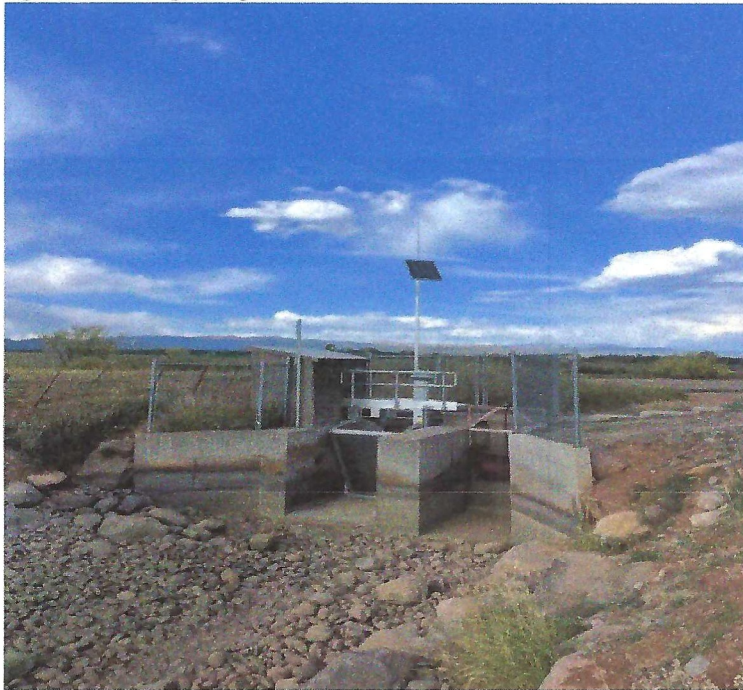
Figure 4 Pastorius headgate installed and commissioning completed Oct 9th.
