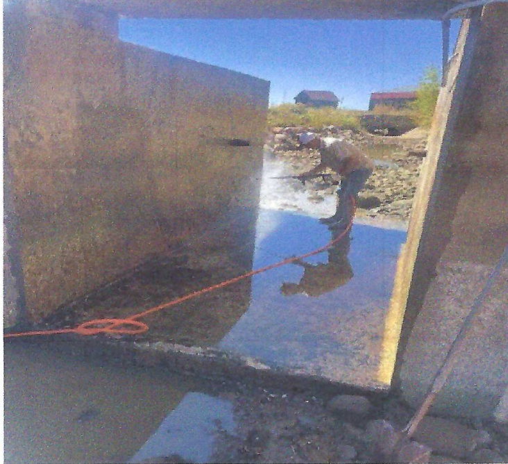
Figure 1 Power washing concrete to remove loose debris/organics a week ahead of time to allow time for concrete to dry thoroughly.
