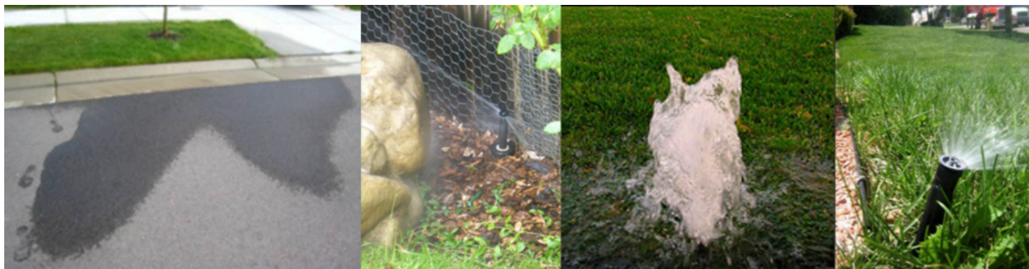
A variety of irrigation issues requiring simple maintenance: overspray, blocked nozzle, broken sprinkler head, and tilted head, via https://resourcecentral.org/sprinklers/sprinkler-maintenance .
