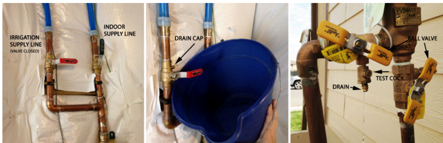
Common components of an irrigation system, via https://crconserve.com/254/Fall-Landscape-and-Irrigation-Prep .
