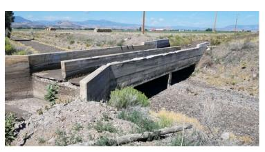
structures that would allow water in their canal to flow underneath the Rio Grande Canal.
