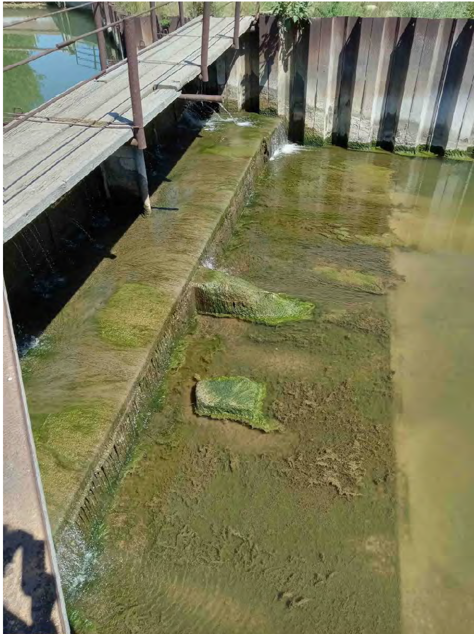
Fig. 4: Structure floor and downstream scour pad (from south abutment).
