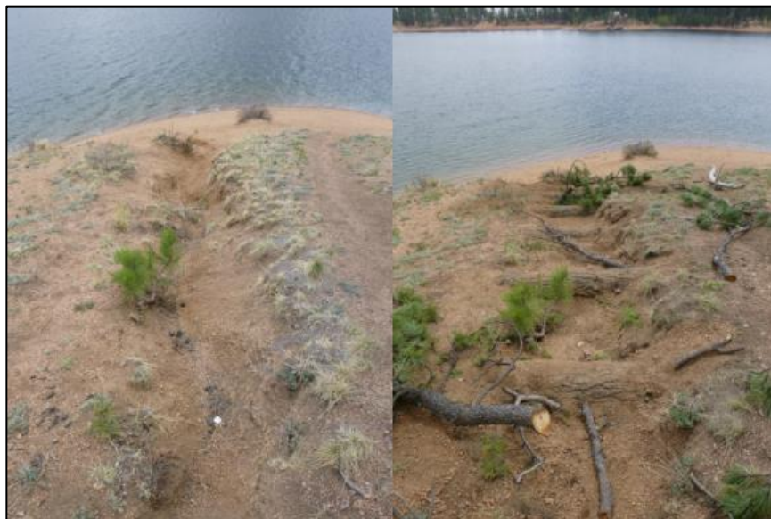
Before and after of check dam installation
