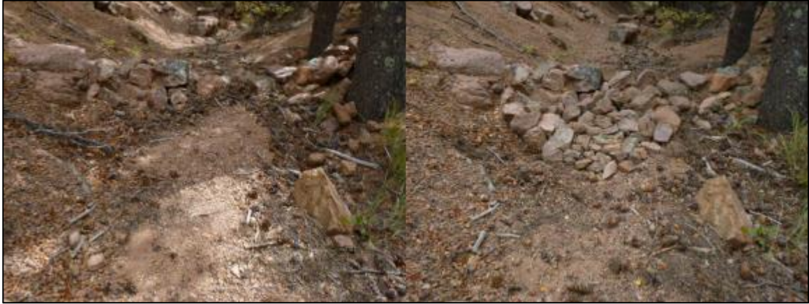
Before and after of fortified check dam
