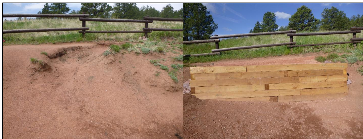
Before and after of retaining wall construction
