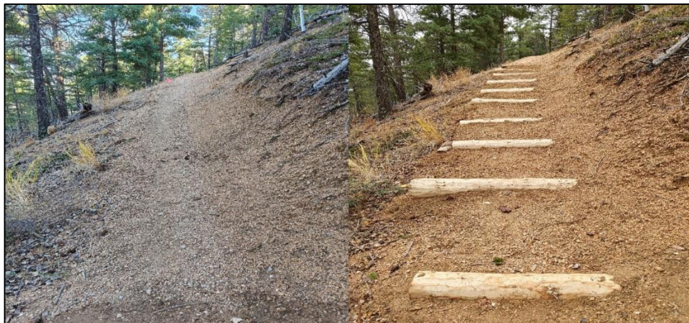
Before and after of check installation
