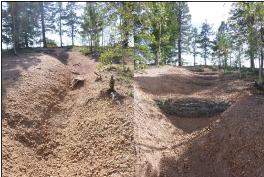
Before and after of check dam installation
