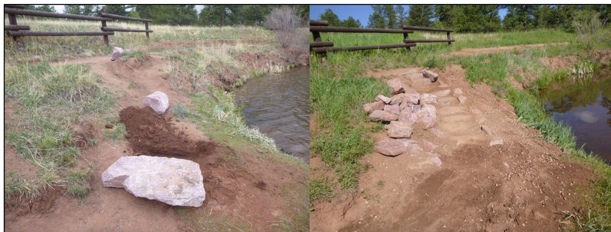
Before and after of rock step construction
