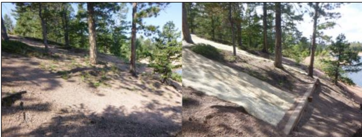
Before and after of retaining wall construction and erosion control matting installation
