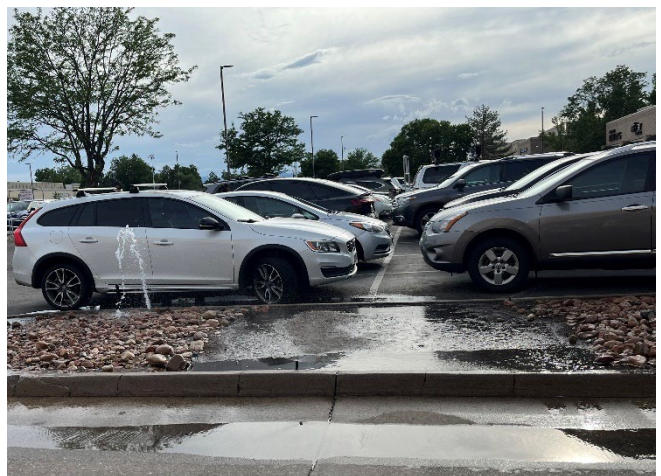
Photo 6. Commercial parking lot median converted to rock and bare ground with irrigation still occurring and running off into gutter, along with broken sprinkler heads.
