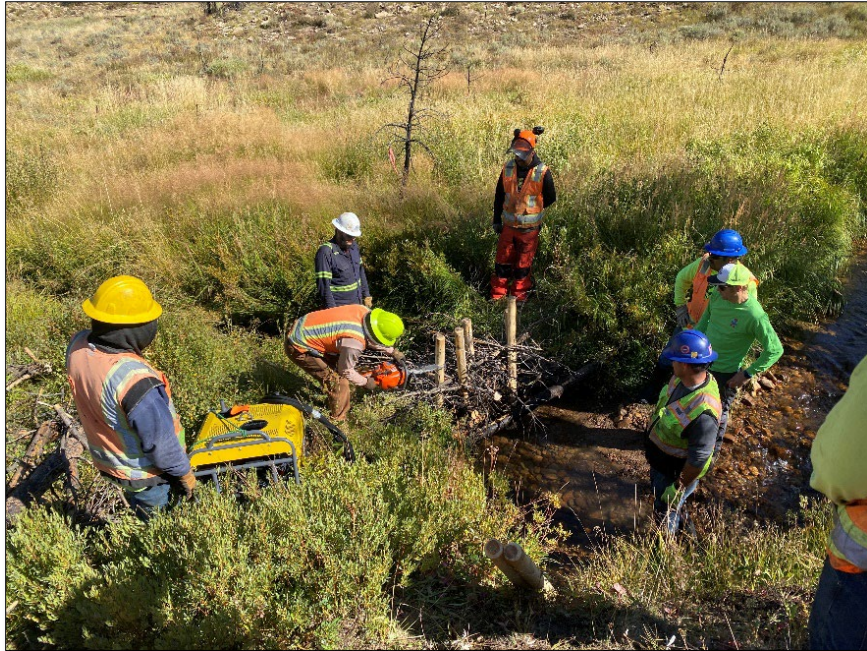
Installation of PALS on Kauffman Creek
