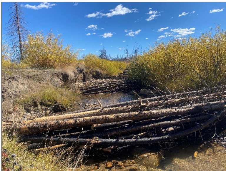
Constructed PALS on Stillwater Creek
