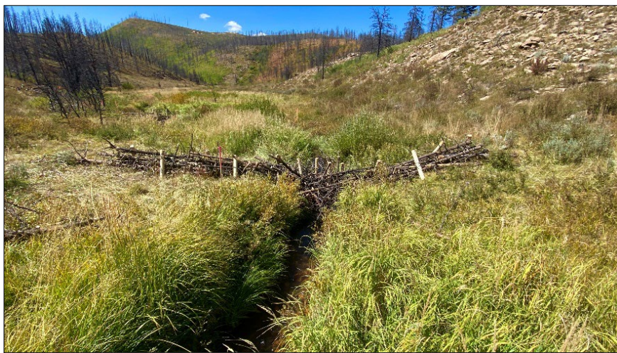
Constructed PALS on Kauffman Creek
