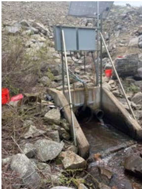
Photos 25 & 26: Jetting outlet works conduit. Multiple passes were made until debris and dirty water were no longer observed to be discharging from conduit.
