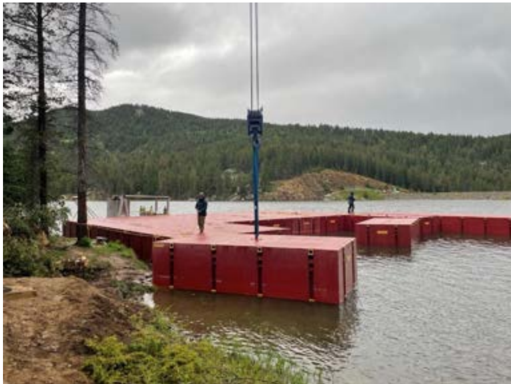
Photo 7: Contractor working on assembly of barge segments.
