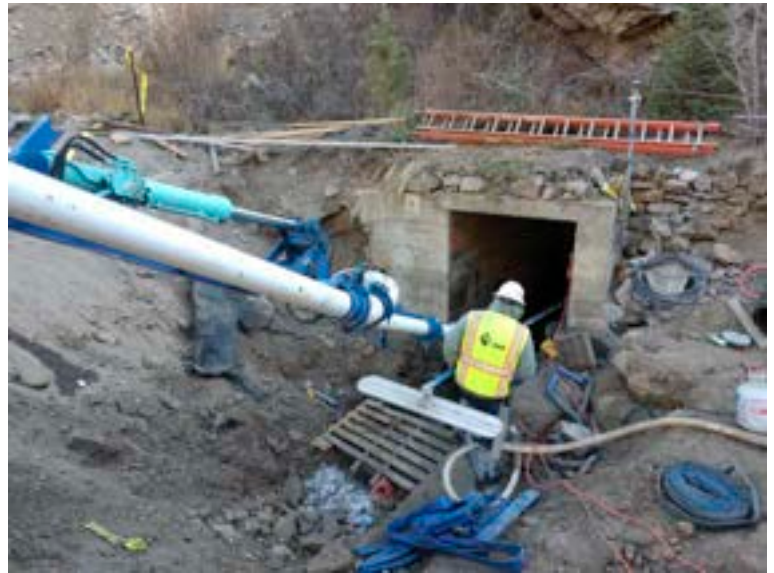
Working to fill and seal the man tunnel
