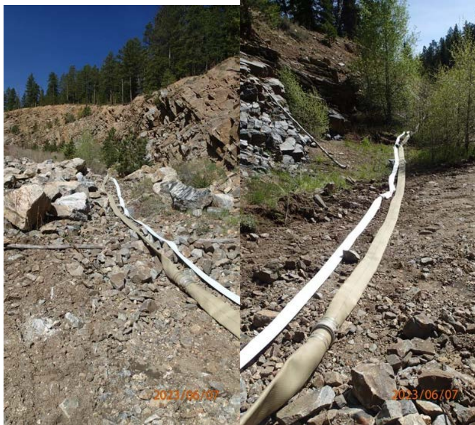
Photo 5: Bypass hoses setup along spillway.
