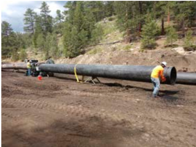
Bypass pipe to carry flow of Beaver Brook through site
