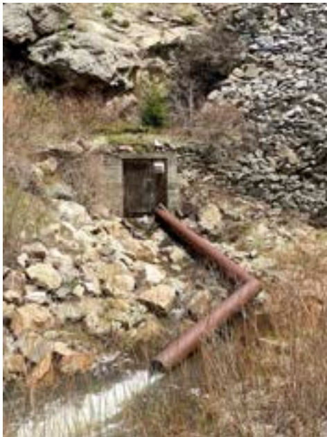
Outlet Pipe from man tunnel
