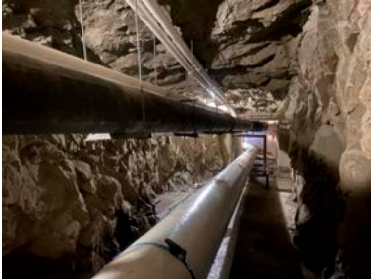
New outlet pipes in man tunnel
