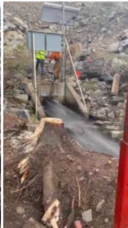
Photos 25 & 26: Jetting outlet works conduit. Multiple passes were made until debris and dirty water were no longer observed to be discharging from conduit.
