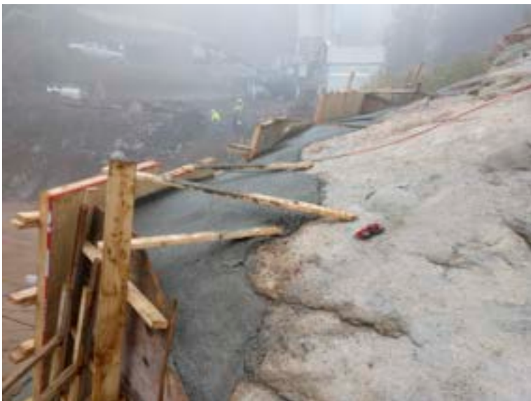
Dental concrete on outer upper edges of dam site
