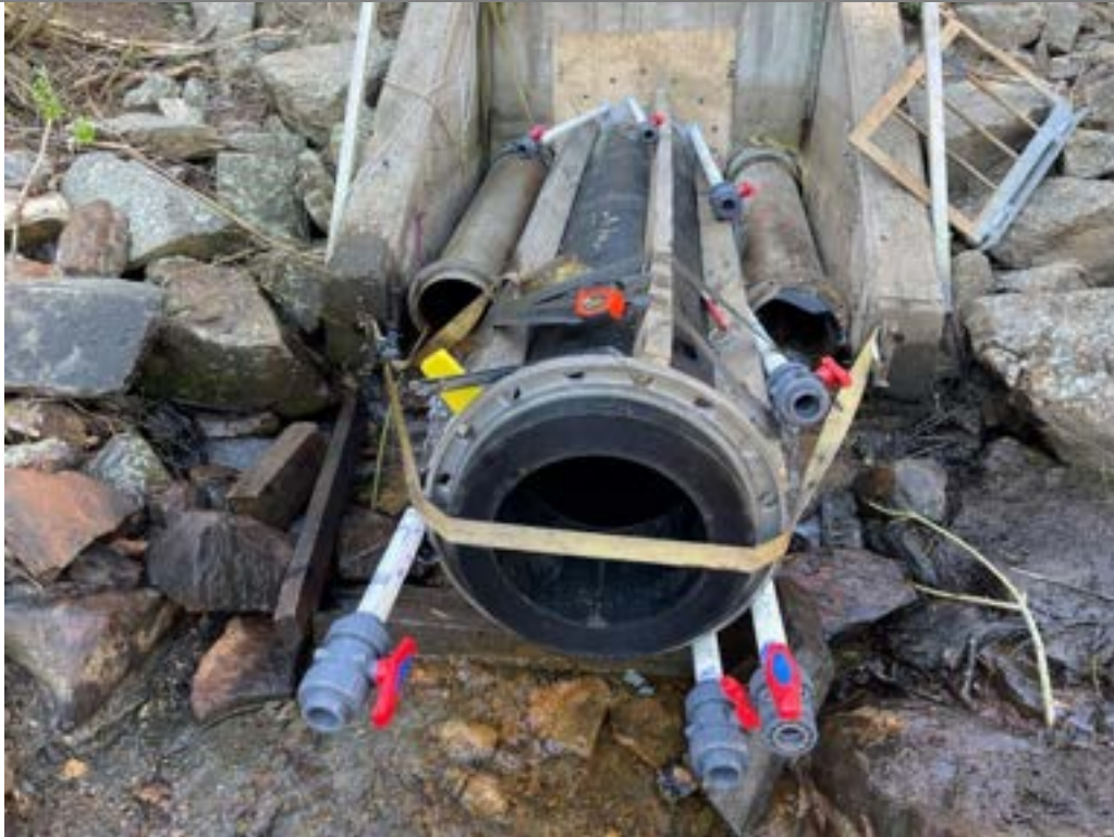
Photo 1: Downstream bulkhead and grout injection / vent pipe assembly.
