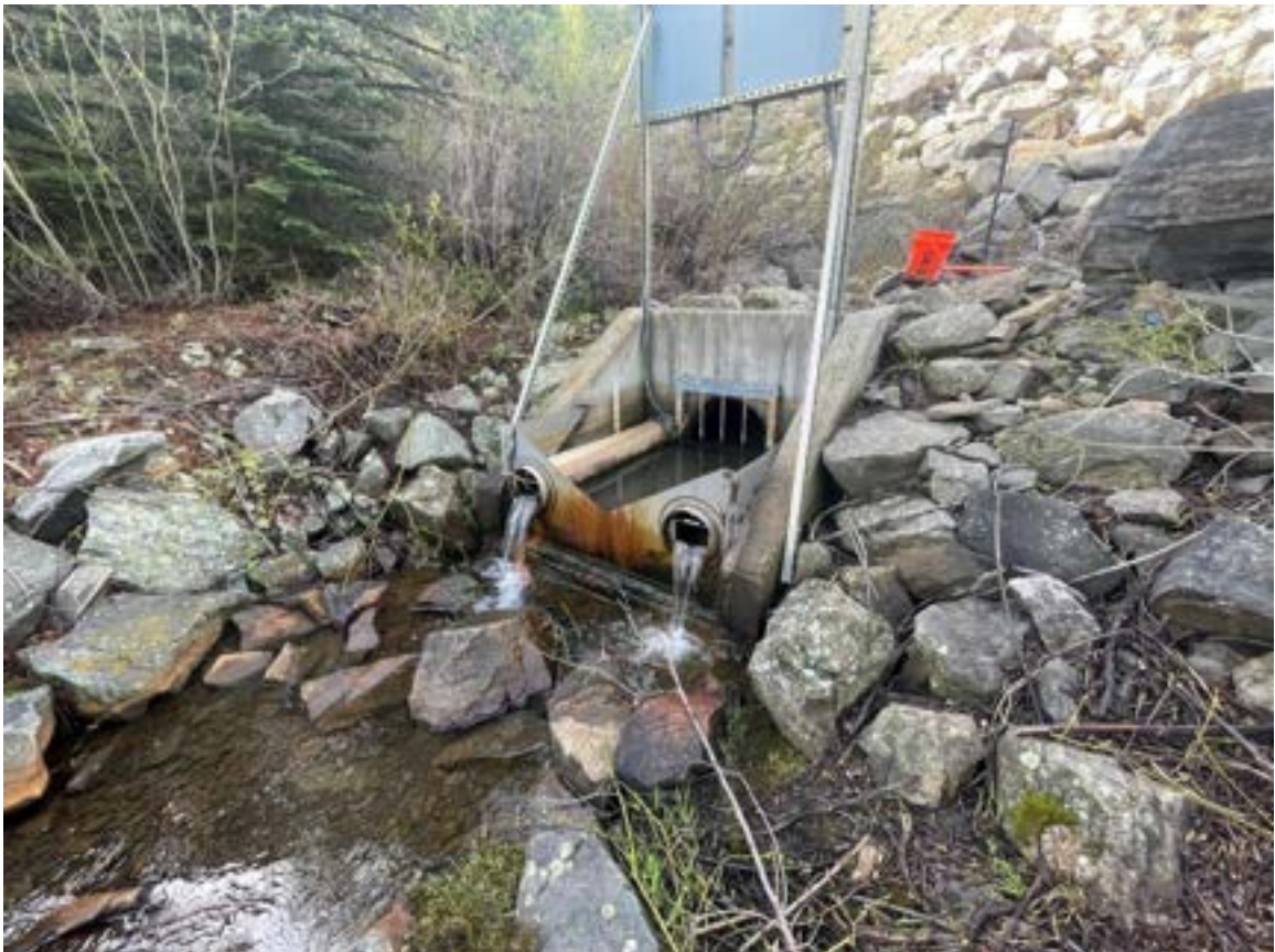
Photo 12: Outlet closed in preparation for conduit jetting / sliplining operations.
