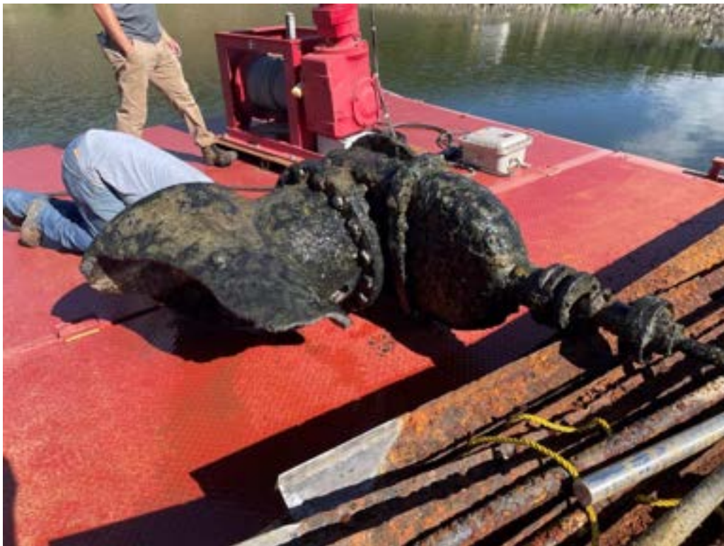
Photo 9: Left side of tee broken off and removed from structure.
