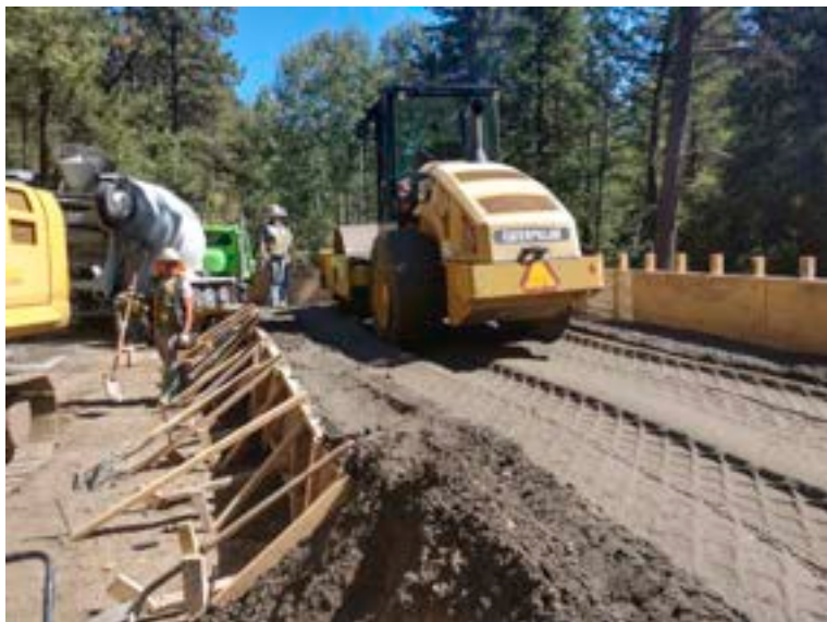
RCC test patch is laid and rolled to compact it
