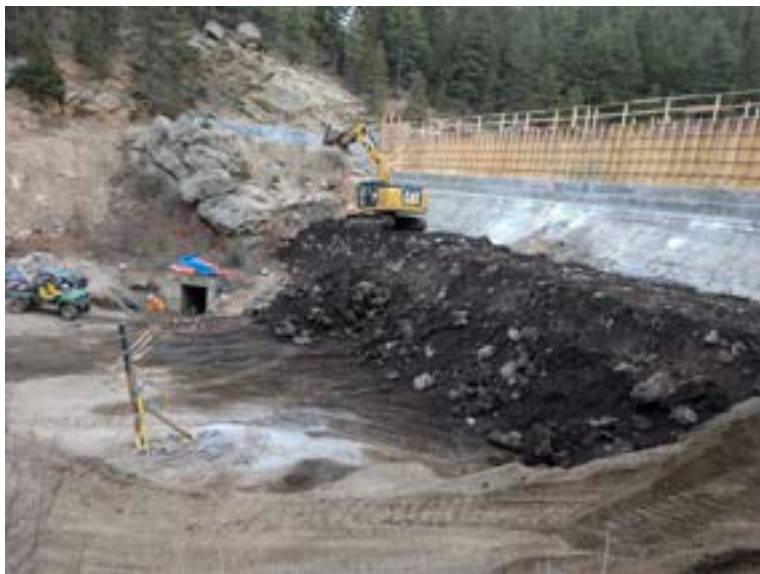
Bed is laid on downstream face for rip rap to be placed
