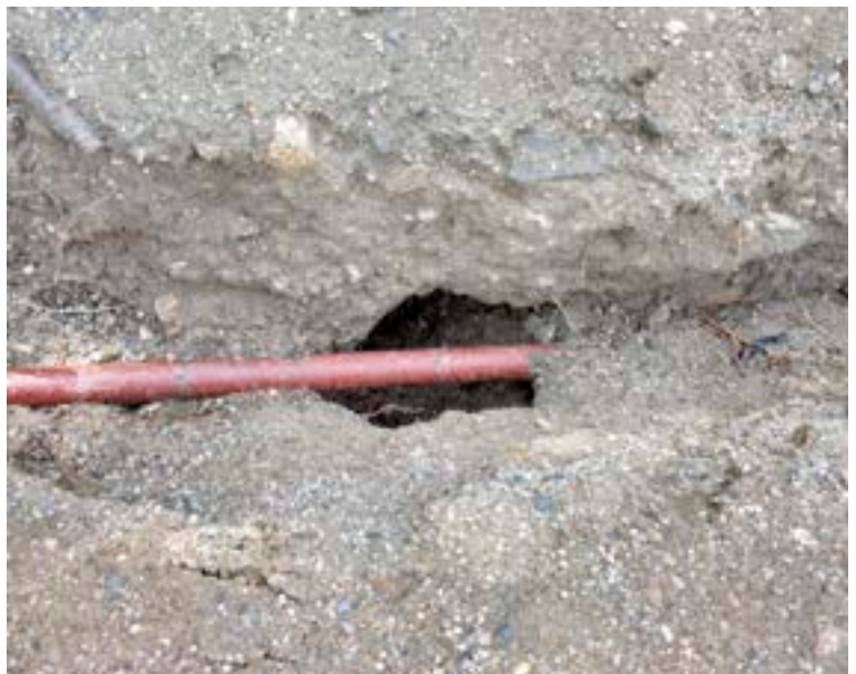
The xcel high pressure gas line running through the job site
