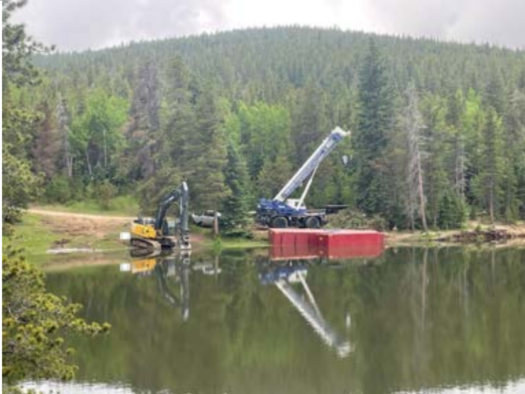
Photo 1: Barge setup and launch area. Crane staged for transferring barge segments to launch area.
