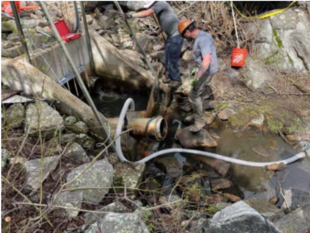
Photo 18: MDS deconstructing v-notch weir to drain outlet structure and facilitate conduit access.
