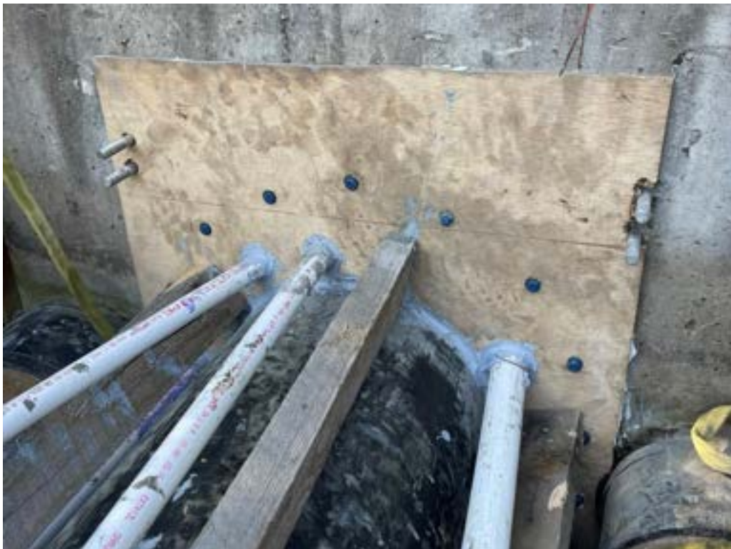
Photo 2: Downstream bulkhead anchoring and sealing.
