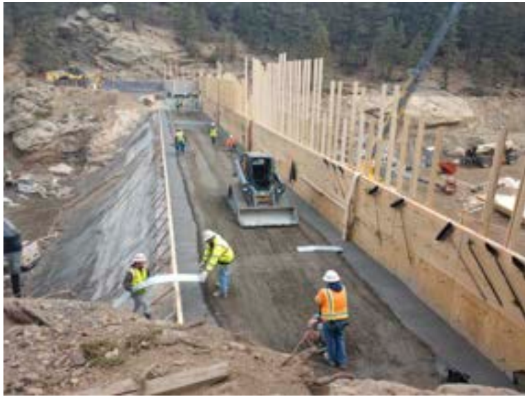
Last RCC lift getting finishing work
