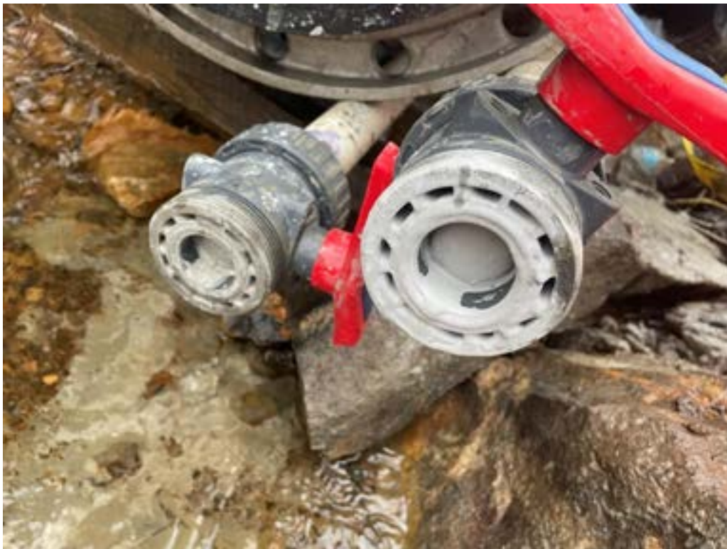
Photo 14: Grout return observed at 25% and 50% pipe lengths. Grout return also observed at 75% pipe length (not shown).
