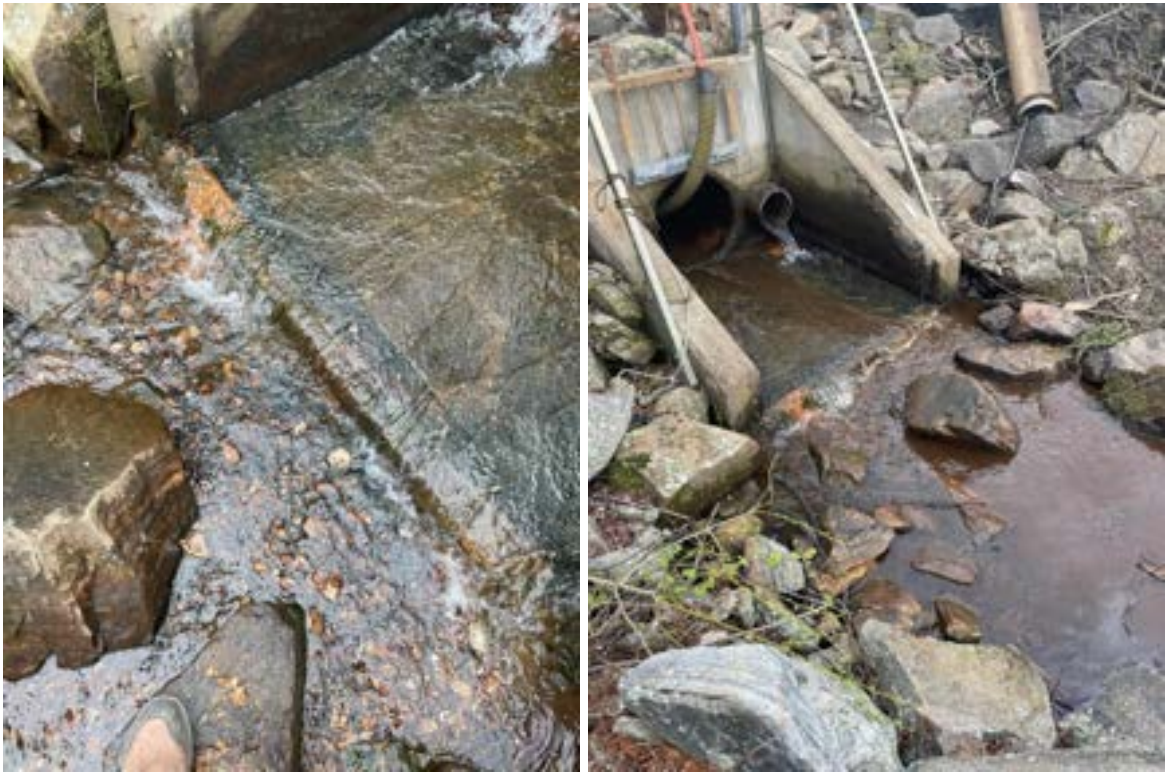
Photos 27 & 28: Lime scaling, corroded iron, and water with high suspended solids observed during jetting.
