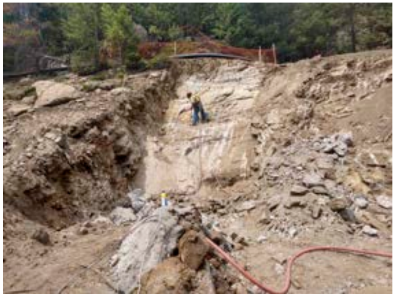
Find solid rock to interface with new dam
