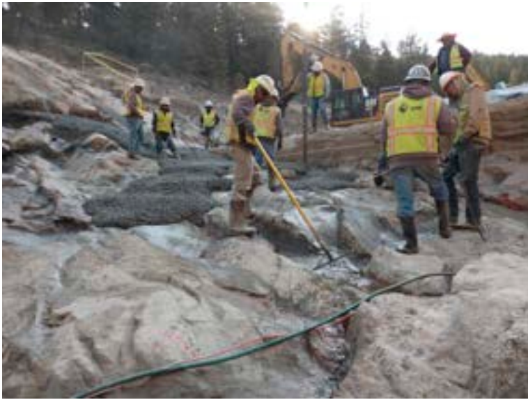
Dental Concrete being spread
