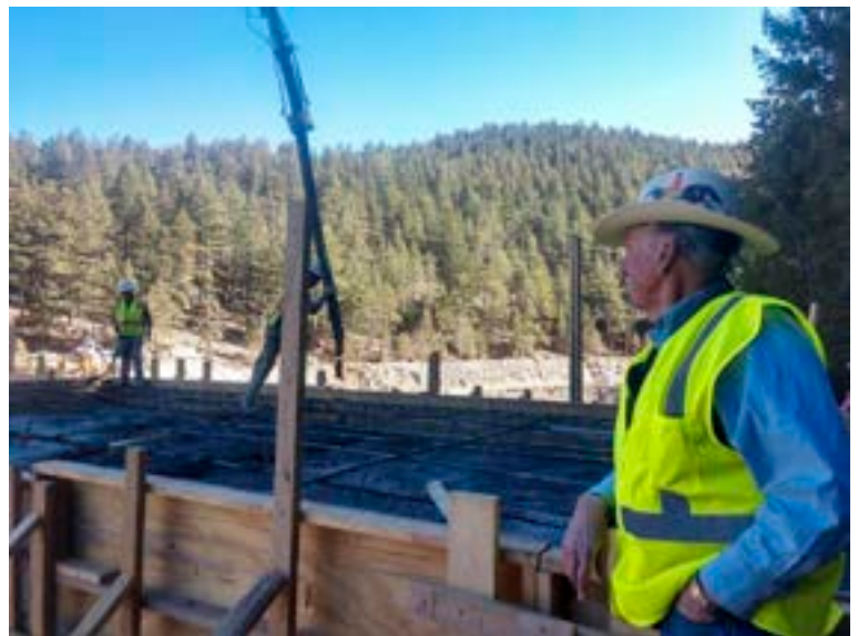
Dean Snyder watching conventional concrete final levels being placed
