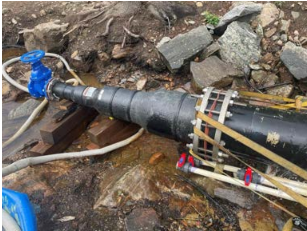
Photo 6: Temporary valve placed on downstream end of pipe.
