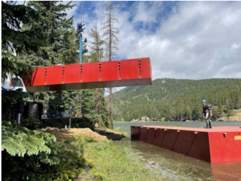
Photo 6: Placing Flexifloat barge segment at launch area.
