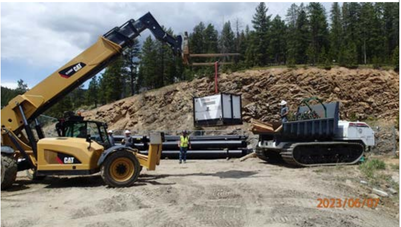
Photo 10: Loading crawler-carrier with HDPE fusion equipment.
