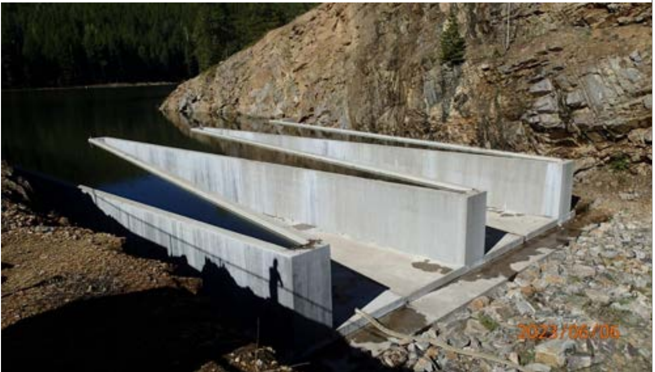
Photo 4: Reservoir level has been draw down below spillway crest elevation due to operation of the outlet works.
