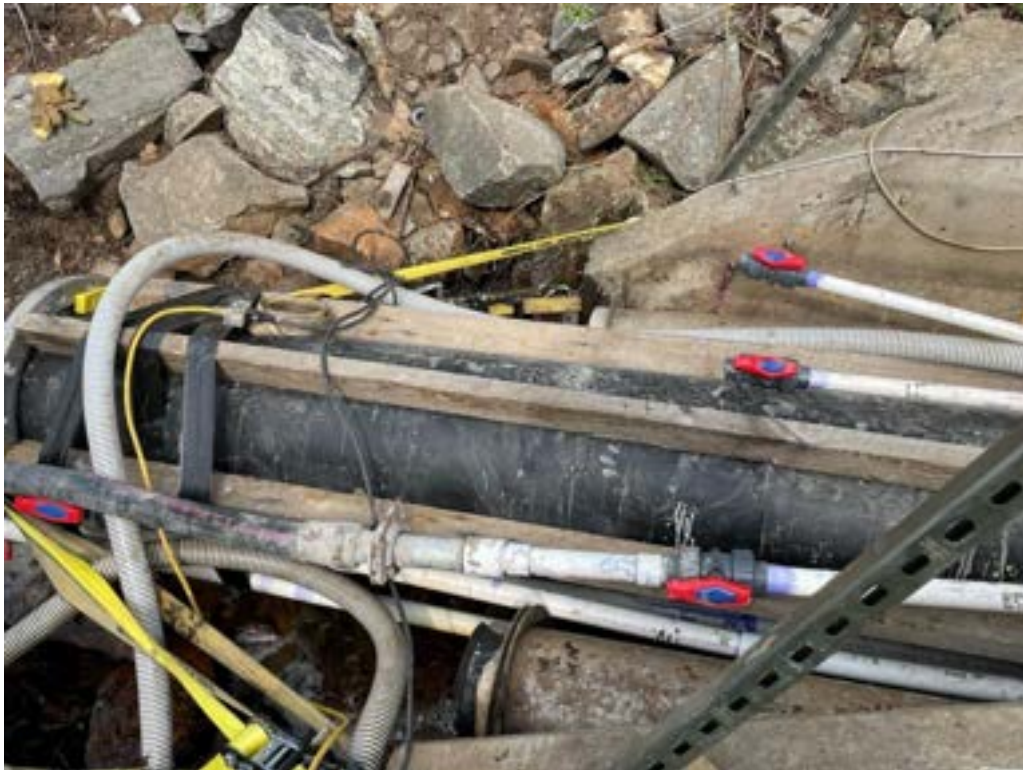
Photo 13: Grout hose connected to grout injection pipe.
