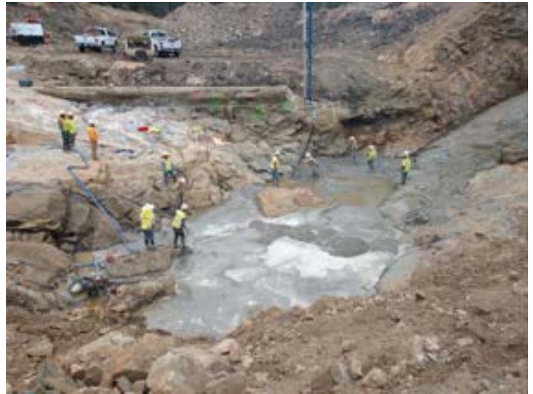
Starting 2nd pour of leveling floor for dam
