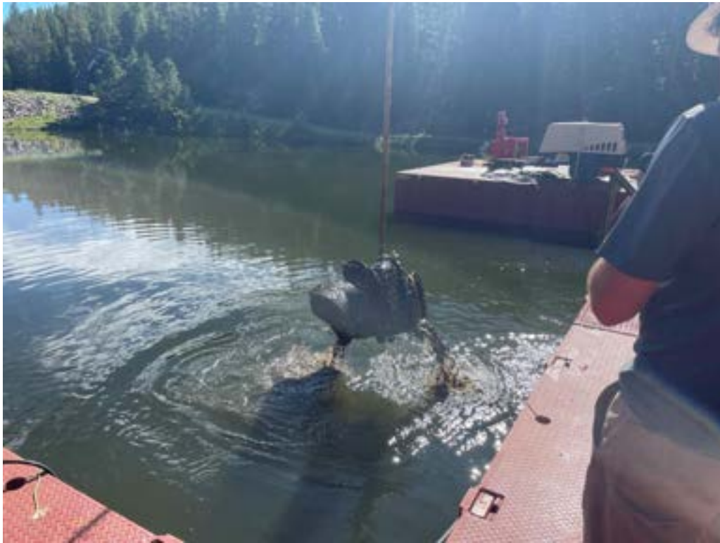
Photo 8: Left side of tee broken off and removed from structure.
