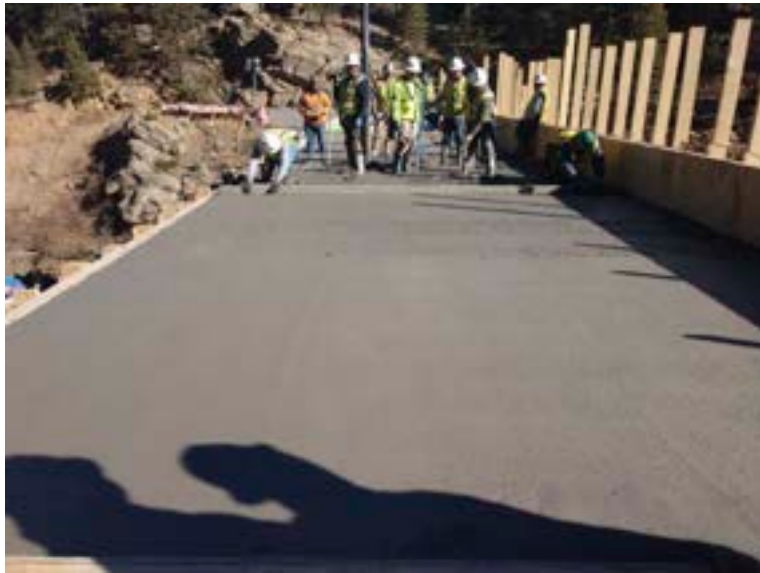
Concrete cap went on in layers
