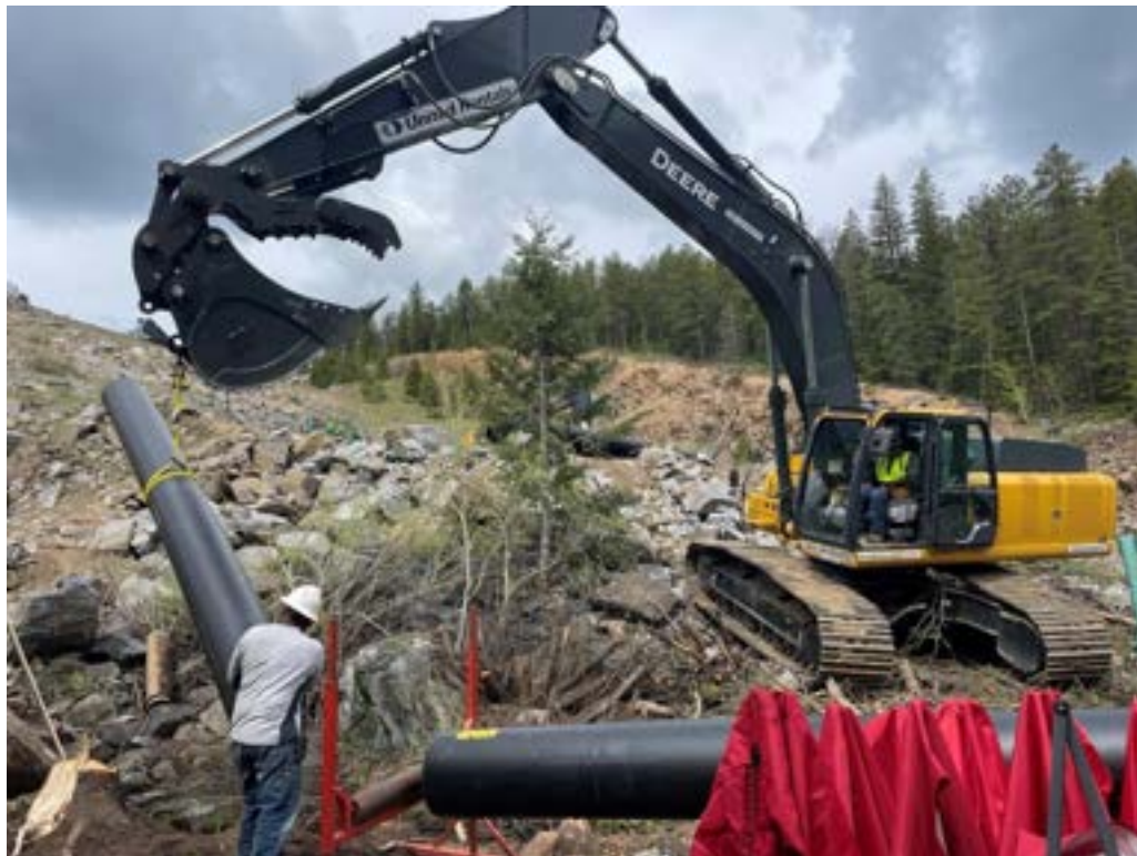
Photo 20: Excavator transferring HDPE section to prep for fusion.
