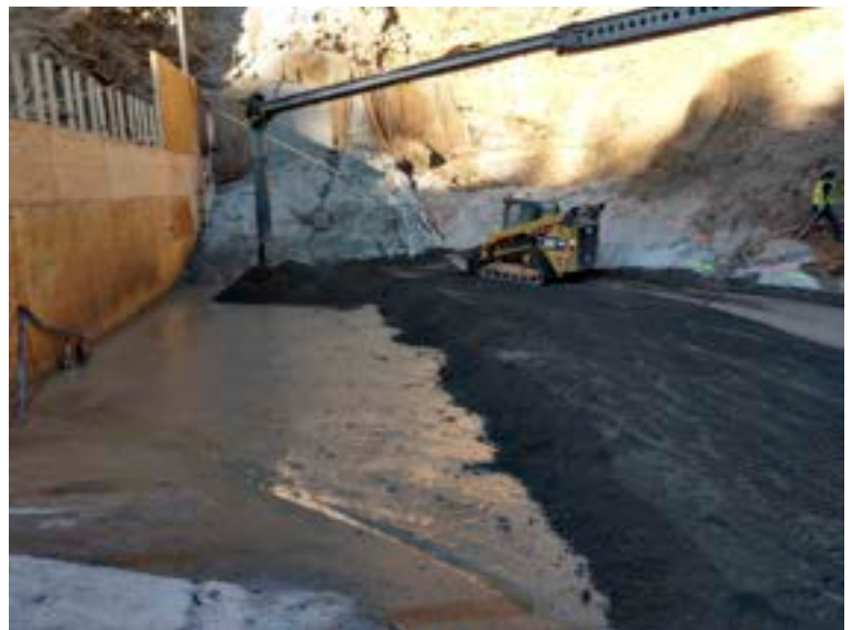
First placement of RCC underway
