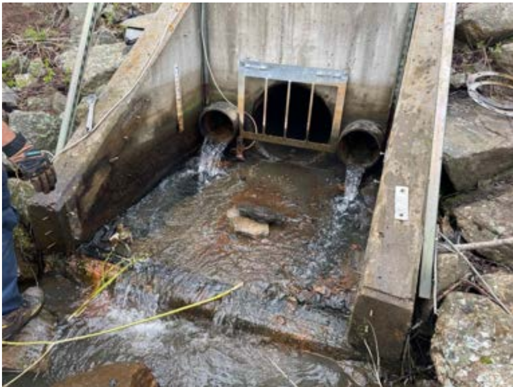
Photo 19: V-notch weir removed at outlet.
