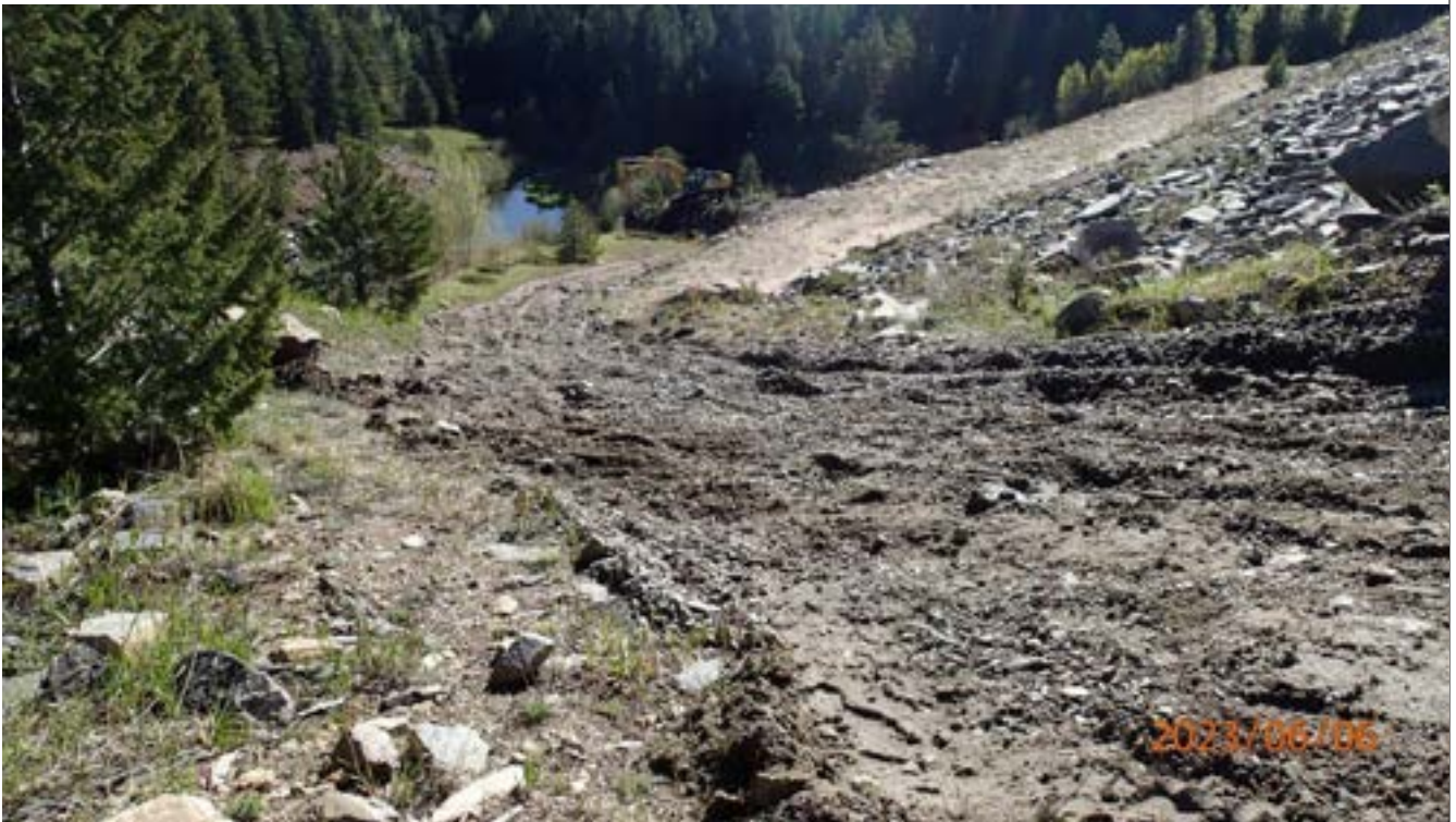
Photo 2: Fill material placed along access road to provide more even travel surface.
