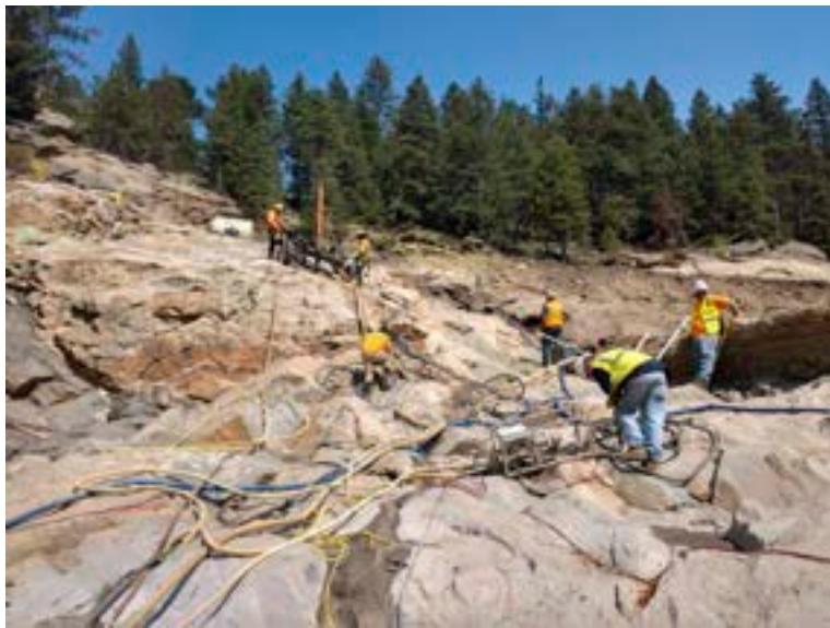
Drilling holes and injecting grout
