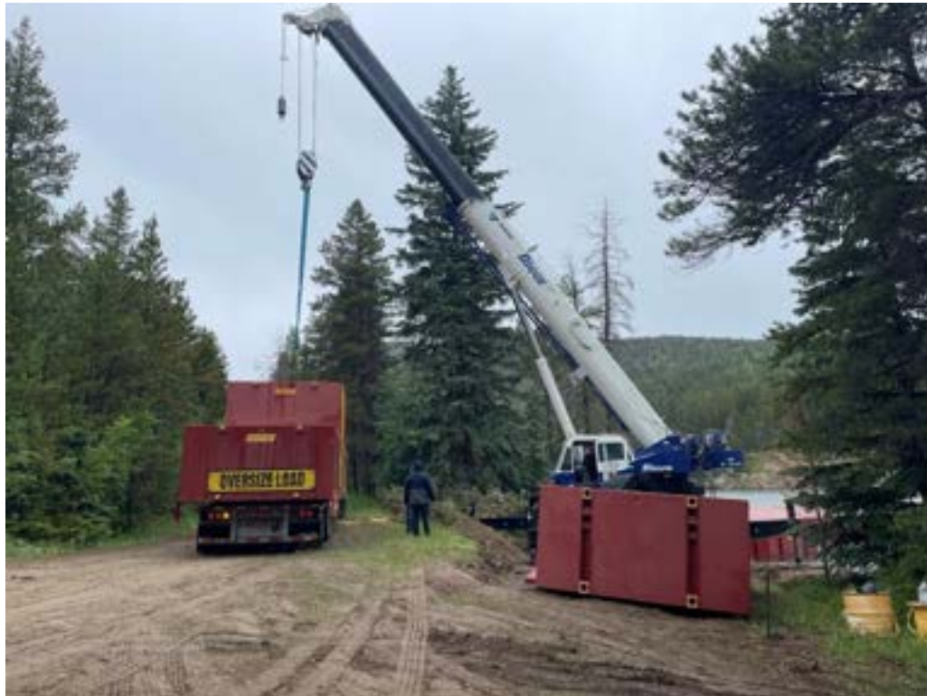
Photo 5: Crane picking Flexifloat barge segment from delivery truck.
