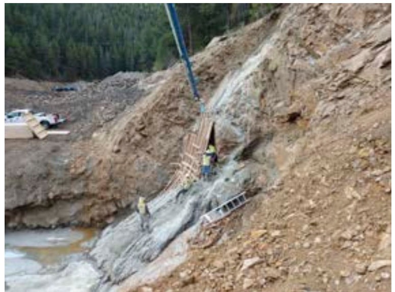
Dental concrete is laid all rock face for dam to seal
