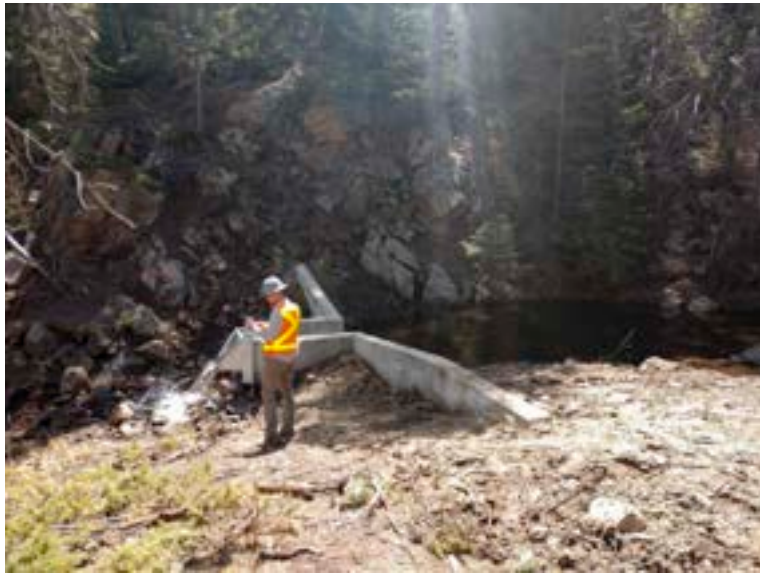
New Lower Beaver Brook inlet flume
