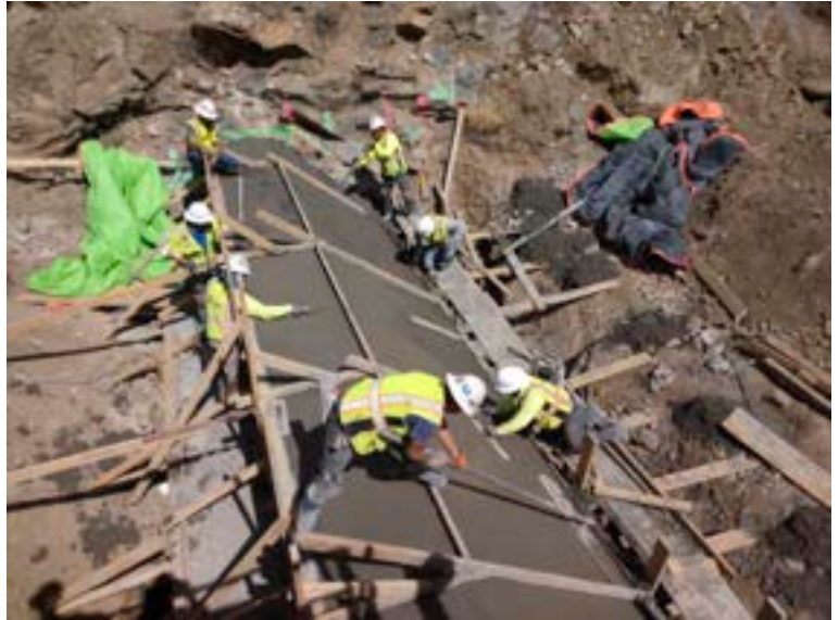
New spillway being finished
