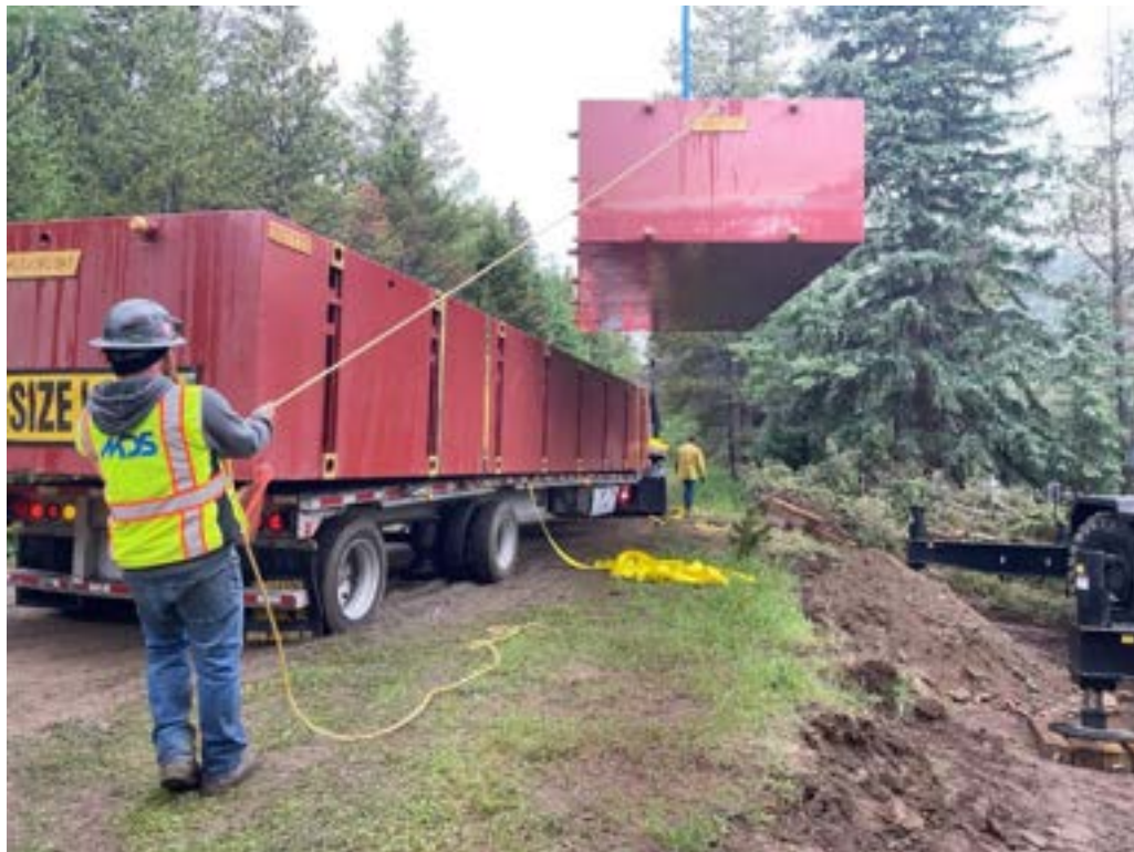
Photo 5: Transferring Flexifloat barge segment.
