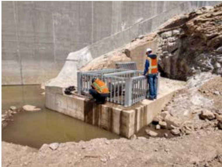
New trash rack over outlet valves
