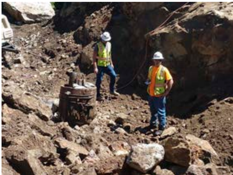
Original 1903 reservoir outlet, pipe with cement in a barrel
