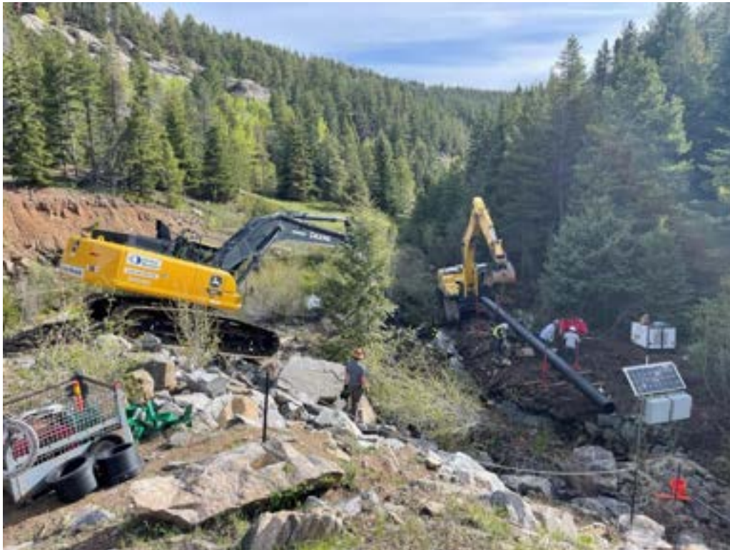
Photo 13: Site layout for HDPE fusion operations. Excavator on left is used to transport HDPE sections to the work area, excavator on right is used to pull HDPE string back as sections are fused.
