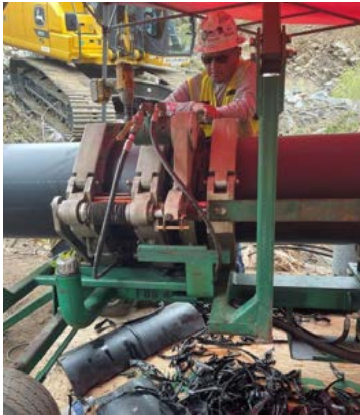
Photo 21: Pipe surfacing and welding performed using McElroy 18" HDPE Fusion Machine.
