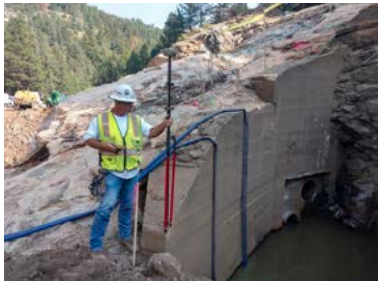
Establishing position of concrete headwall that ties into new dam
