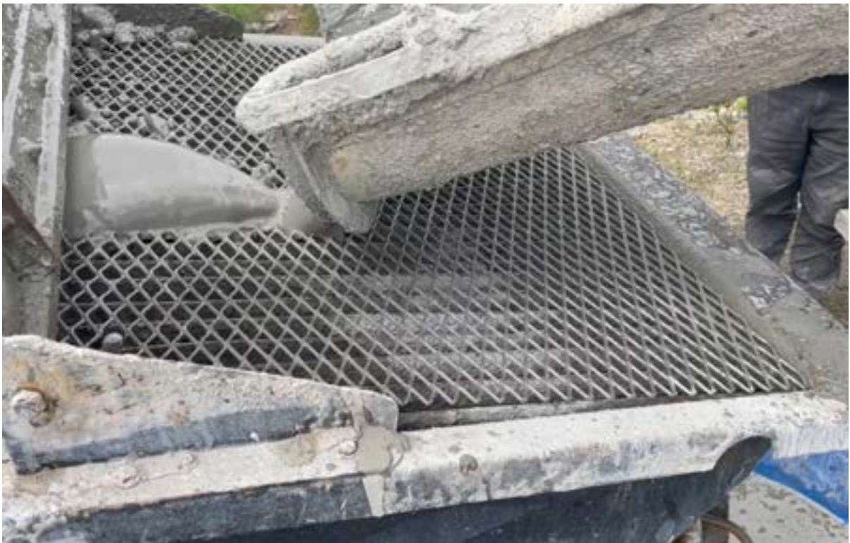
Photo 12: Grout pour into concrete hopper. Some doughballs observed in mix, as shown on strainer.
