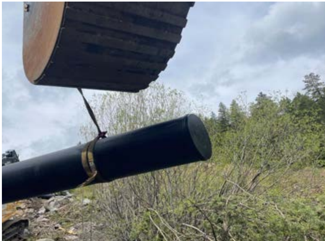
Photo 23: Downstream end has temporary cap to allow pressure testing upon completion of welding.
