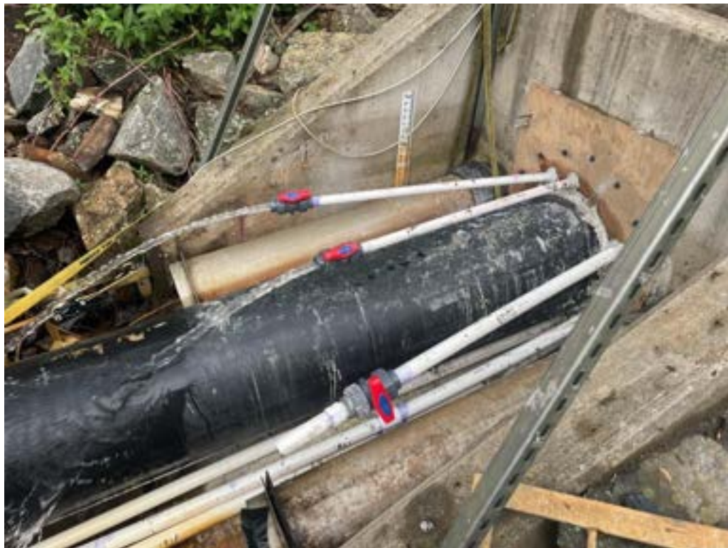
Photo 5: Water free flowing through grout vent pipes (approx 95% of pipe length) indicating grout is not placed up to the crown of the pipe at the full length.
