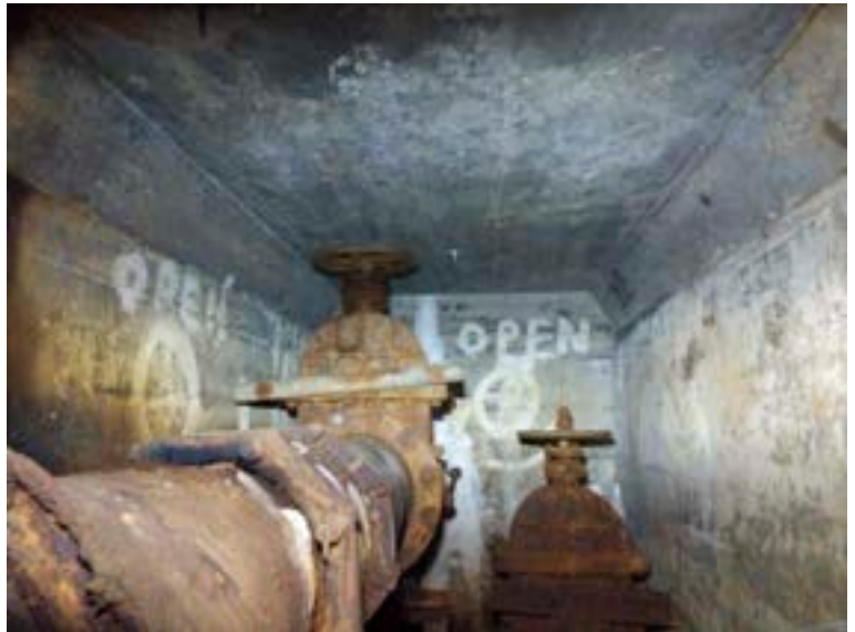
Original outlet and WTP plant pipe in man tunnel
