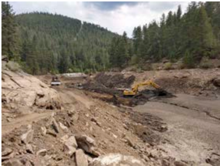
Working to dry out sediment
