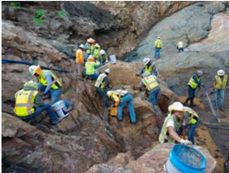
Many Zac workers cleaning and grouting by hand
