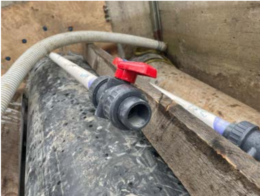
Photo 15: Partial grout return observed at 100% vent pipe lengths, as indicated by dried grout collected in pipe valve.
