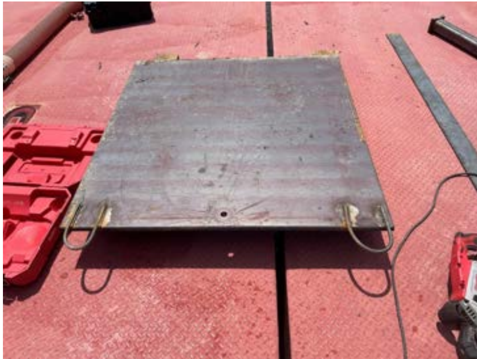
Photo 1: One of two 4'x4' steel plates placed against downstream headwall to brace hydraulic ram and push of tee at bell and spigot.
