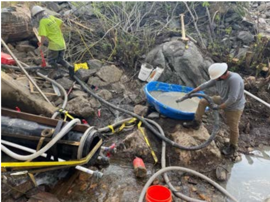
Photo 16: Contractor performing final line cleanout following completion of grouting.
