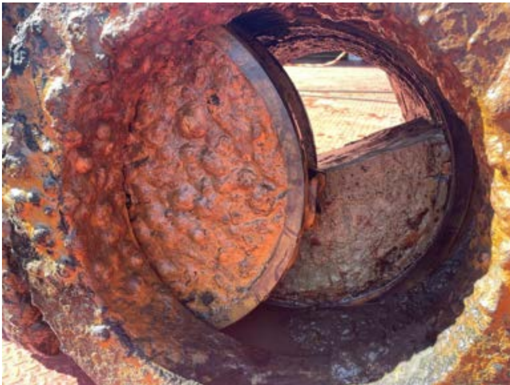
Photo 11: Grout placement within tee (approximately 50% full).
