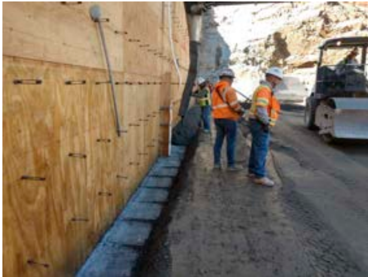
Conventional concrete being pumped into place while RCC rolled
