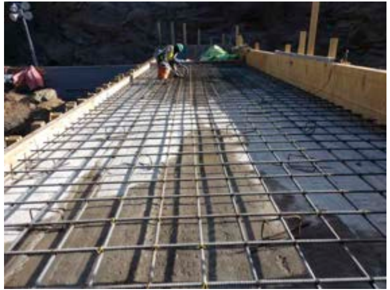
Rebar for conventional concrete cap
