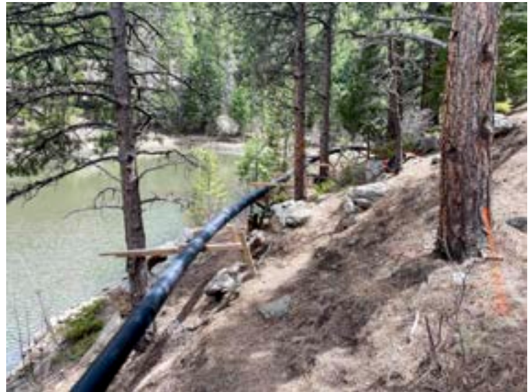
Temporary feed for WTP so reservoir can be drained
