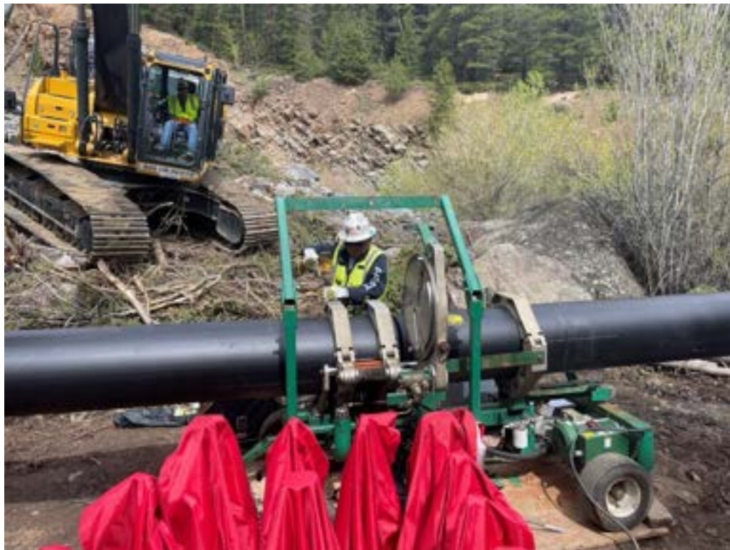
Photo 21: HDPE sections in place for surfacing/fusion
