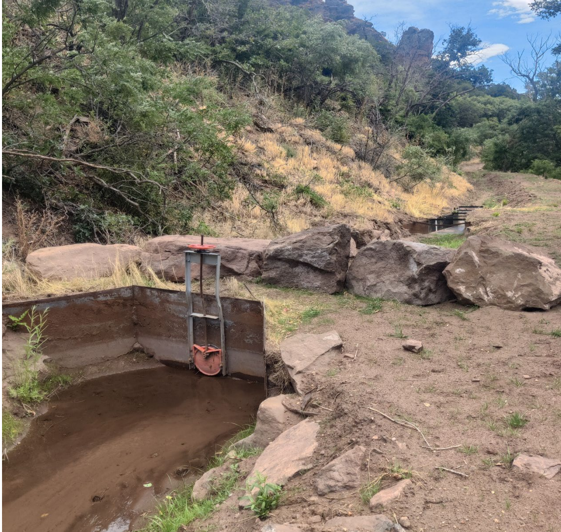
Diversion (background) and headgate with boulders to mitigate flood surges
