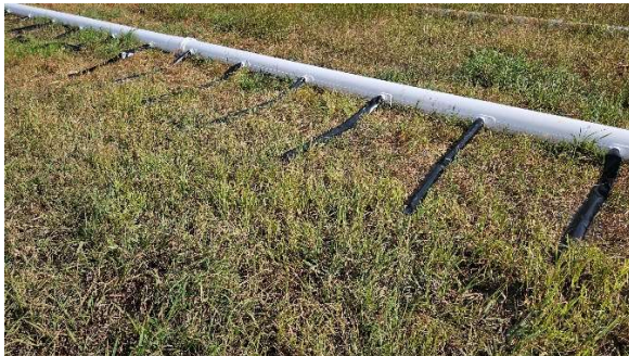
Figure 8 Anti-erosion sock attachment (left), 2" lay-flat slitted pipe extensions (right)
