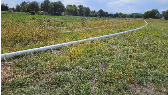
Figure 7 Hayfield Installation of pre-assembled 8" pipe
