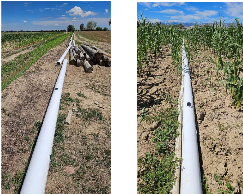
Figure 3 Pre-assembled pipe ready for placement (right), automated gated pipe replacing existing lay-flat (left)
