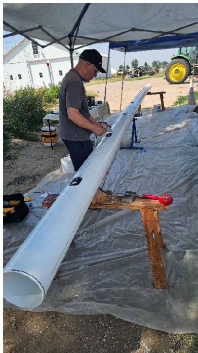
Figure 2 Pipe assembly process (left), thirty completed pre-assembled pipes (right)
