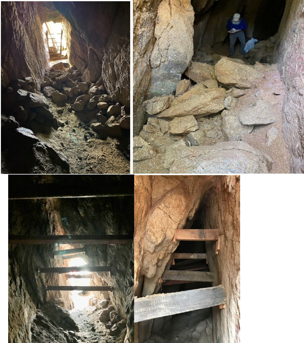
Figure 5: Temporary Stabilization of Flaking Rock 2023 – 2024
