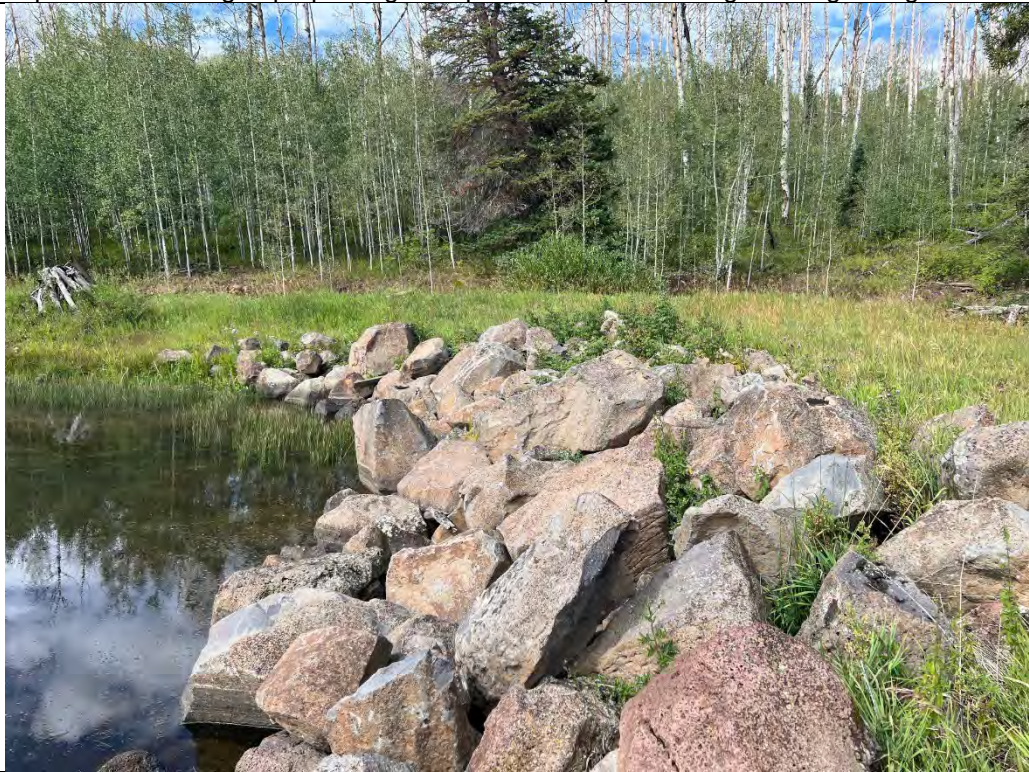
Photo 4. View of the upstream slope riprap looking left from the outlet works catwalk.
