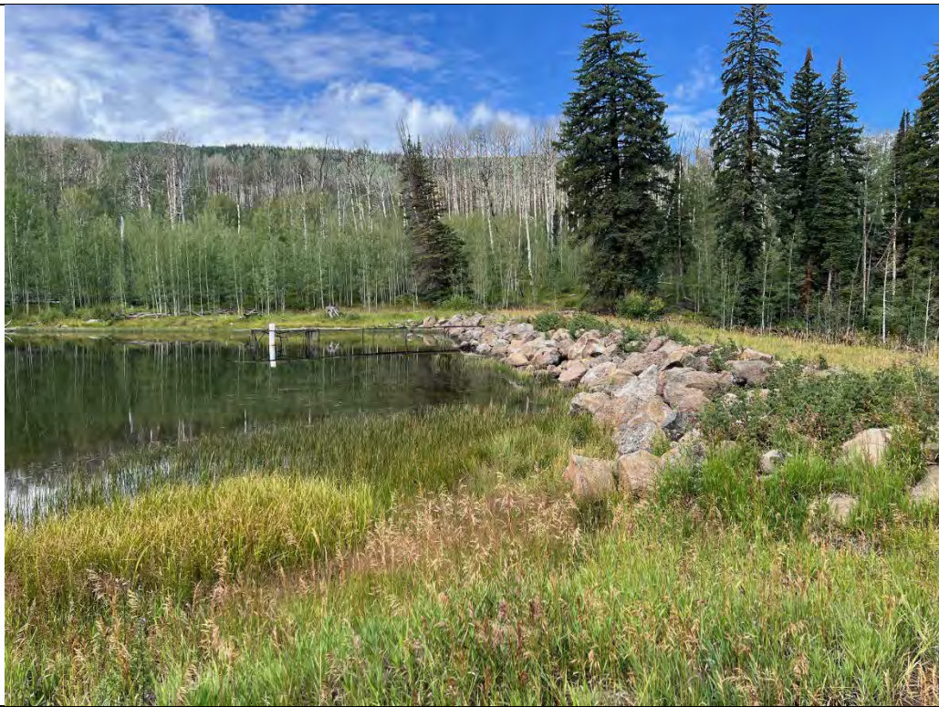
Photo 1. View of the upstream slope looking left from the right abutment. Note the large riprap and vegetation growing in the riprap.
