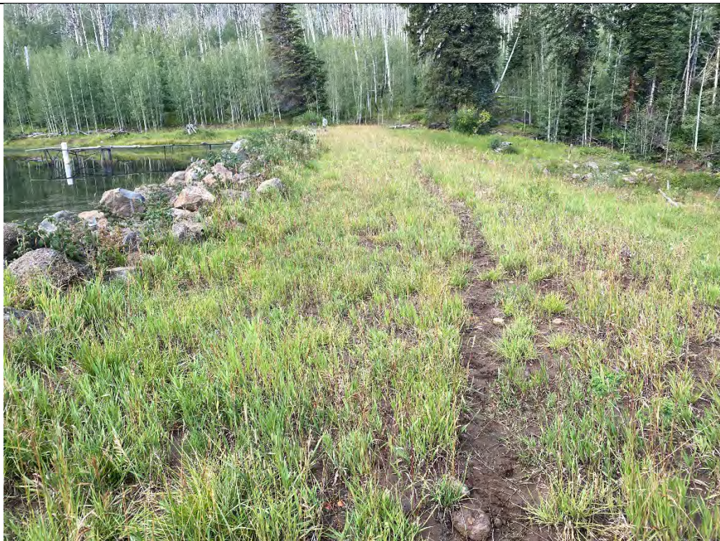
Photo 5. View of the dam crest looking left from the right abutment. Note the animal trail along the crest.
