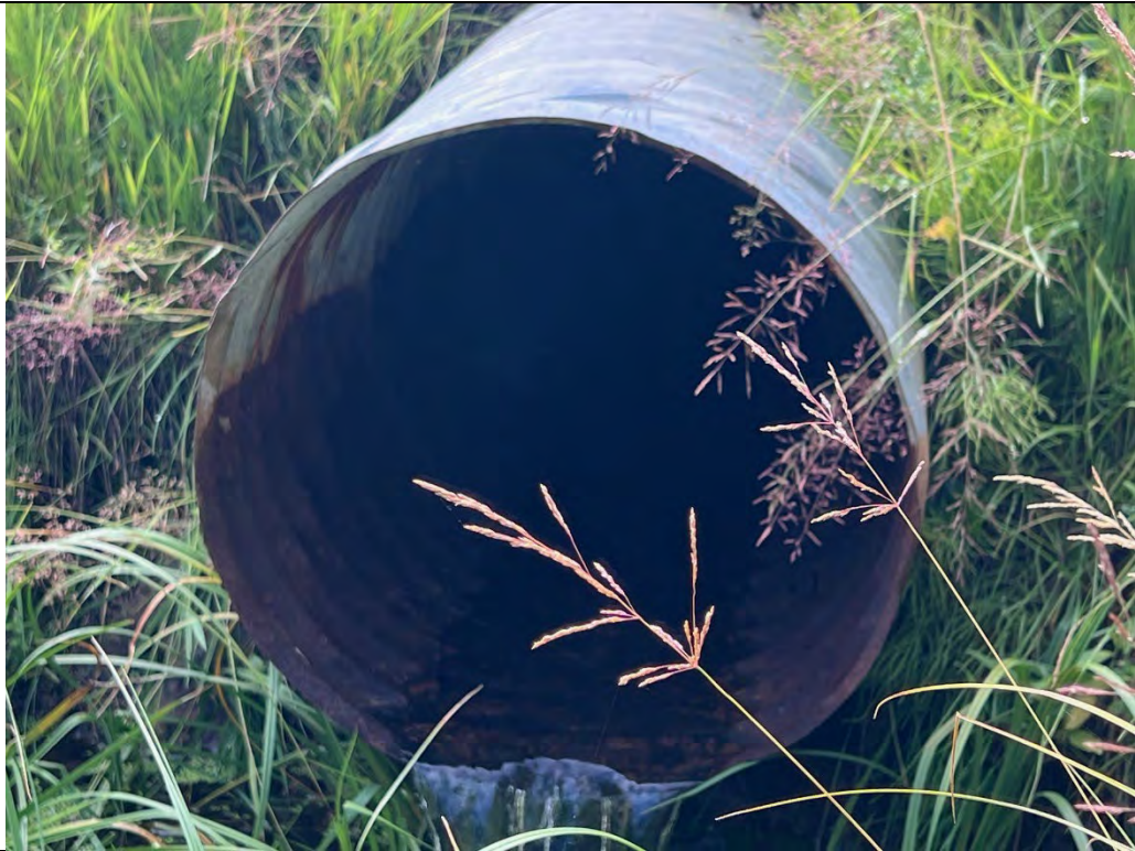
Photo 19. Close up view of the 24-inch CMP Outlet Pipe. The invert of the pipe appears to be eroding.
