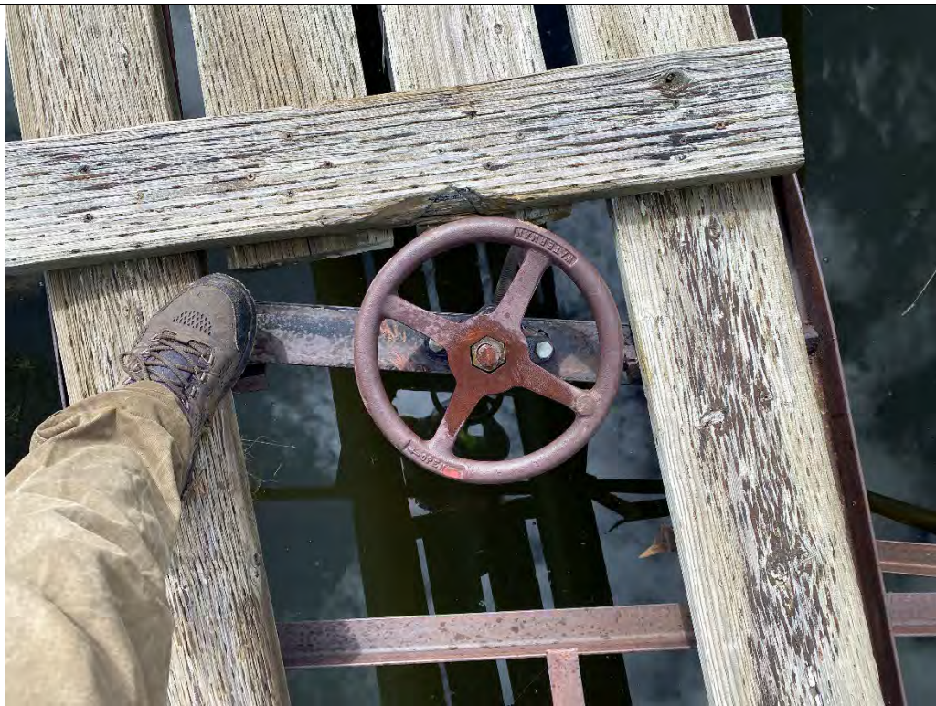
Photo 15. Close up of the existing outlet works gate operator. Note that gate is fully exposed in reservoir and appears to be slightly bent and showing signs of corrosion.
