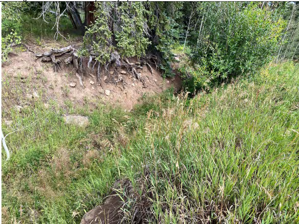
Photo 10. View of the primary spillway bank erosion. This erosion is downstream of the dam but should potentially be armored with riprap to reduce erosion over time.
