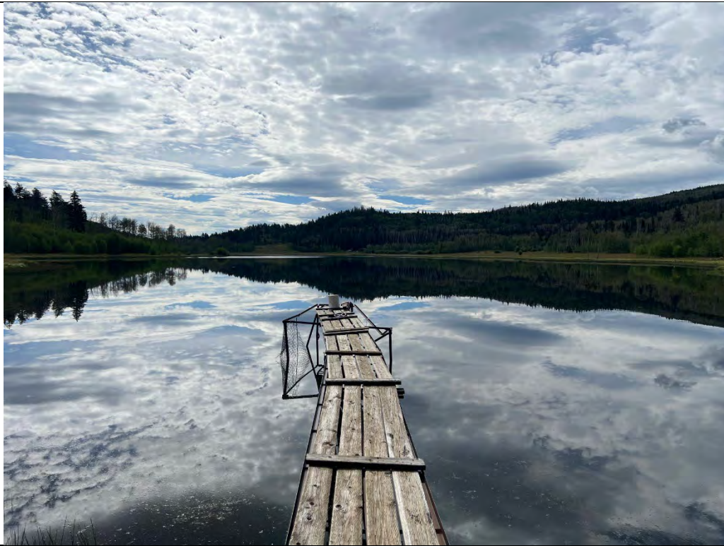
Photo 13. View of the outlet control gate and siphon system access walkway. Note that walkway should be repaired and stabilized for a safe access to operate the gate.
