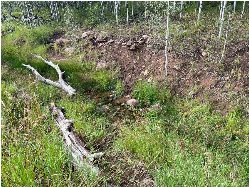
Photo 7. View of the apparent control section of the primary spillway located near the left abutment. Note the woody debris and vegetation in the spillway.
