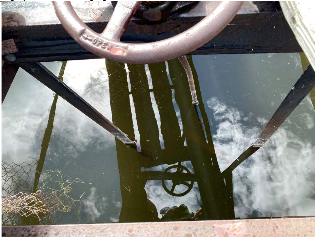
Photo 16. View looking down into the reservoir at the outlet gate. Notice the bend in the gate frame, indicating the gate is likely bent as well.
