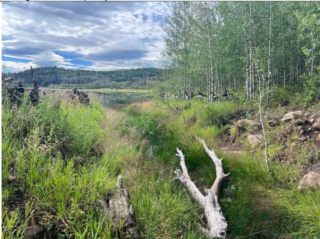
Photo 8. View looking upstream at the approach channel of the primary spillway. Again note the vegetation and debris in the spillway.
