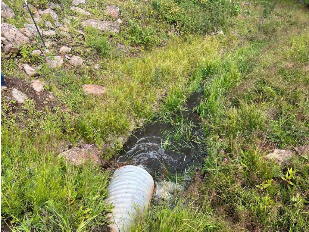
Photo 17. View of the 24-inch CMP outlet discharge conduit.
