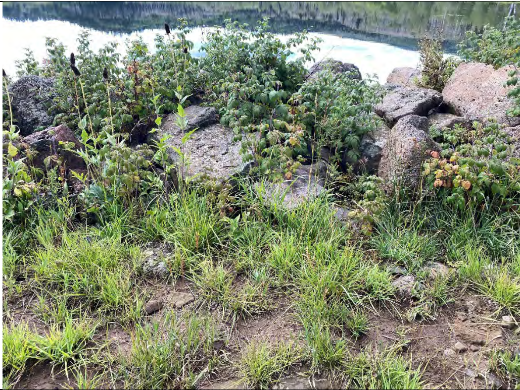
Photo 3. Close up view of the large riprap along the upstream slope with vegetation growing between the riprap.
