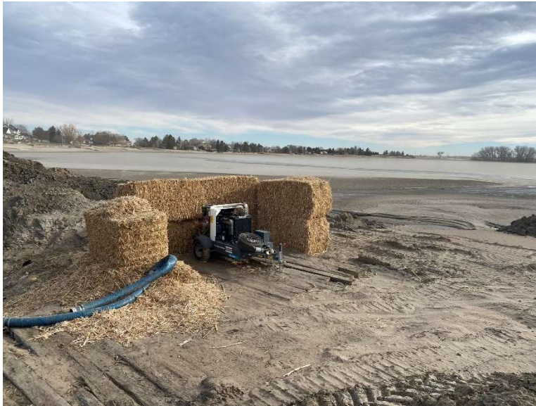
Pump setup for dewatering – 12/13/23
