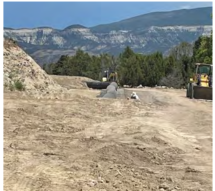
Standing on buried section of 36" HDPE
