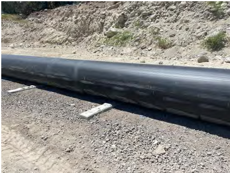
Exposed section of 36" HDPE
