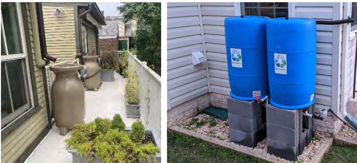
Figure 1. Rain barrels harvesting roof runoff at residential households.
