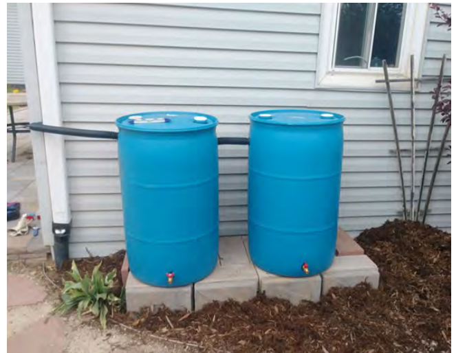
Photo 1. Two 55-gallon rain barrels at a residential household.
