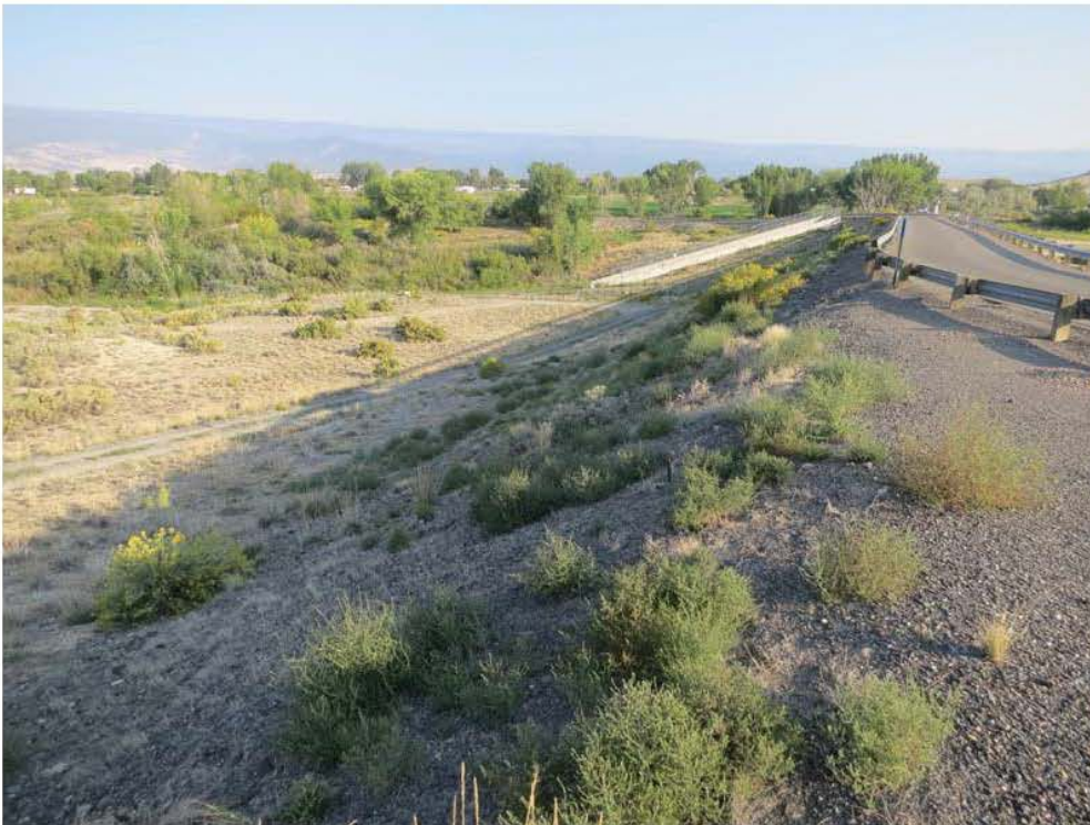
Photo 2 - Downstream face, looking right from the left abutment; 9/9/2021.
