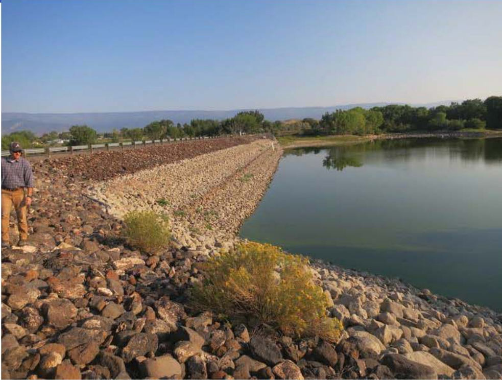
Photo 1 - Upstream face, looking right from the left abutment; 9/9/2021.
