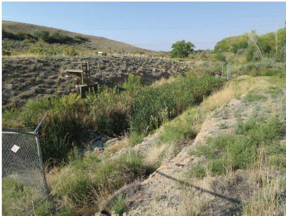
Photo 14 - Alfalfa Run (outlet channel) downstream of the dam; note thick vegetation between stilling box and flume; 9/9/2021.
