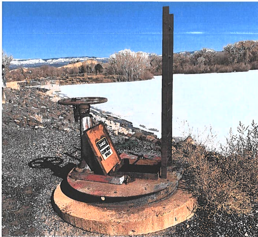
Photo of the access to the gate valves in the outlet works.
