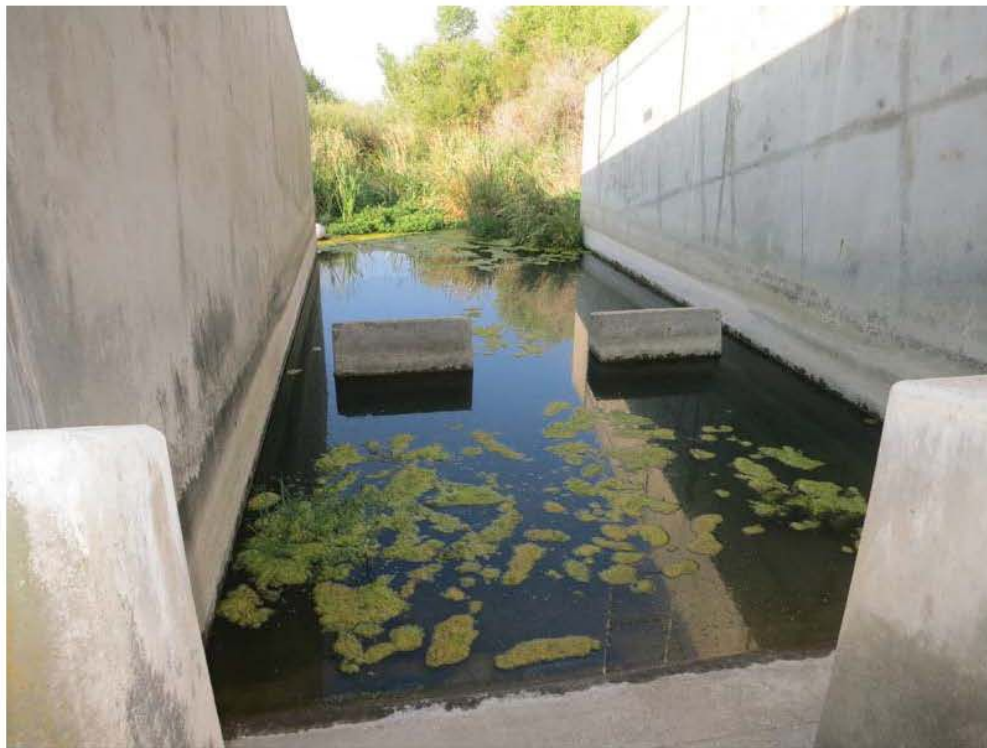
Photo 9 - Spillway stilling basin looking downstream. Note thick vegetation in the channel; 9/9/2021.
