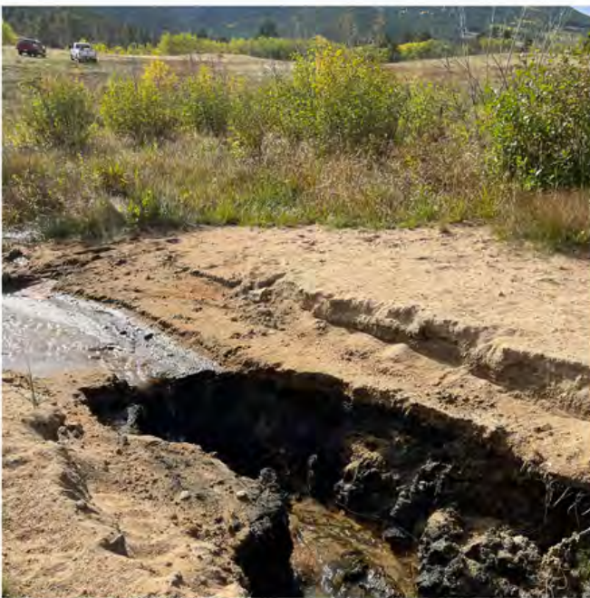
Back side of the headcut that needed repairs, second wash out of the earthen berm (September 2022).
