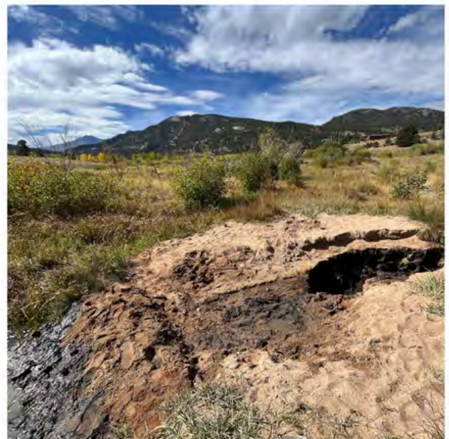
Repaired headcut using fill and handwork (September 2022).
