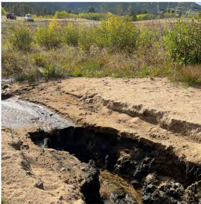
Back side of the headcut that needed repairs (September 2022).
