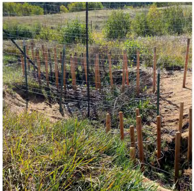
Repaired headcut using willow weave simulated beaver structures, sod mats and native vegetation (Sept 2023).
