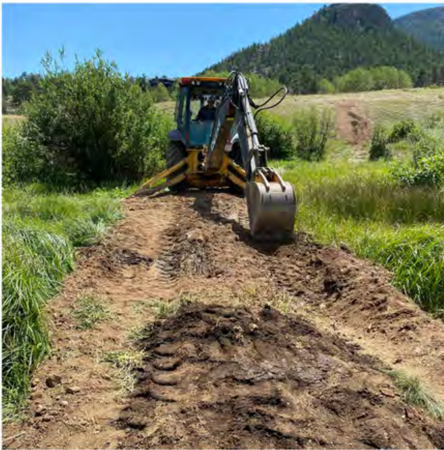
Excavator helping to build berm (August 2022).
