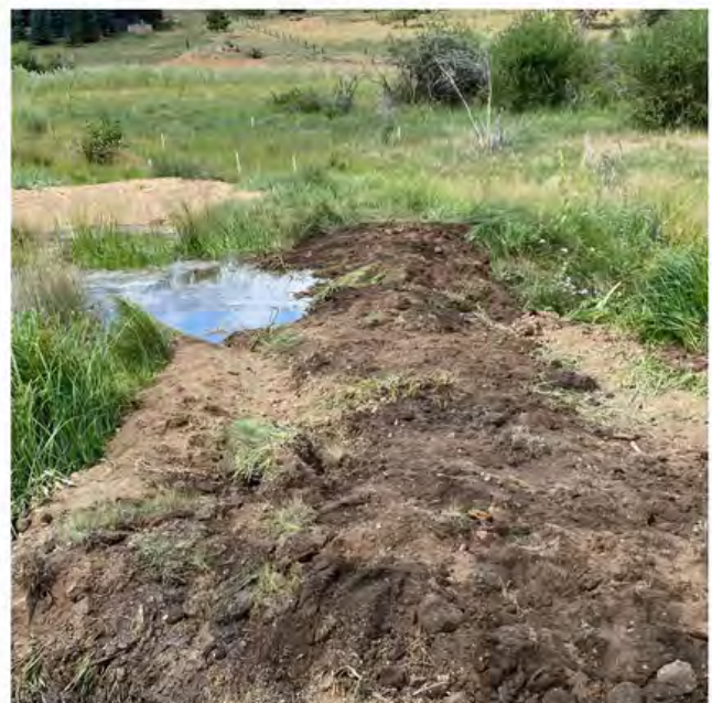
Same location facing the other direction showing berm and headcut filled in (August 2022).
