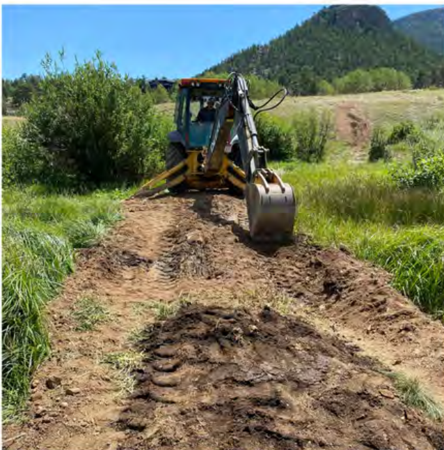
Excavator helping to build berm (August 2022).
