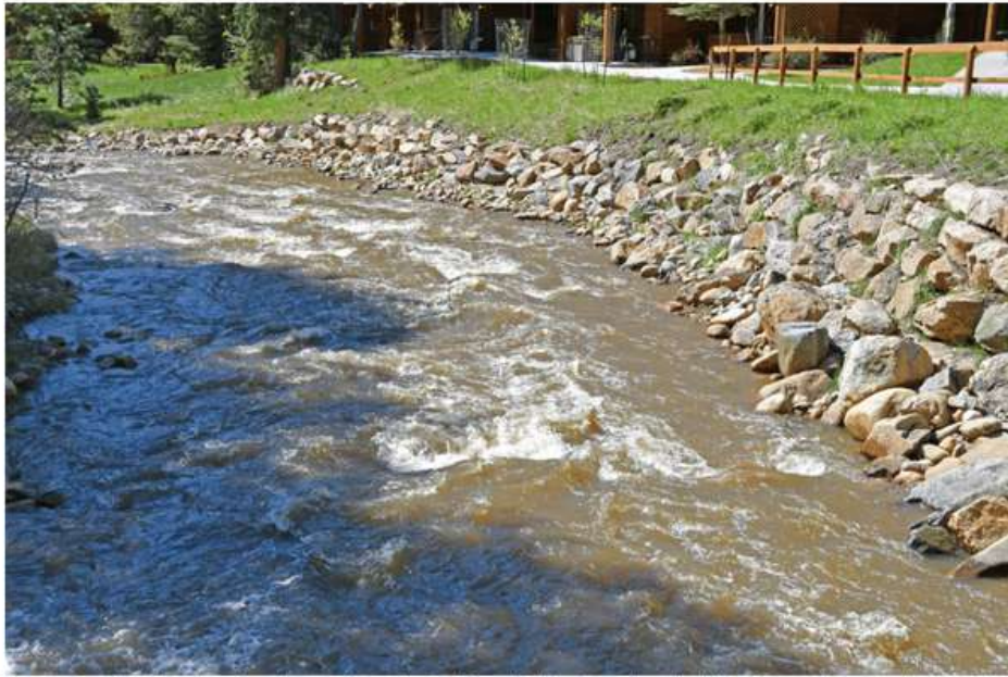
Photo 5. Fall River at Bugle Point showing riprap along banks (installed before the rehabilitation project) and poor willow stake survival.
