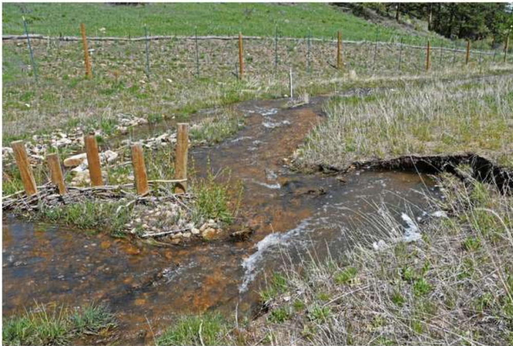
Photo 18. Fish Creek at Brook Drive - lowest BDA with largest extent of flanking (note this is a secondary check structure serving as grade control for the primary check located just upstream (and out of the photo) – pool habitat is not the goal of this structure.)
