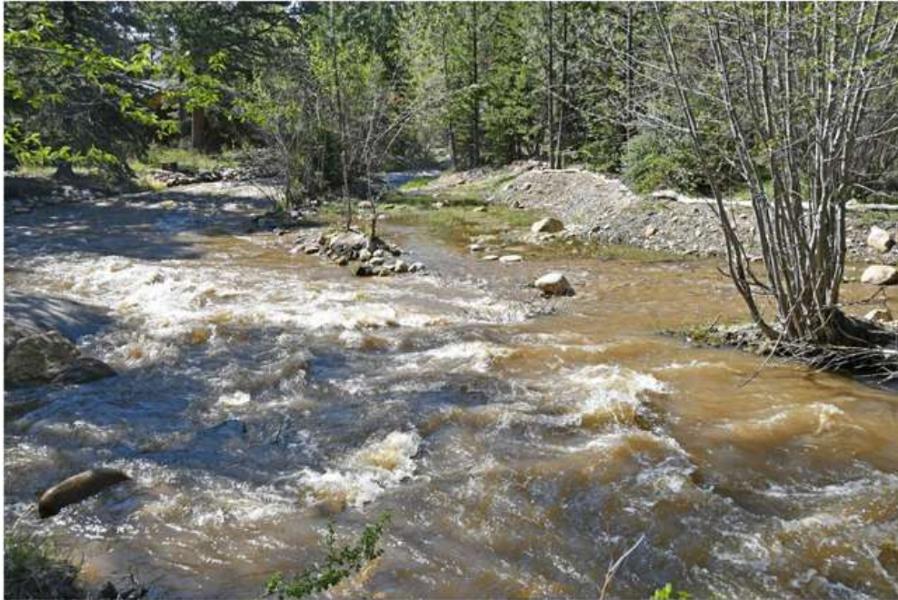
Photo 7. Fall River at Bugle Point - 1.5-year flow bench (right side) with some flow across it.
