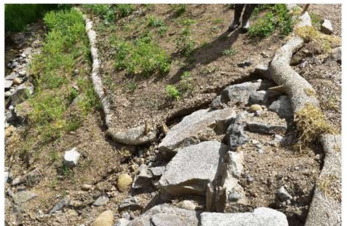
Rock-n Roll: Note initiation of rill erosion.
