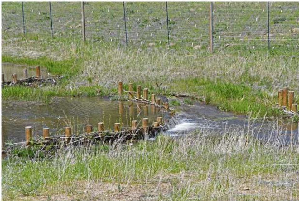
Photo 17. Fish Creek at Brook Drive - middle BDA functioning as expected (primary check structure in center of photo).
