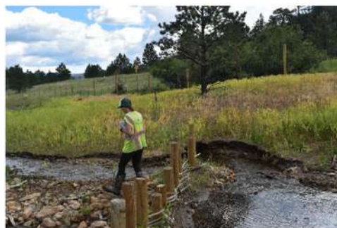
Middle Fish R4: Showing flanking around Beaver dam analogues and bank erosion and Vegetation Regrowth
