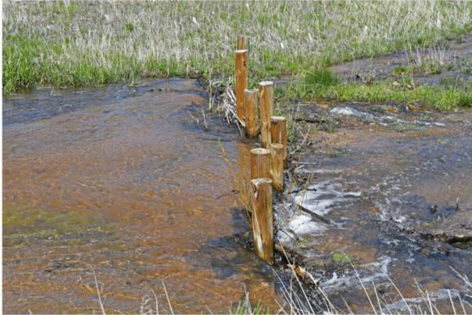
Photo 16. Fish Creek at Brook Drive - upper BDA showing sediment buildup and minor flanking.
