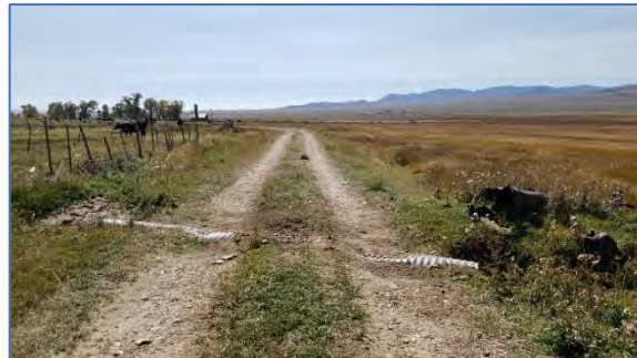
Dilapidated culvert.
