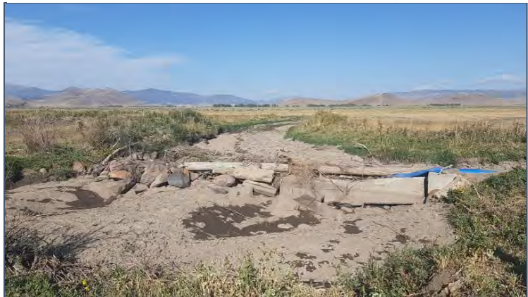
Water diversion on the Hill SLB property on Saguache Creek.
