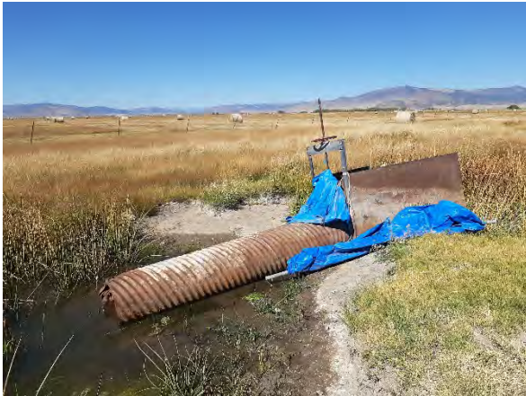
Water control structure with potential for rehabilitation and restoration.
