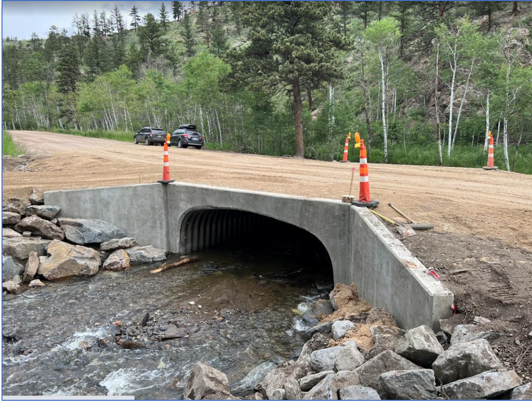
Photo 30: Post-Construction - Sheep Creek Corrugated Plate Arch Structure – substantially complete (looking North) June 2023
