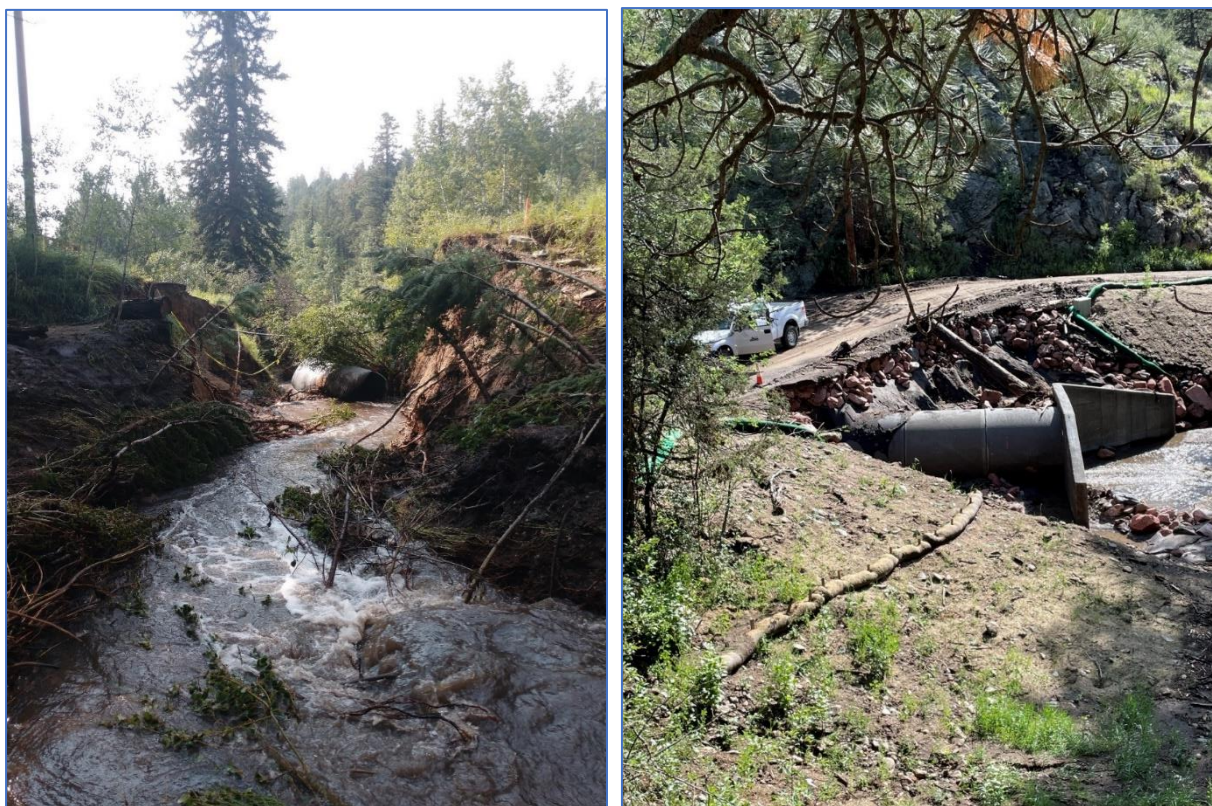
Photo 16 (Left): Upper Streamside Drive Culvert (The metal pipe clogged with debris which resulted in severe erosion), 2021. Photo 17 (Right): Upper Streamside Drive – July 2022 Flooding: An 84" reinforced concrete pipe (RCP) was installed after the 2021 flood; however, the culvert was overtopped during multiple storm events in 2022. The D50 24" riprap (ungROUTED) was replaced with D50 12" matrix (partially-grouted) riprap in 2022 to improve resiliency.
