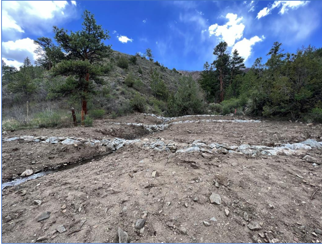
Photo 26: Post-Construction – Looking South at the rock check dams installed at Bears Gulch (2023)
