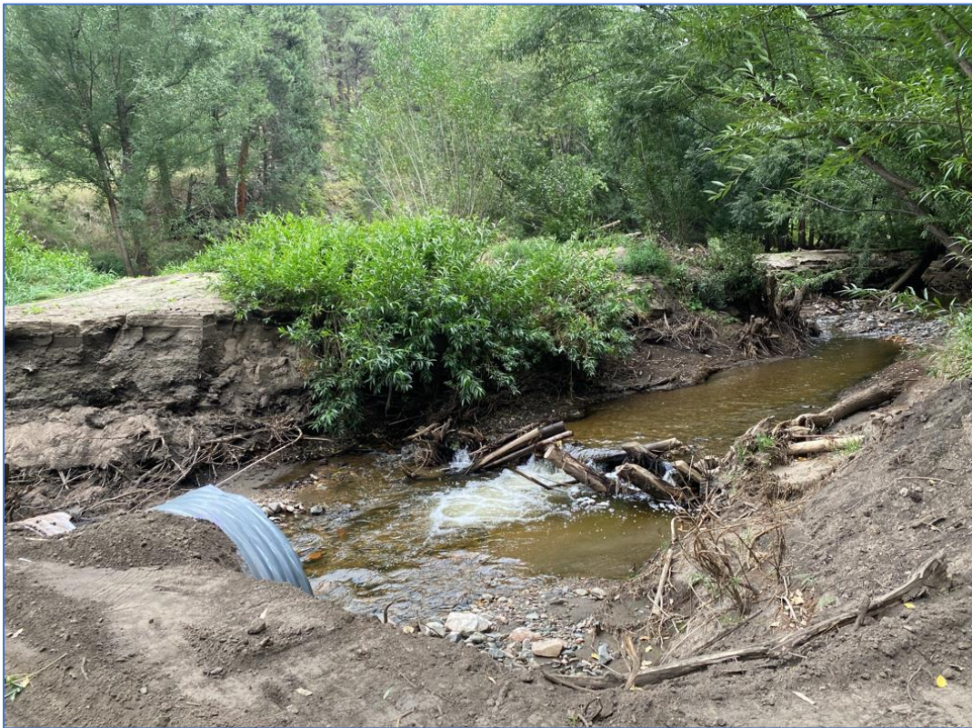
Photo 33: Pre-Construction – Debris deposit on the upstream side of the Deerpath culvert (2022)
