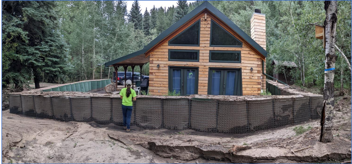
Photo 19: Post-flood event at 719 Streamside - Flood barrier bags surround the home and were fully activated by the flood
