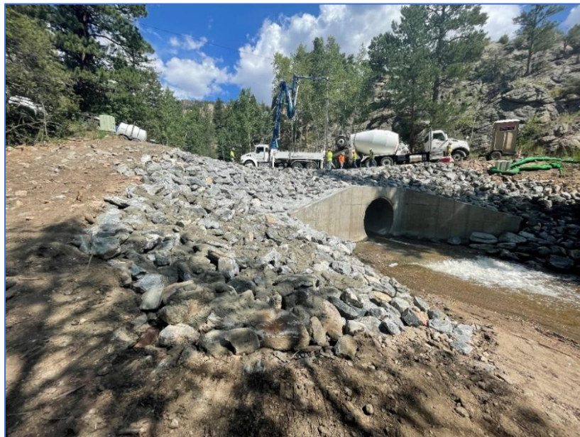
Photo 18: Upper Streamside Culvert – This photo shows the grouting operation for the overtopping protection
