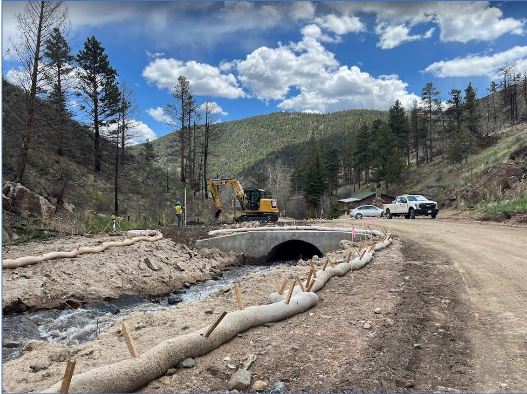
Photo 15: Post-Construction - Looking downstream at the culvert inlet and construction of a low-water crossing to help facilitate flows back into Sevenmile Creek past the downstream end of the structure (2023)
