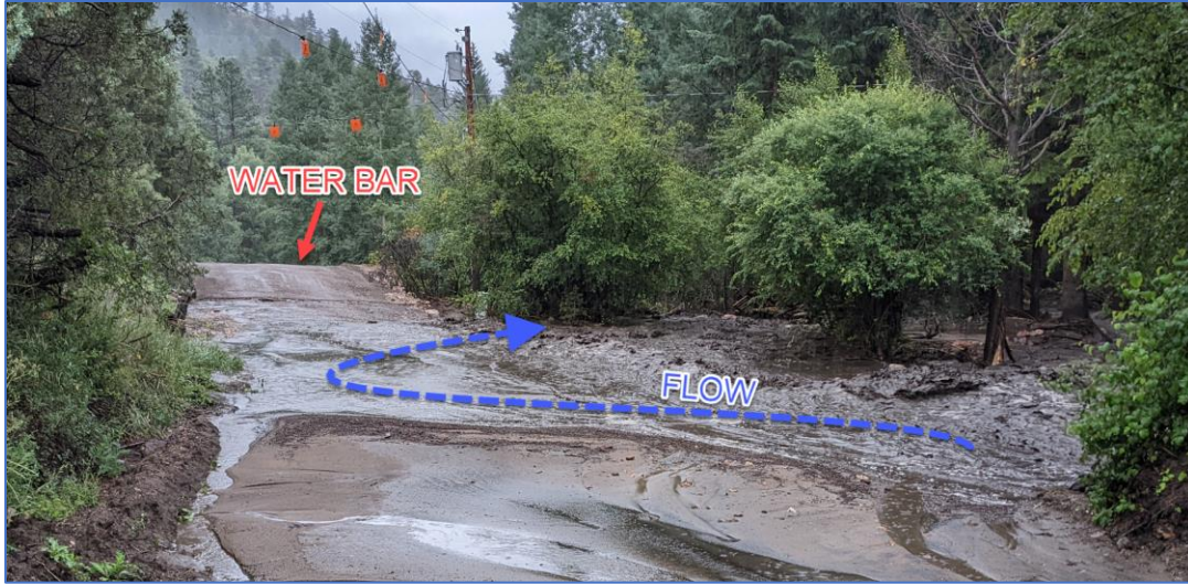
Photo 20: Effectiveness of Water Bar Demonstrated During High Flow Event
