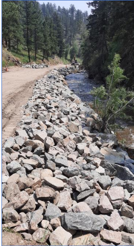
Photo 28: Typical Riprap Installation (Completed in August 2021)
