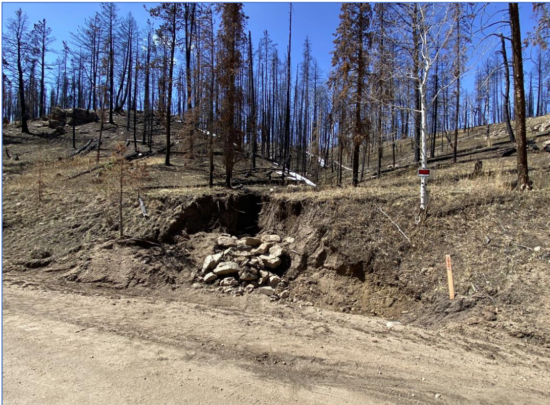
Photo 21: Pre-Construction – Example of roadway embankment erosion at 063E-0.26-44H (2022)
