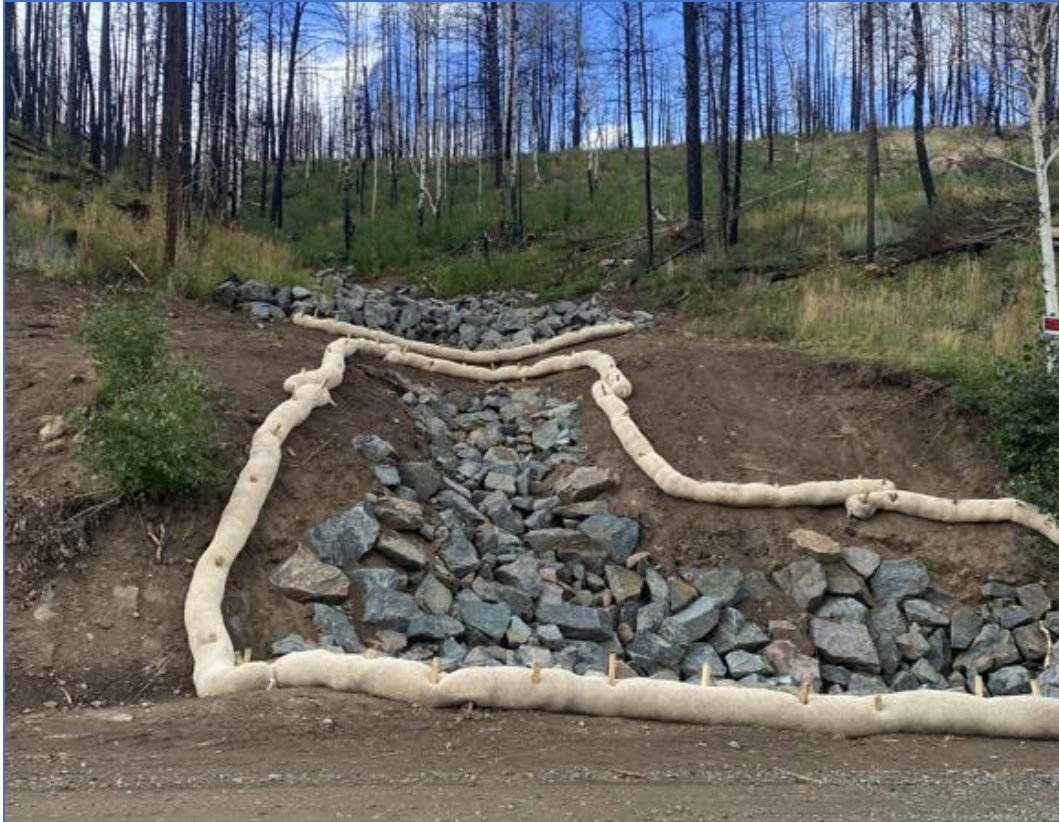
Photo 22: Post-Construction – Example of rock checks and rock chute at culvert inlet (2022)
