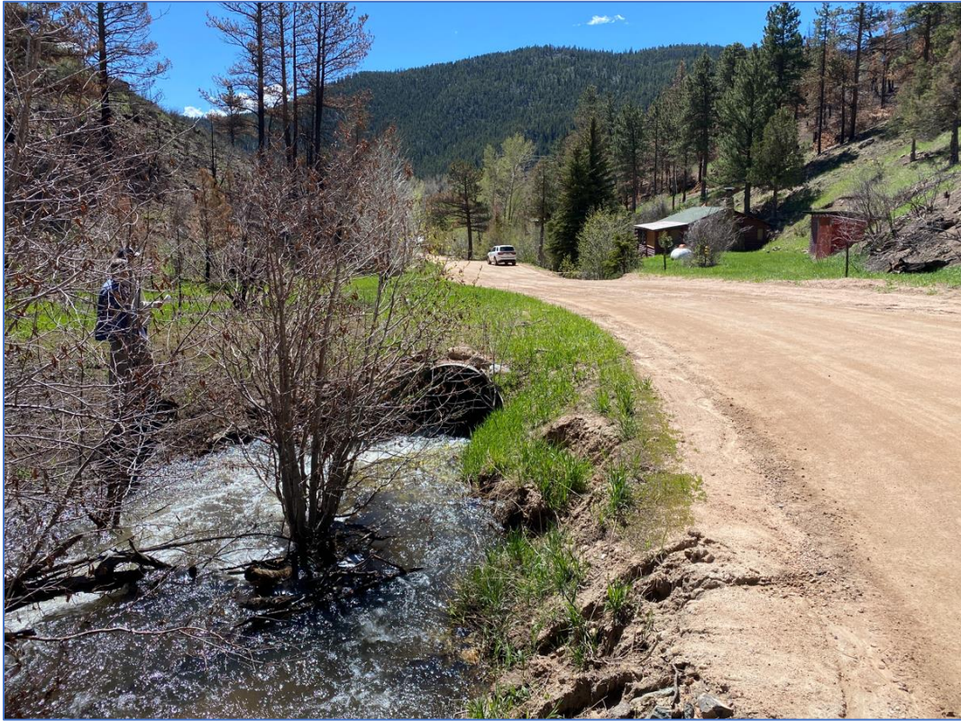
Photo 14: Pre-Construction - Looking South towards the line of cabins; the existing culvert had frequent overtopping events (2021)
