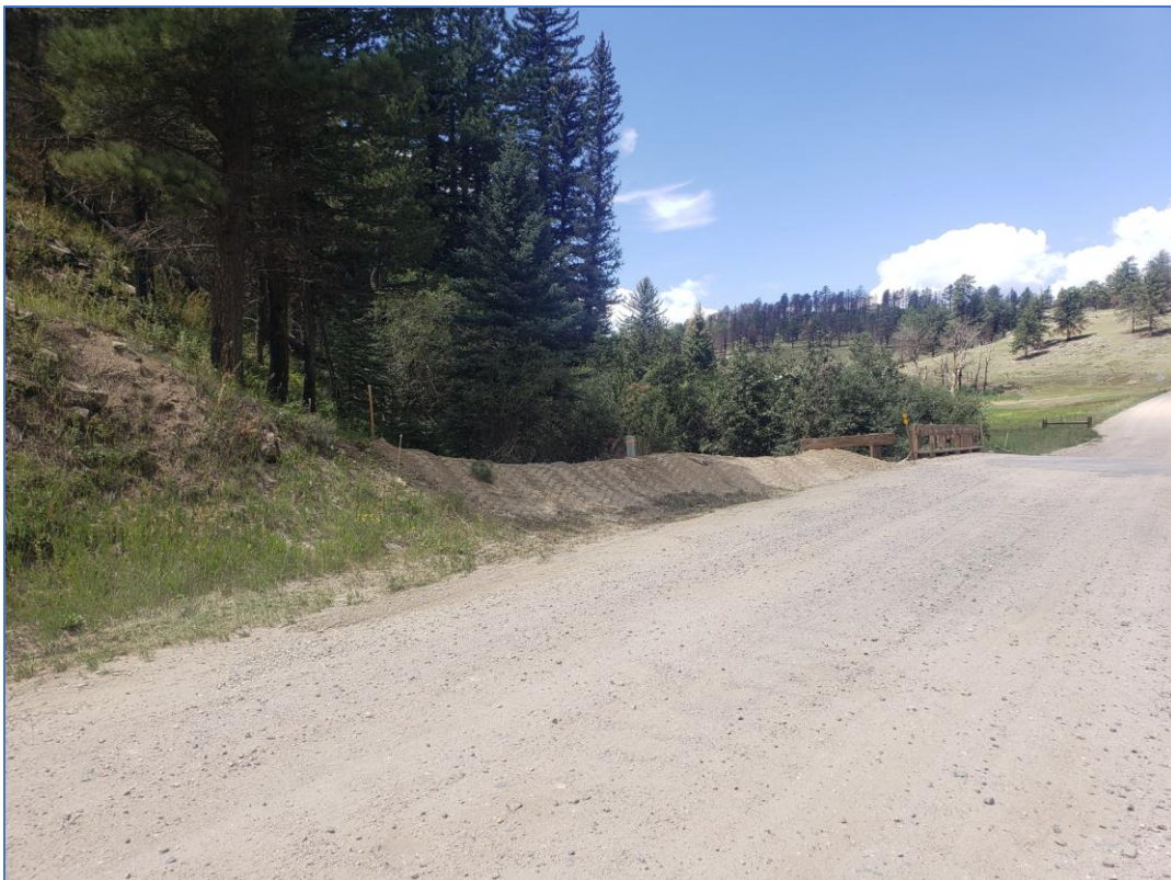
Photo 7: Post-Construction - Installation of the Earthen Berm (2022)
