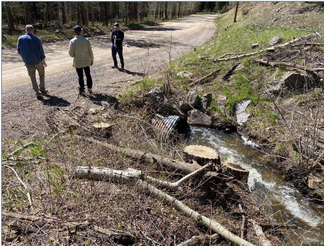
Photo 8: Pre-Construction - Undersized Culvert Inlet (2021)
