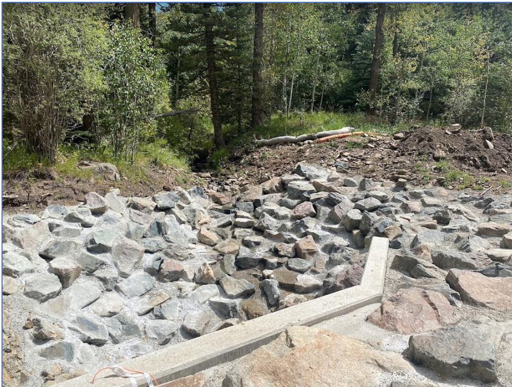
Photo 9: Unnamed Tributary looking Upstream at the grouted boulders (2022)
