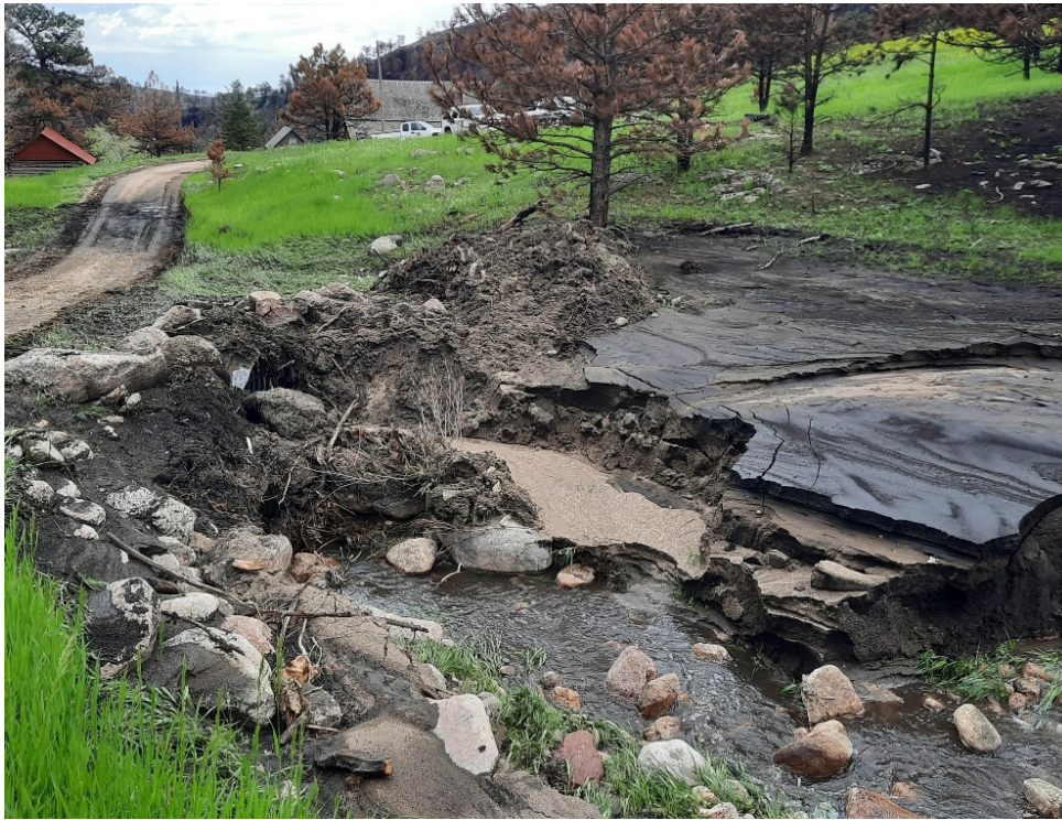
Figure 14. Clogged culvert and sediment deposition following May 30 rain event on Heil Valley Ranch.
