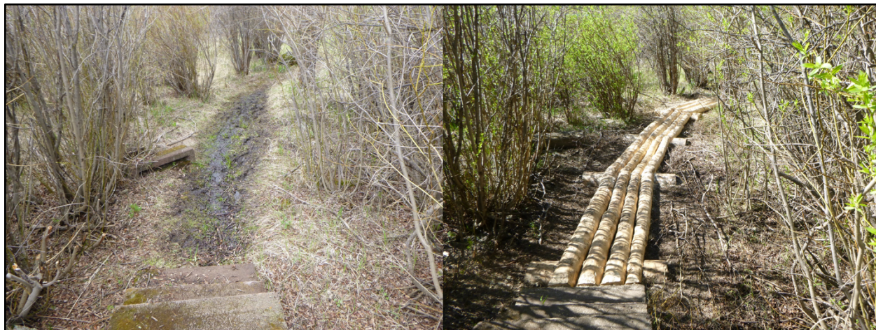
Figure 24. Before (left) and after (right) of puncheon constructed through wetland area.
