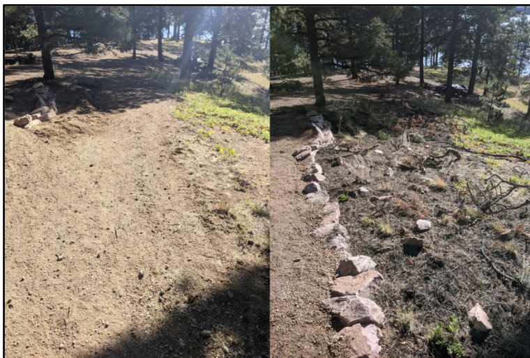
Figure 31. Before (left) and after (right) of barrier wall construction and restoration.
