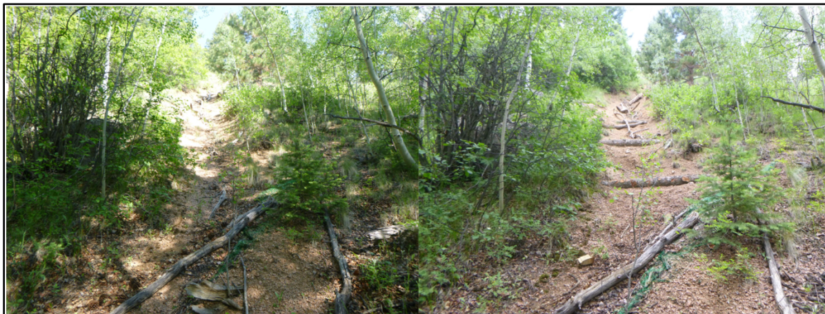
Figure 26. Before (left) and after (right) of check dam construction at Nichols Trail.
