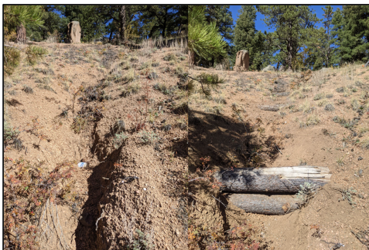
Figure 32. Before (left) and after (right) of check dam installation. An example of a 2-tiered check dam center right.
