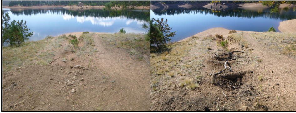
Figure 33. Before (left) and after (right) of check dam installation in a gully flowing towards the reservoir.
