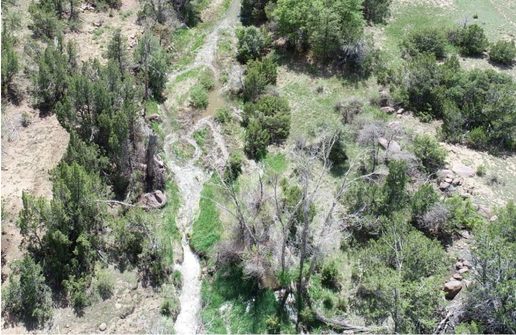
Figure E1: Aerial view of the reference reach looking upstream
