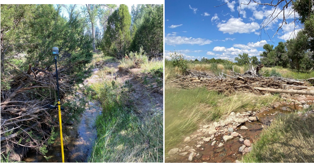
Figure D1: Site 1 location flood debris lines measure about 6' of water (left) and large debris jams piled up (right).
