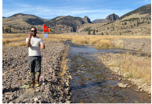
Looking upstream from Station 54+00. Upstream to be stabilized single-channel with 50ft flood-prone zone, while downstream will allow for braiding during high water events.
