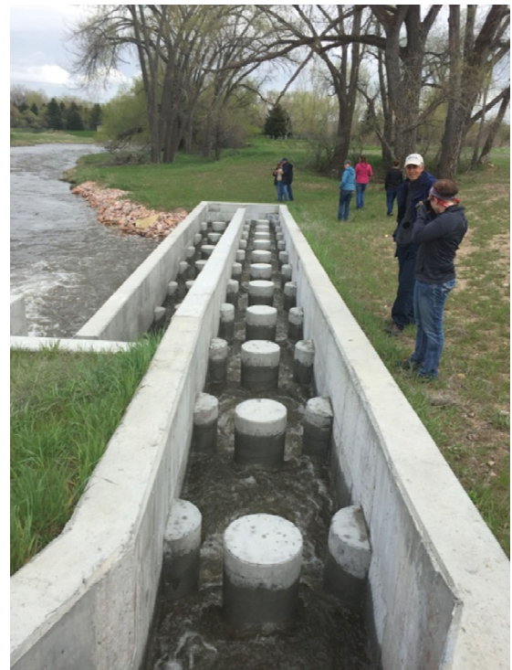
Figure 6 - Dual slot pile fishway designed for passing native fish species near Sheridan Wyoming.
