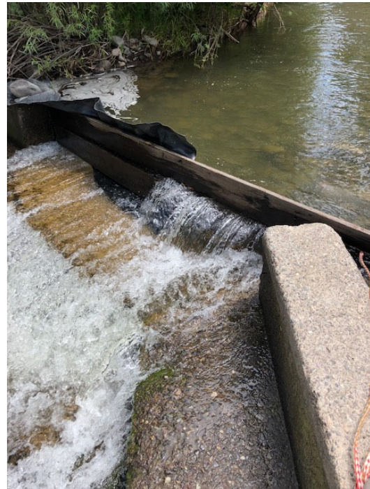
Figure 2 -Typical operation with check boards installed.
