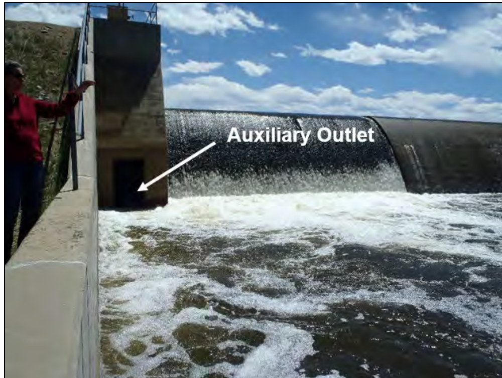
Figure 1-7. Auxiliary Outlet (Standing at the base of the dam looking southeast)
