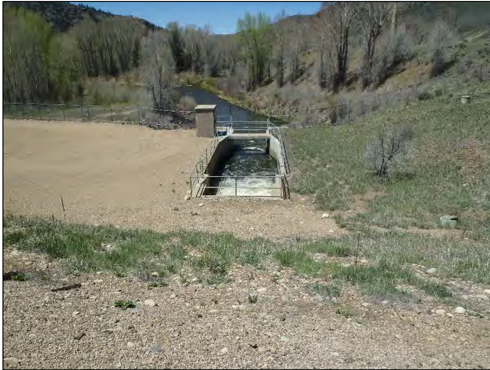
Figure 1-6. Low-Level Bypass Outlet (Standing on the dam embankment looking west/downstream)
