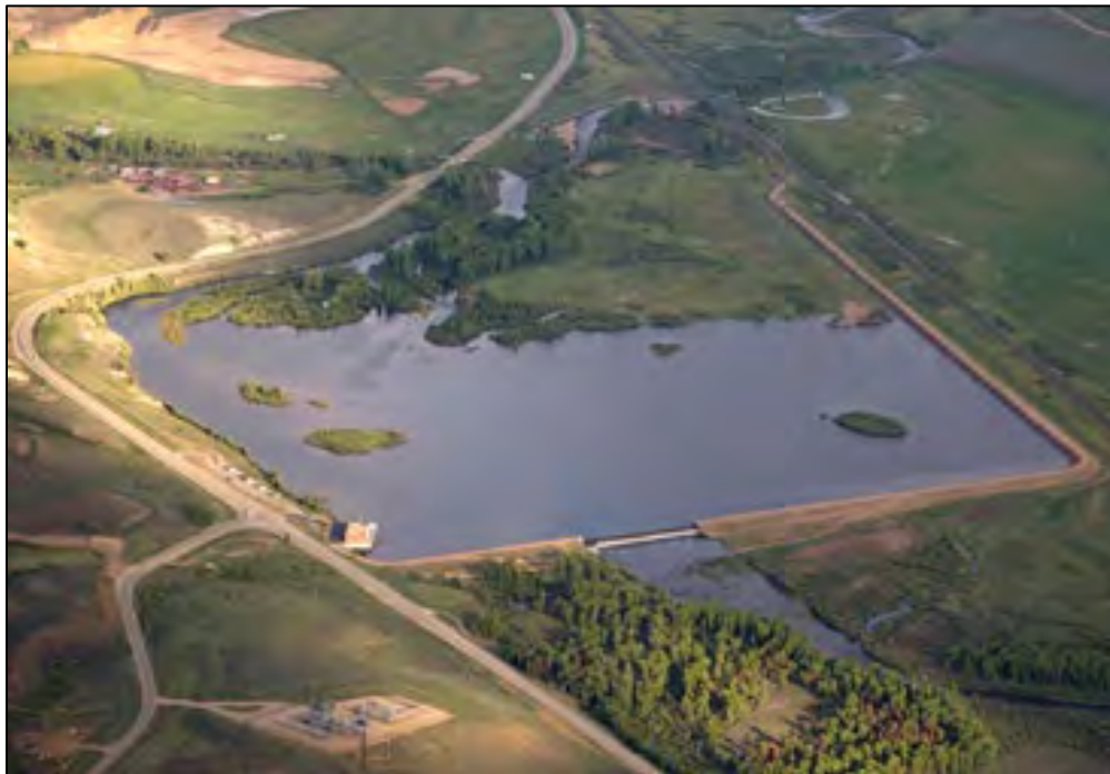
Figure 1-1. Reservoir (Aerial view of reservoir looking southeast)
