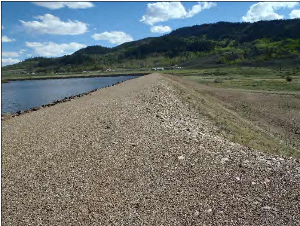
Figure 1-4. Downstream Dam Embankment (Standing on the western dam embankment leg looking south)
