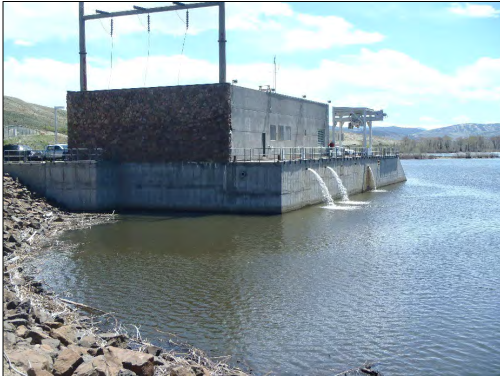
Figure 1-8. Pumping Plant (Standing on the dam embankment looking east)
