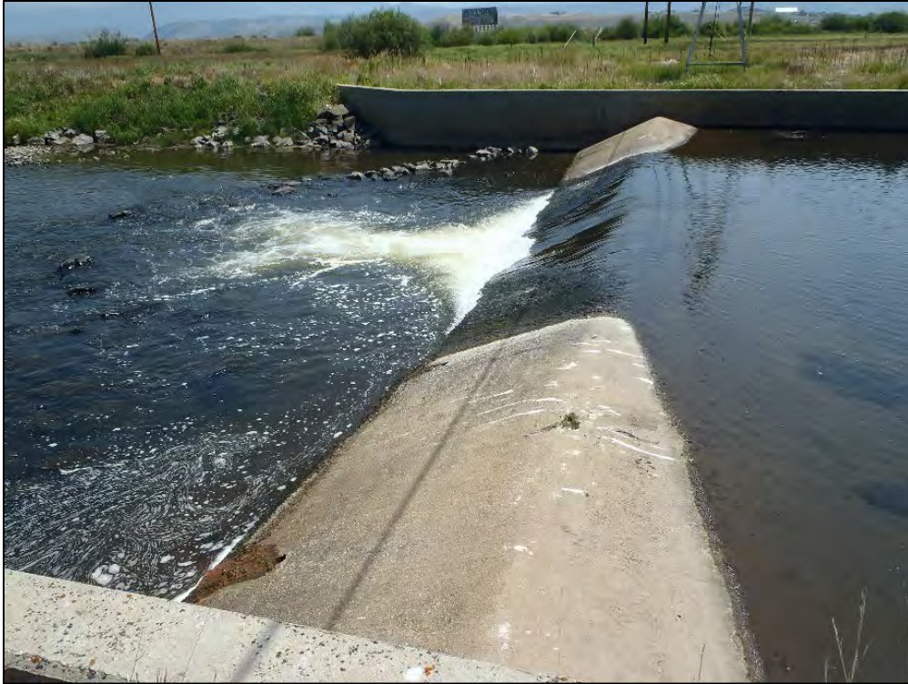
Figure 1-9. Fraser River Weir (Standing on the left wall looking east)
