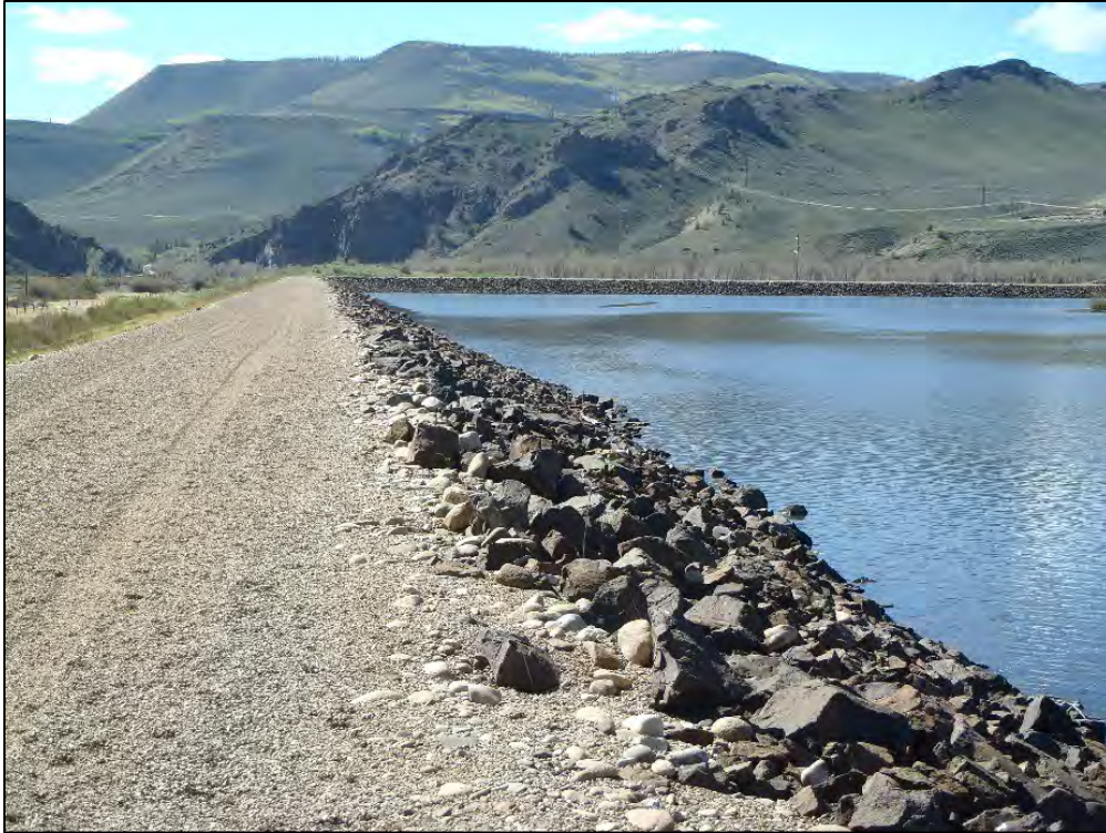
Figure 1-3. Upstream Dam Embankment (Standing on the southern dam embankment leg looking northwest)
