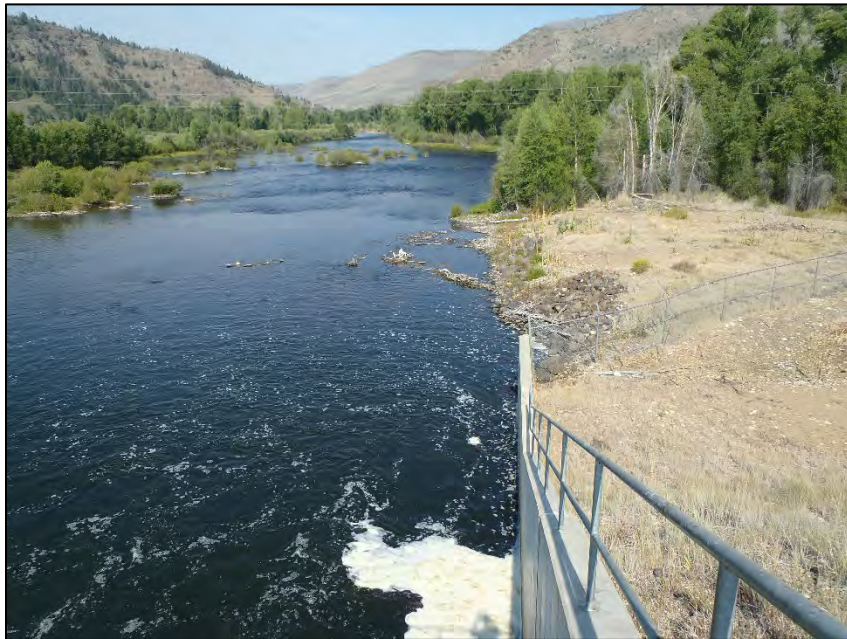
Figure 4-2. General View of Colorado River Riparian Corridor, Downstream of Windy Gap
