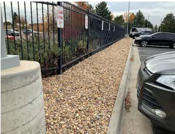
Nonfunctional Parking Irrigation Removed
