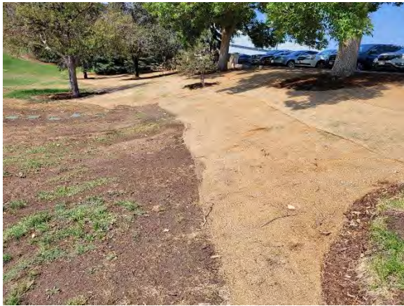
Admin. East Side slope areas blanketed for erosion
